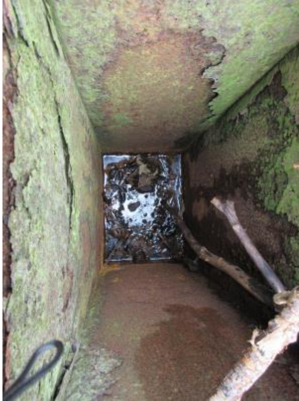
63. Vertical pit between buildings 37 and 38 where UST is suspected.
