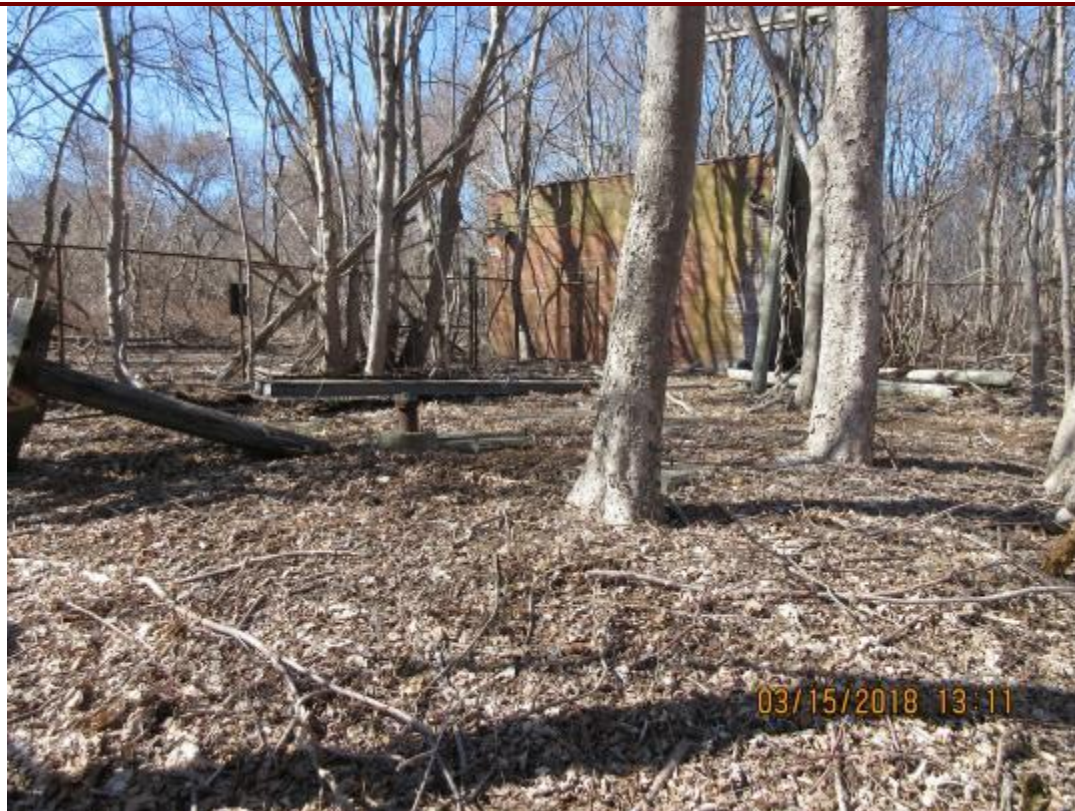
25. NED Site No. 13 Electric Substation/Transformer Pads.
