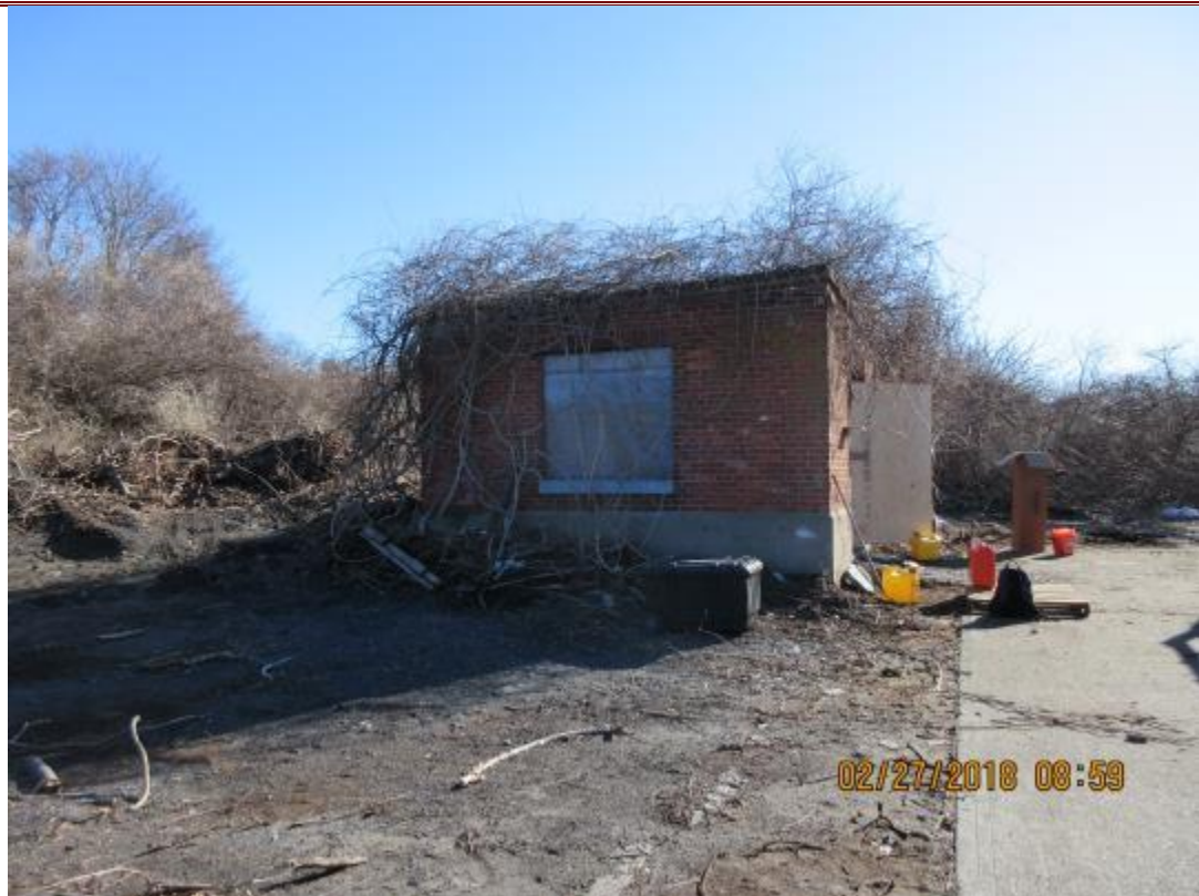
54. NED Site No. 33 Oil and Paint Storage Shed. Used a Credere basecamp during RI Field Activities.
