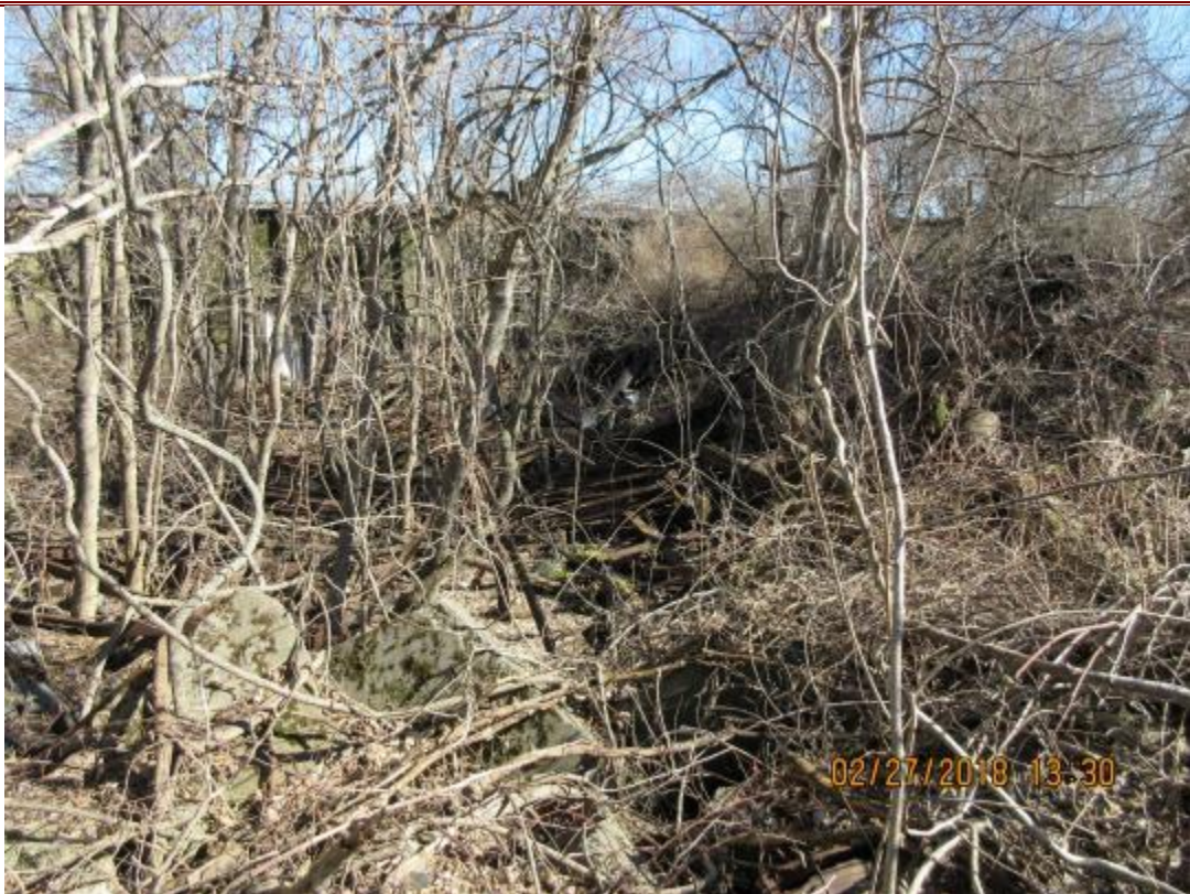
40. Bunkers from back side showing debris and vegetation inhibiting assessment.
