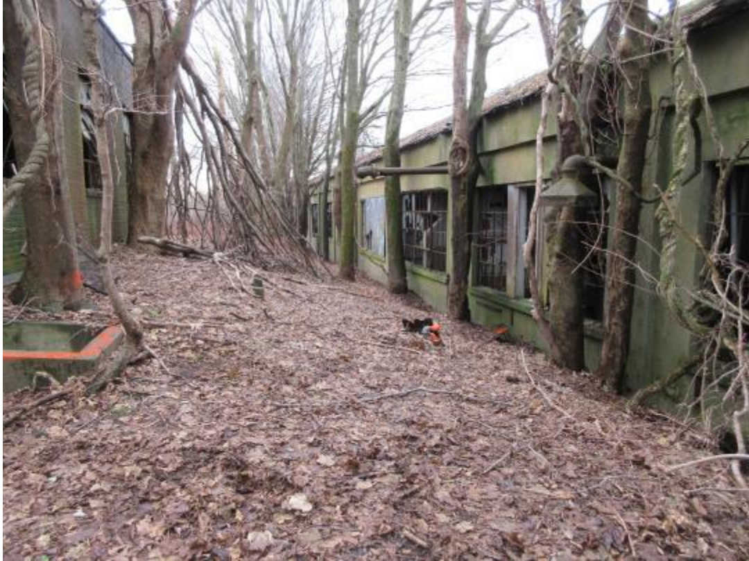
71. Area between Buildings 37 and 38 where vertical pipe chase suspected to be UST was observed.
