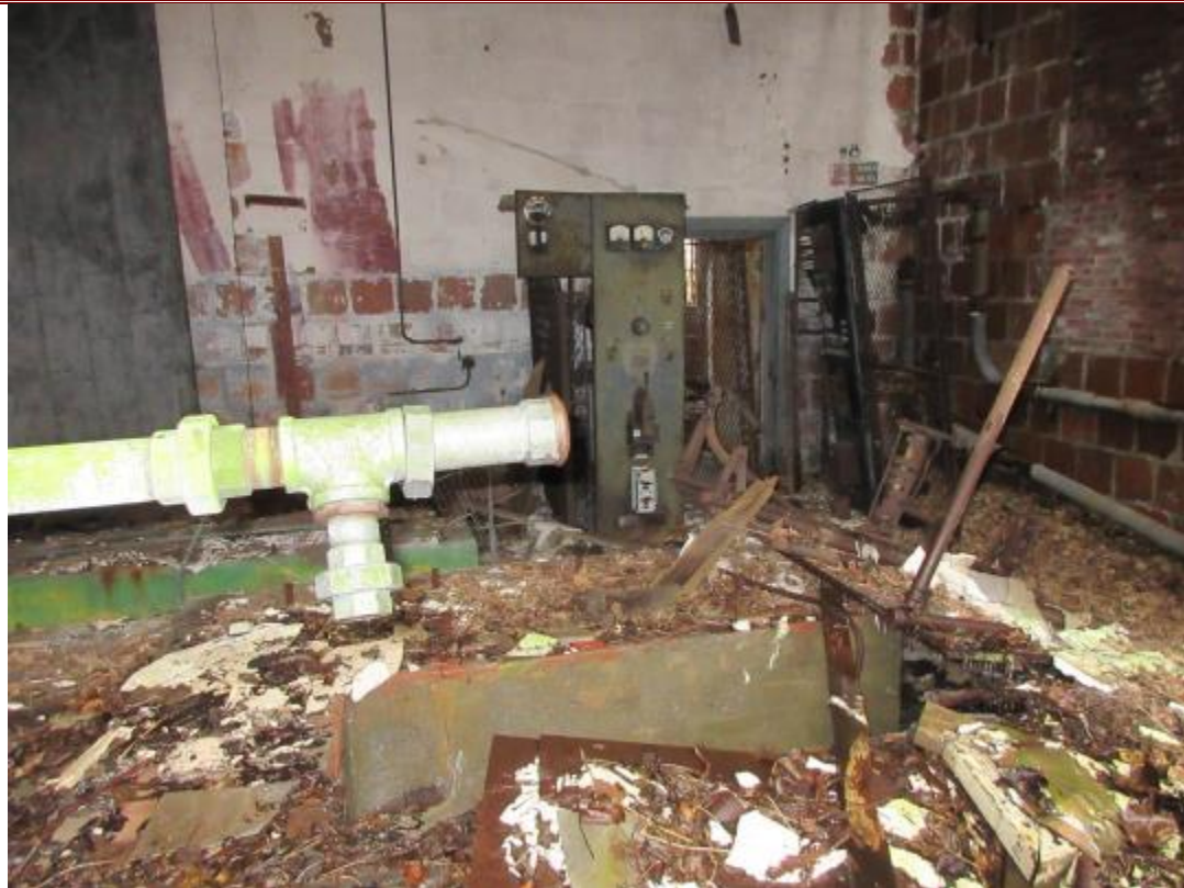
70. Interior of building Torpedo Storage building opposite wall of transformer house where electrical pen was observed.
