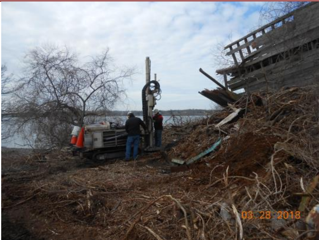
112. Geoprobe drilling at the Boiler House (NED Site 35).
