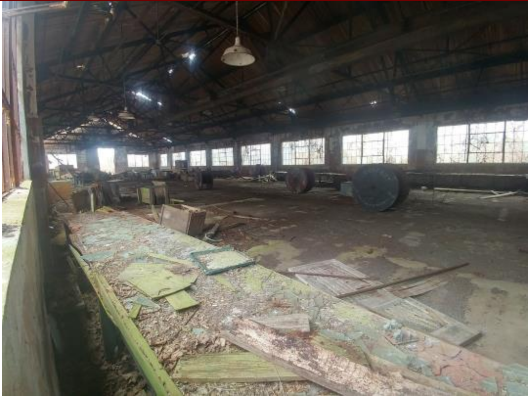
65. Interior of NED Site No. 38 Torpedo Storage building.
