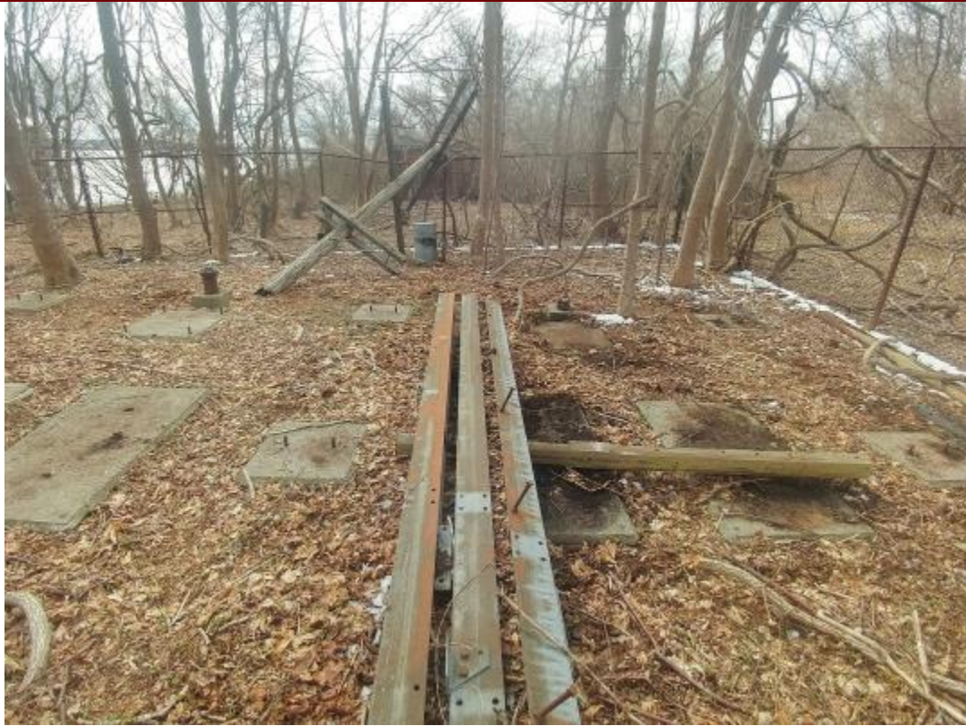
139. Concrete pad layout in NED Site 13 substation/transformer pen.
