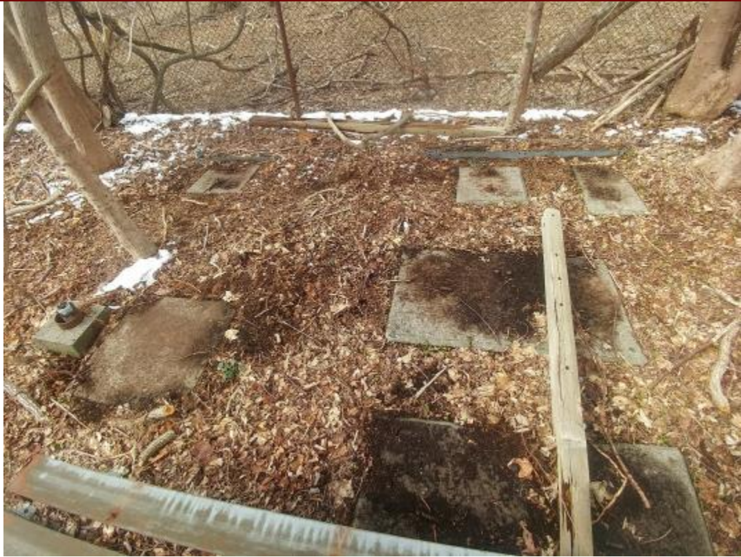
141. Concrete pad layout in NED Site 13 substation/transformer pen.
