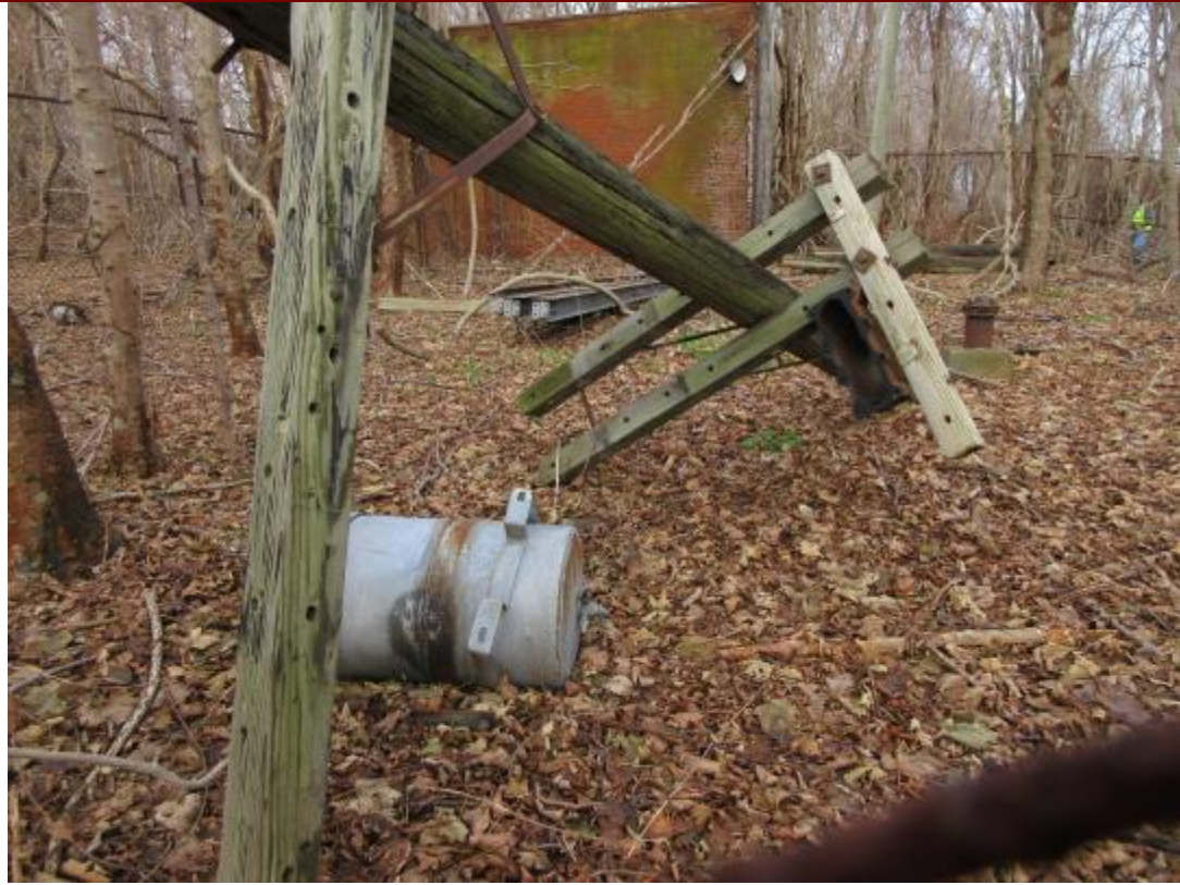
29. Pressure reservoir outside NED Site No. 13 in substation yard.
