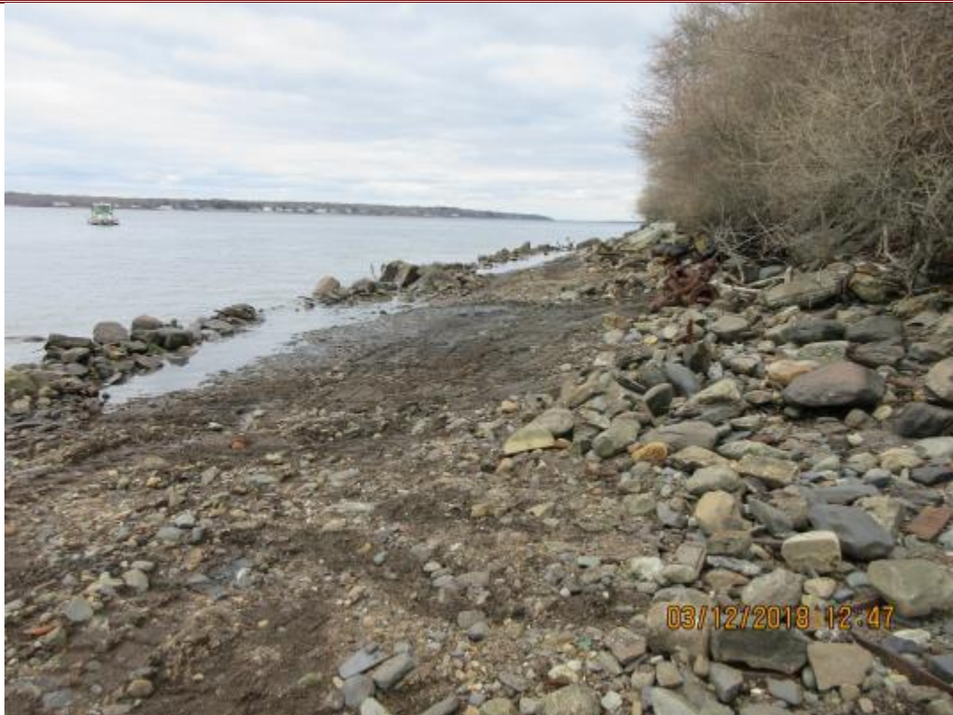
130. Restored beach after 10TP6, 10TP7 and 10TP8.
