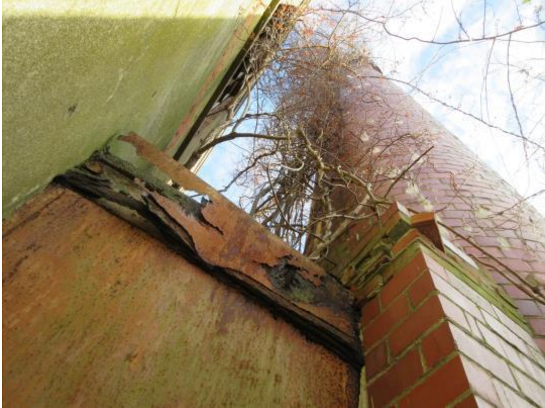
7. Stack on Incinerator (NED Site No. 8).
