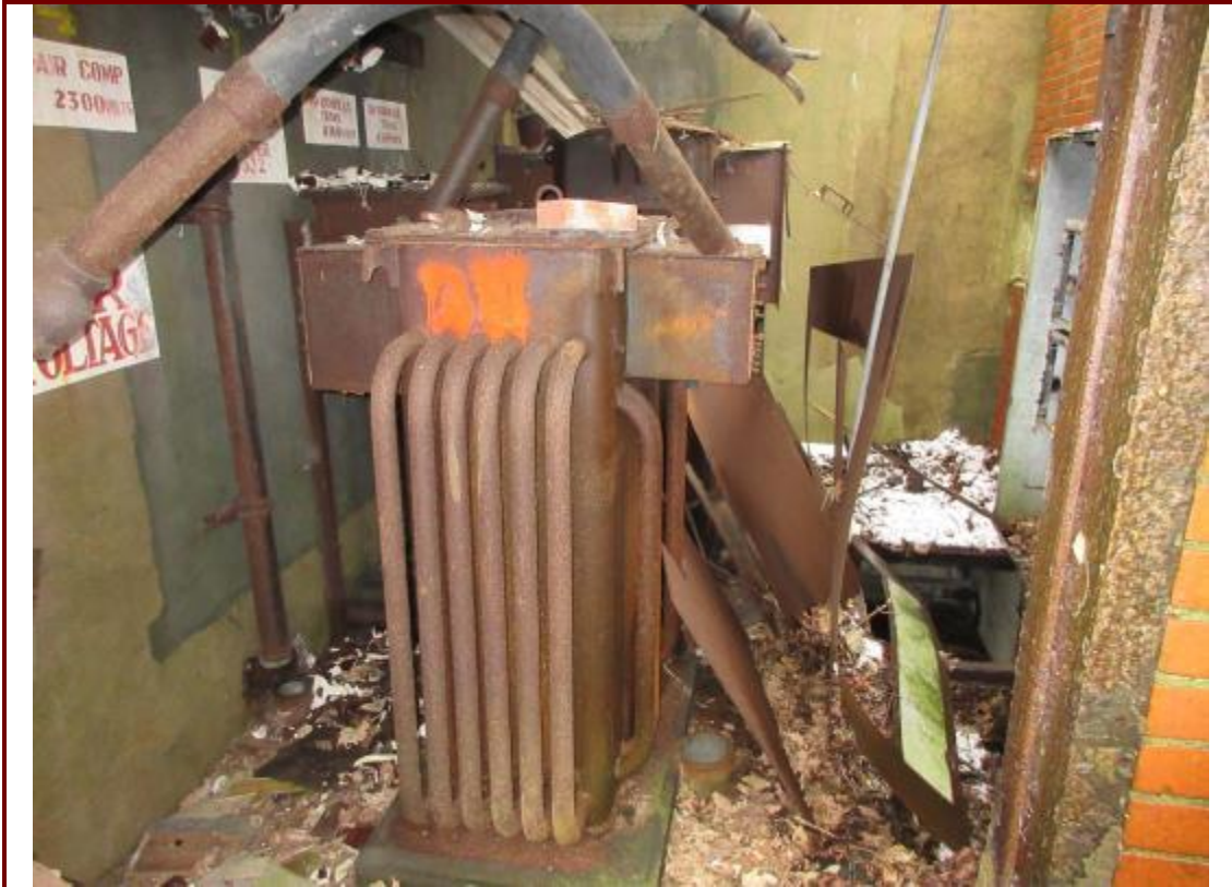
69. Interior of transformer house on north end of NED Site No. 38 Torpedo Storage building.
