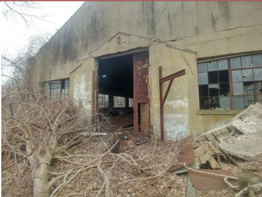
64. NED Site No. 38 Torpedo Storage building. Front southern bay door entrance.
