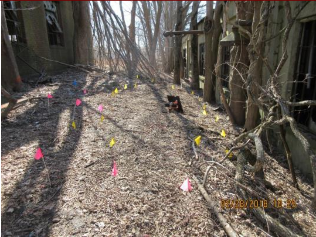
93. Outline of suspect UST between buildings 34 and 38.
