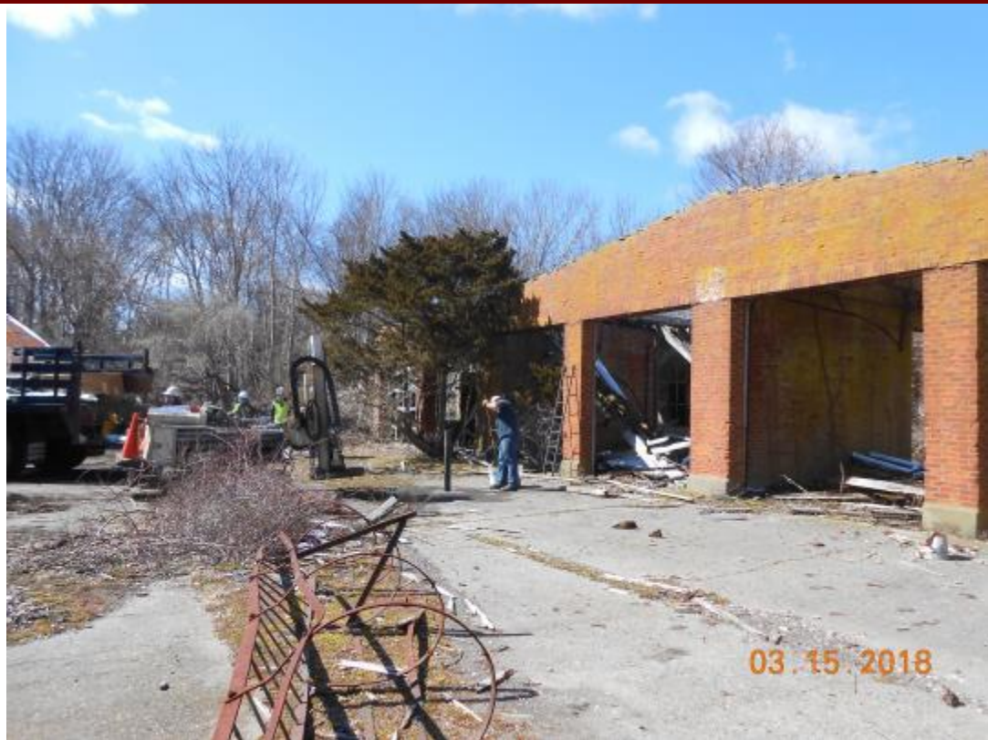
113. Installation of 12OBMW1 by the Fire Station (NED Site 12).
