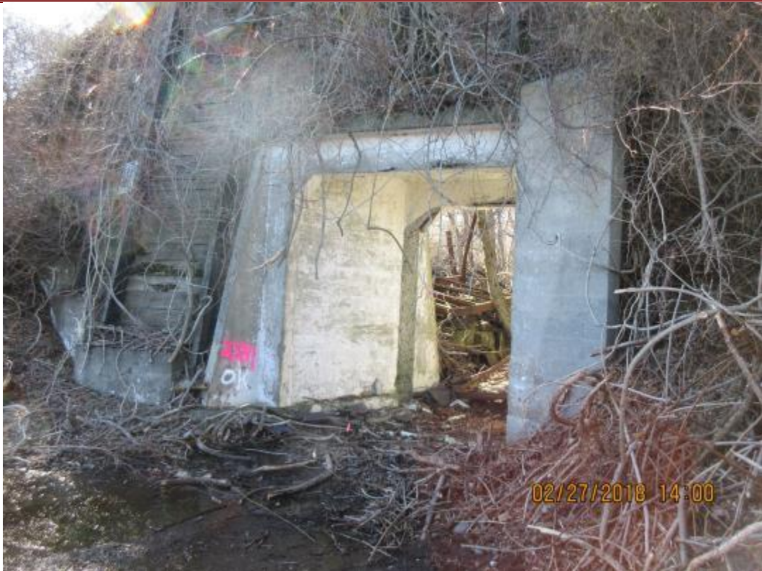
38. Typical bunker entrance condition.
