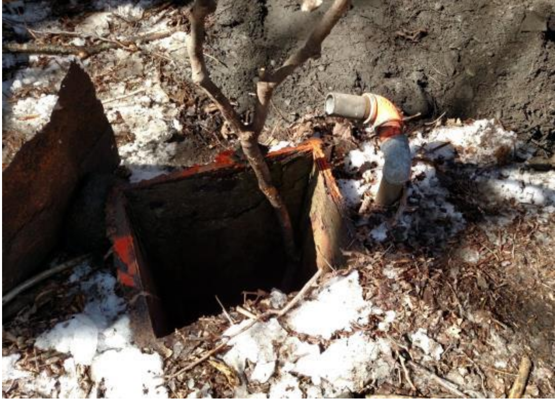
95. Vertical pipe chase to suspect UST between buildings 34 and 38.
