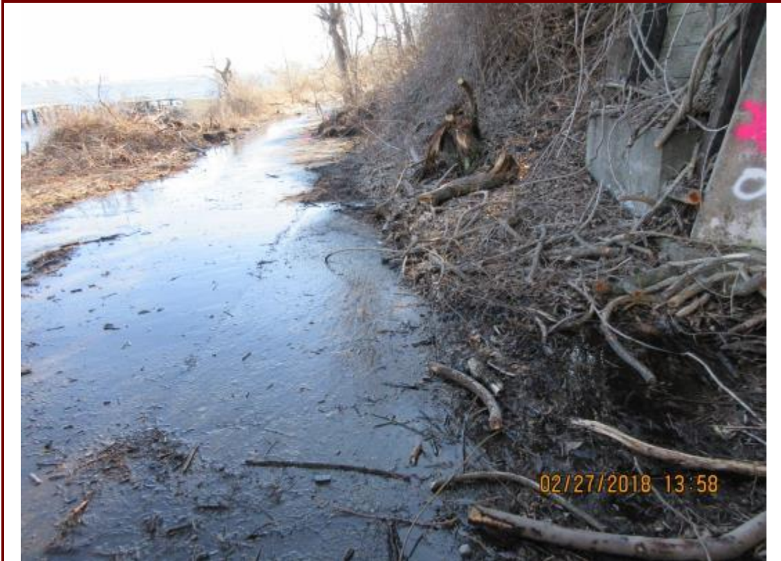
43. Apparent surface water drained observed on multiple occasions from Bunker #11.
