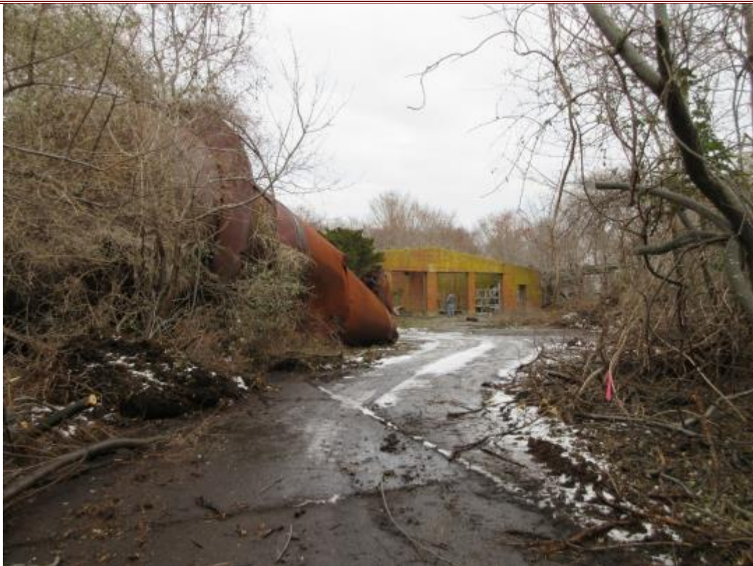
84. Typical concrete road in vicinity of fire station.
