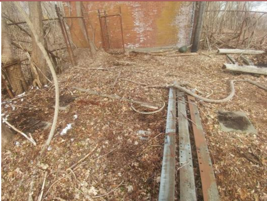
140. Concrete pad layout in NED Site 13 substation/transformer pen.
