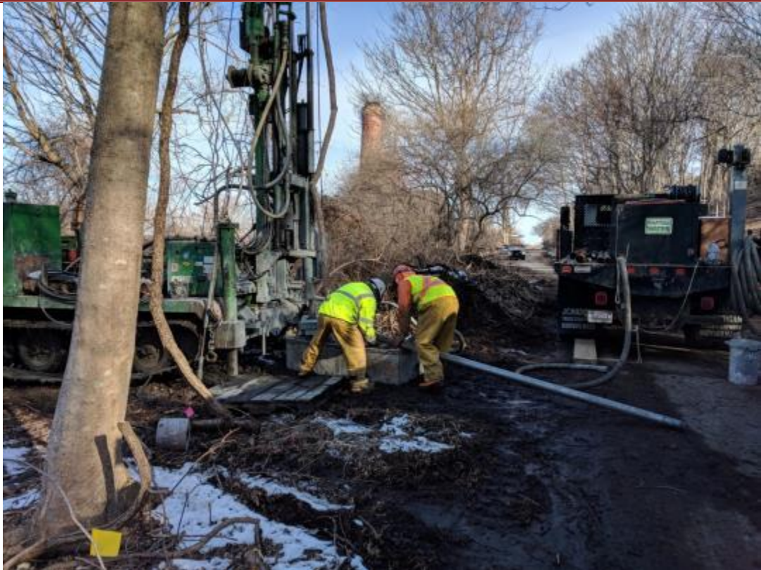
98. Conducting bedrock drilling at BRMW-3.
