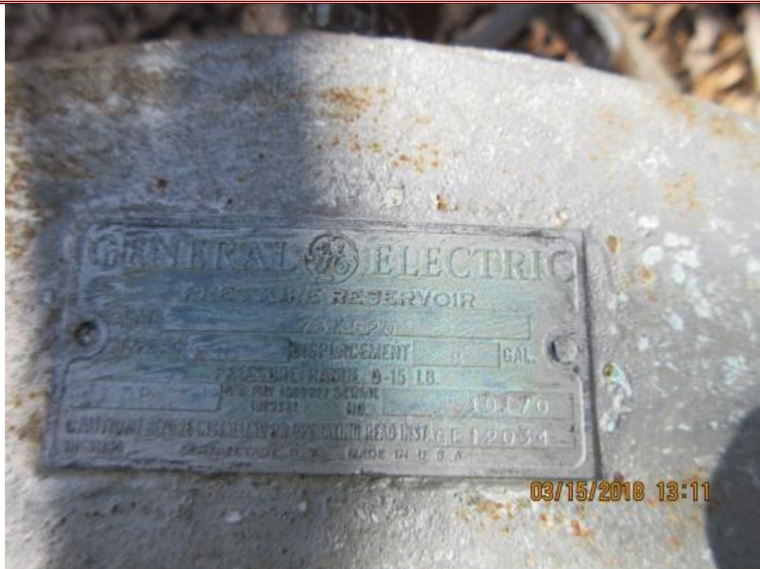
30. NED Site No. 13, pressure reservoir label.
