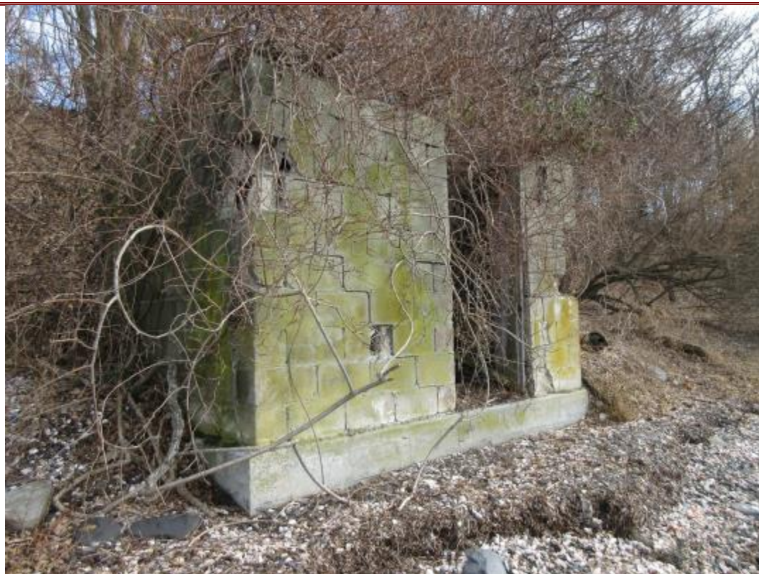
2. NED Site 4 Pump House on beach on western side of island.
