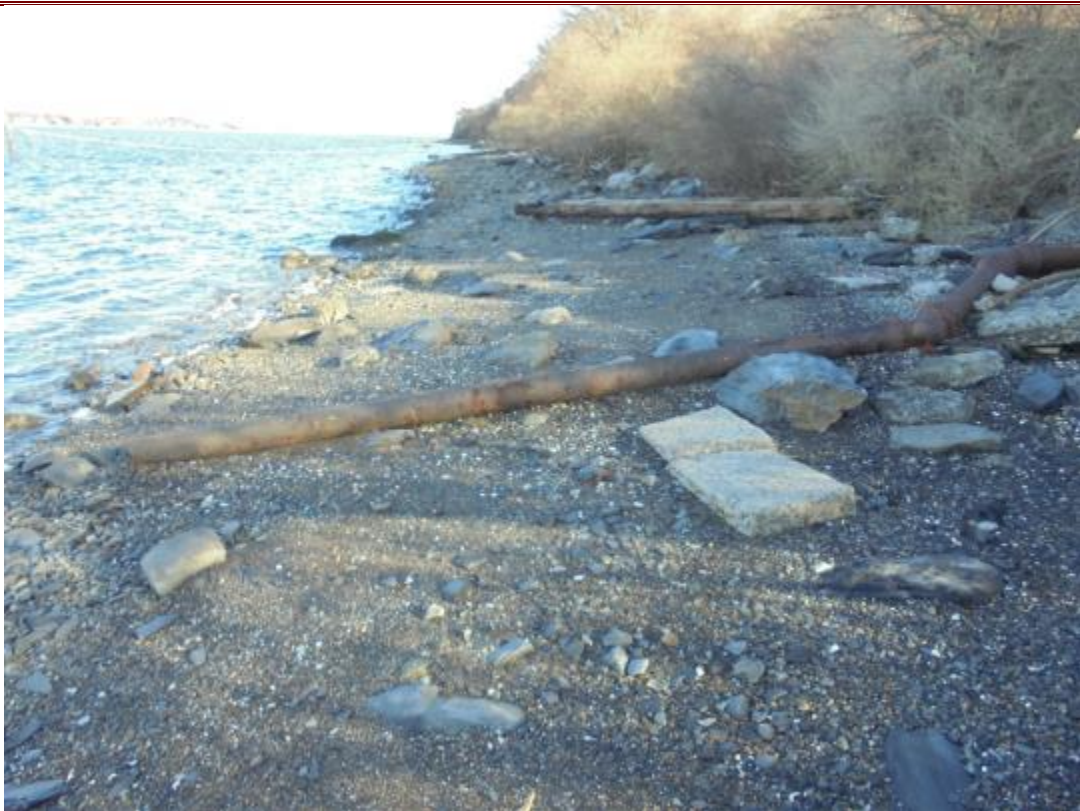
88. Pipe crossing west beach limiting travel of equipment down the beach at low tide.
