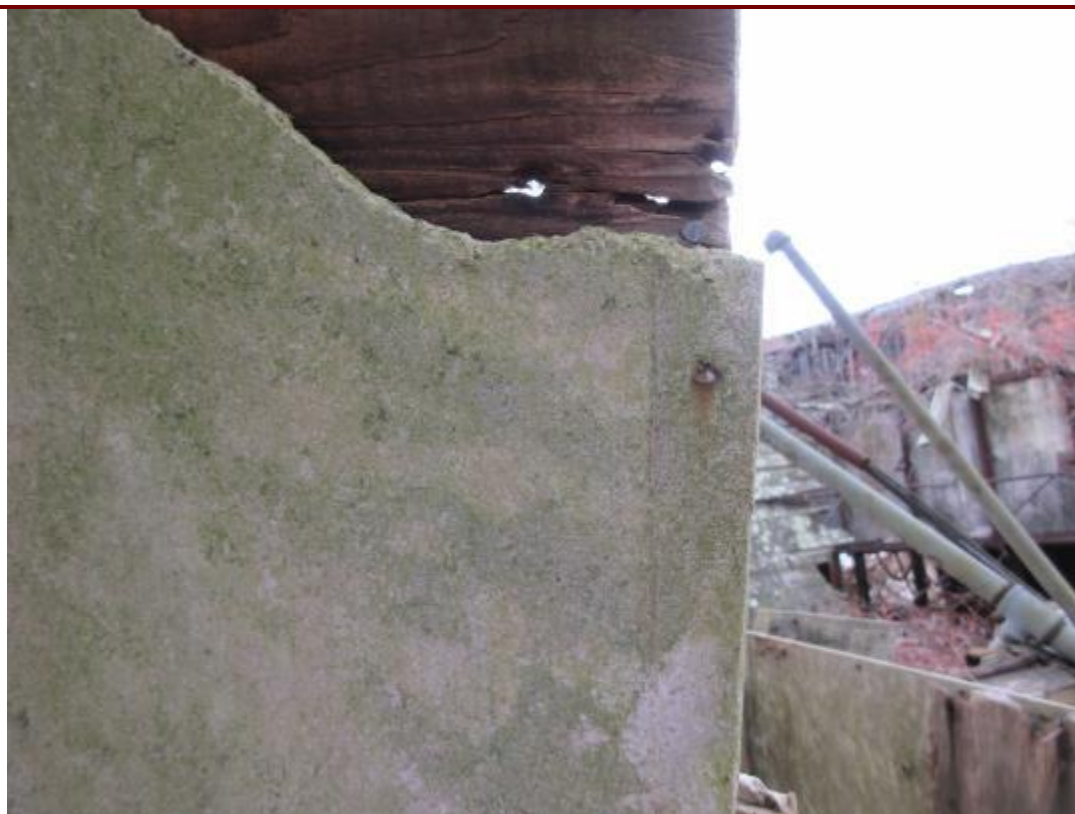
59. Transite paneling on most of collapsed boiler house (NED Site No. 35).
