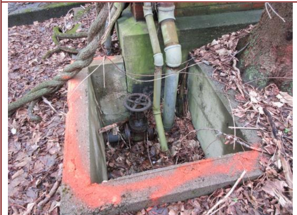
62. Valve outside NED Site 37 Misc. Storage Building.
