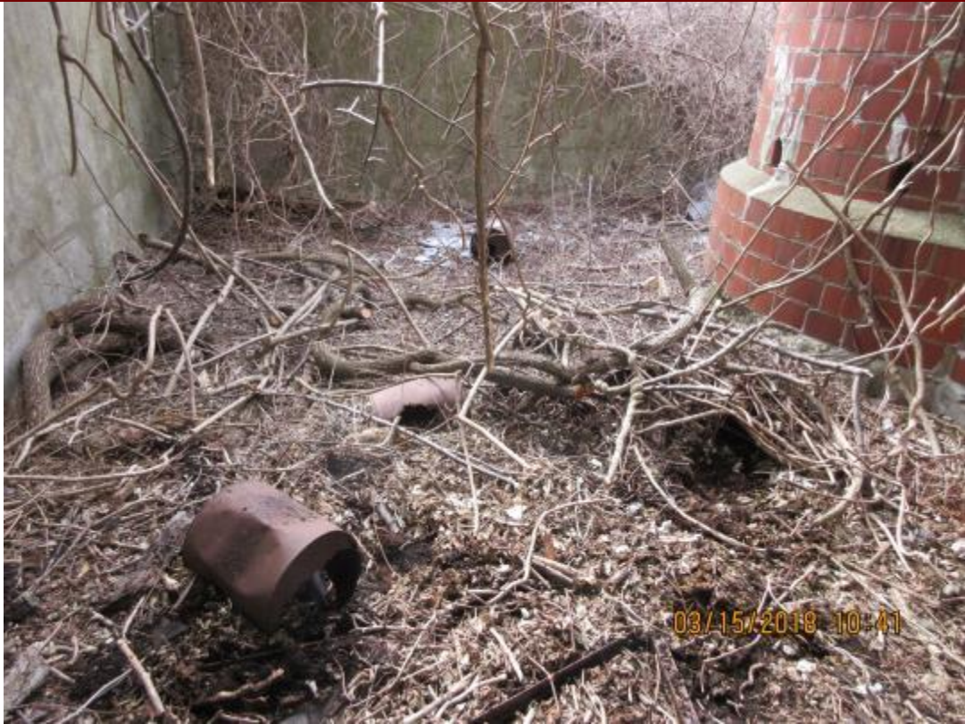
11. Containers at base of Incinerator stack (NED Site No. 8). Location of 08SS-1.
