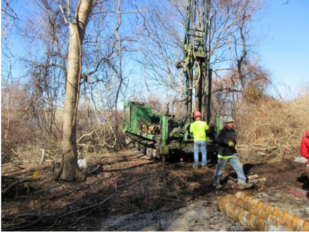
97. Conducting bedrock drilling at BRMW-1.
