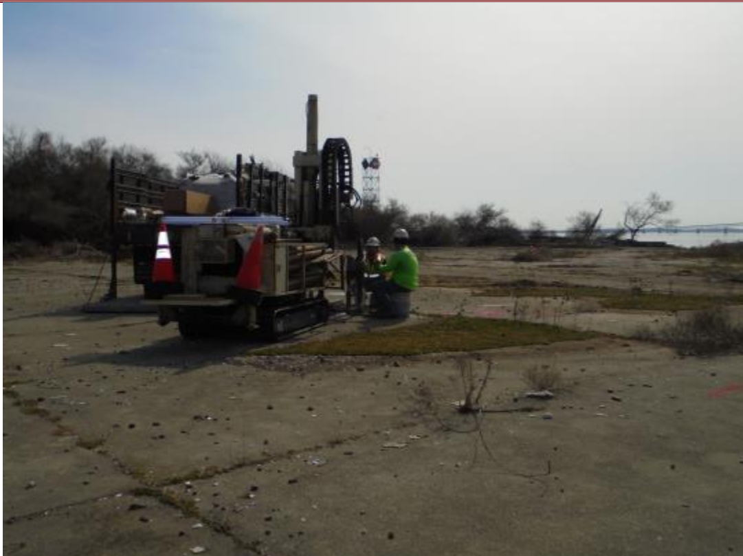
104. Concrete coring on the aviation pad.
