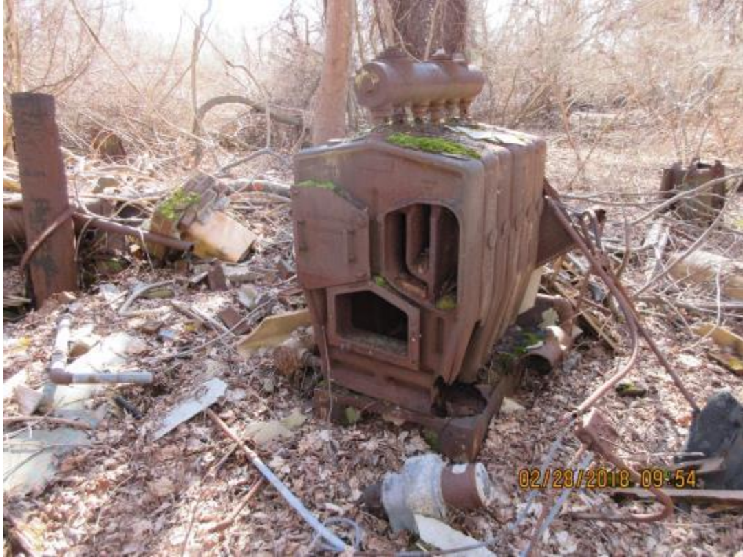
77. NED Site No. 49 Water Tower Pump House, boiler.
