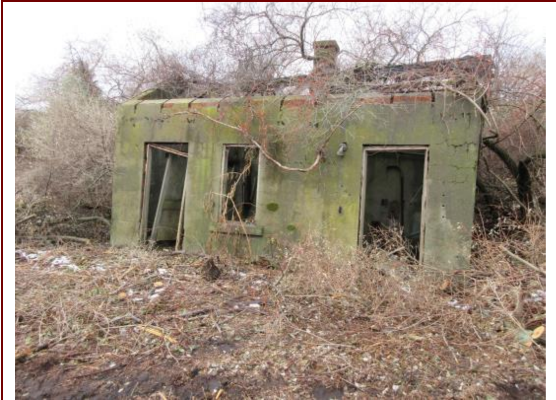
45. NED Site No. 24 Cable Terminal Building.
