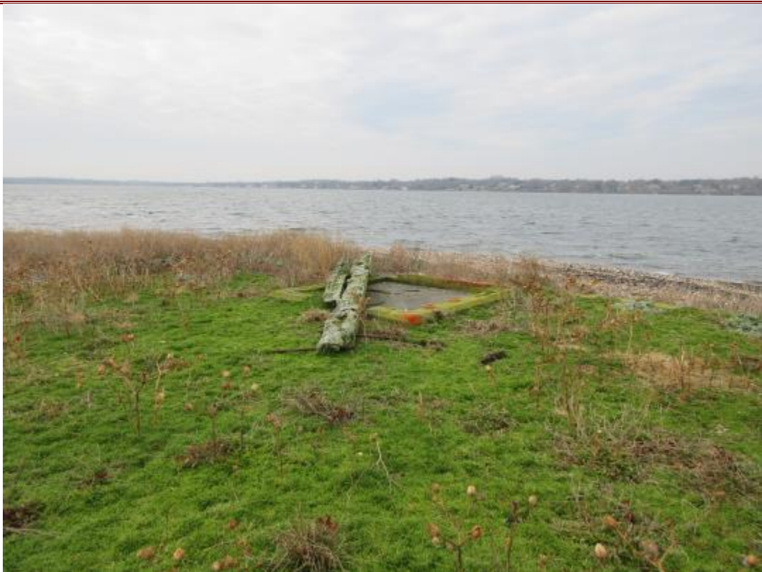
52. NED Site No. 30 Pyrotechnic Storage foundation on southeast corner of aviation pad.
