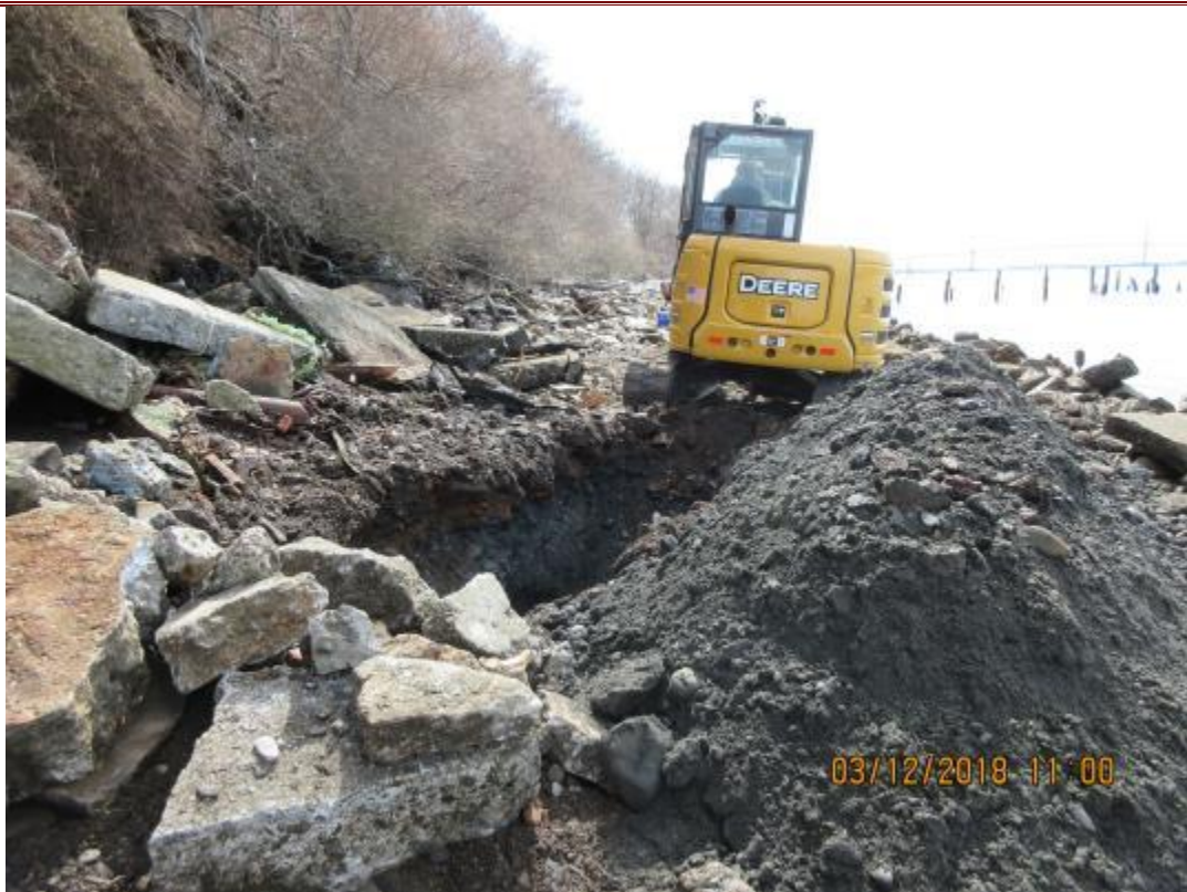
126. Location of 10TP7 facing south.
