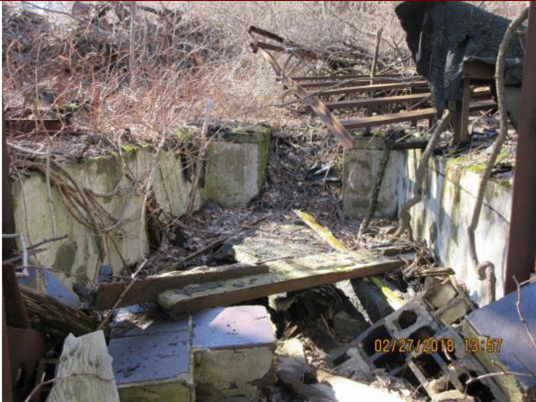
39. Typical bunker interior condition.
