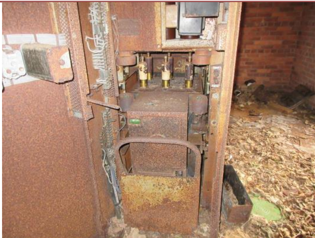
26. Transformers inside NED Site No. 13 building.
