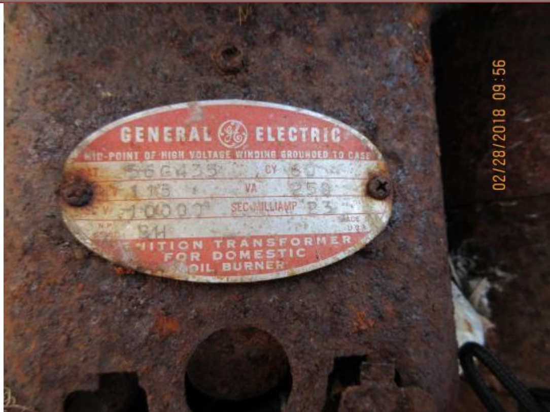
80. NED Site No. 49 Water Tower Pump House, transformer label.
