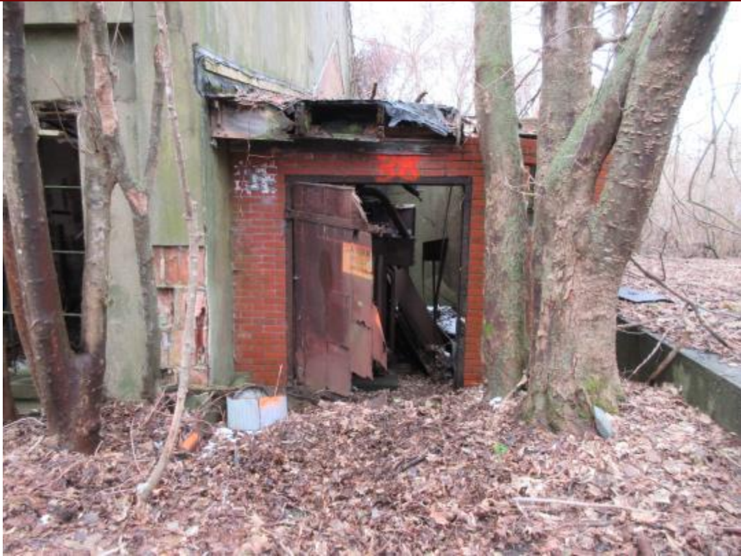
67. Transformer house on north end of NED Site No. 38 Torpedo Storage building.
