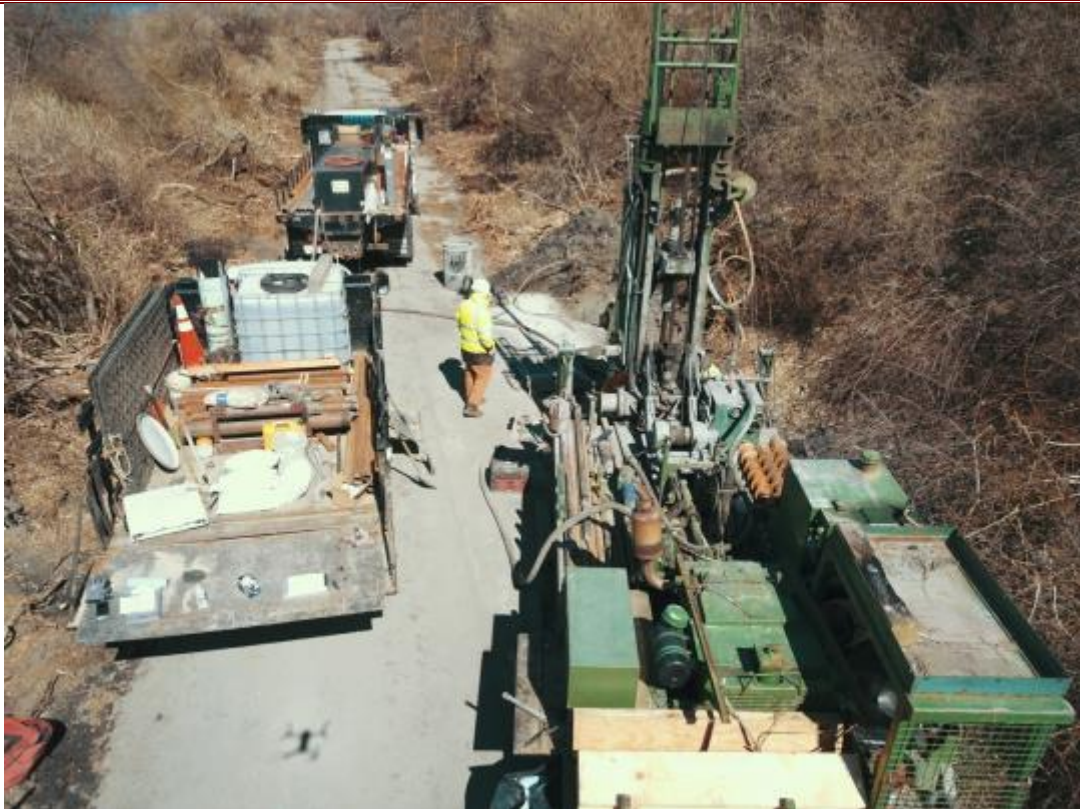
102. BRMW-5 during drilling activities.
