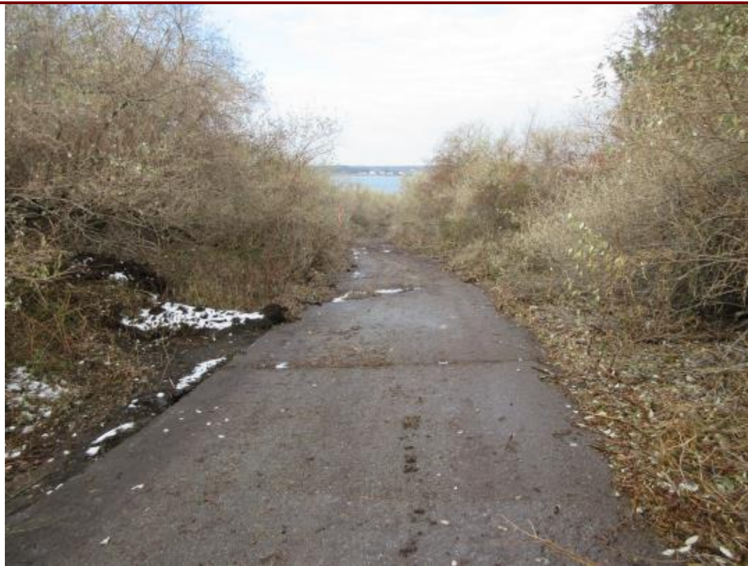
1. NED Site 1 Coal Storage North off end of road and on left of photo.
