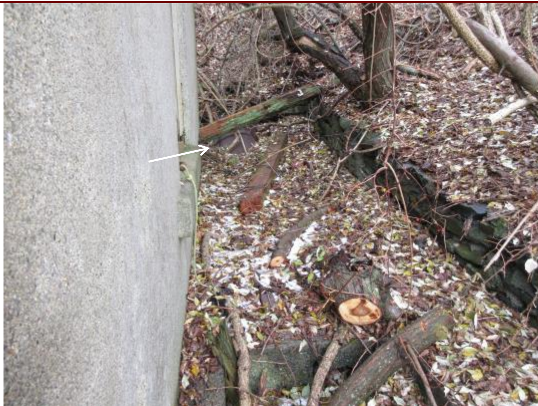
47. Buried drum by northwest corner of Cable Terminal Building (NED Site No. 24).
