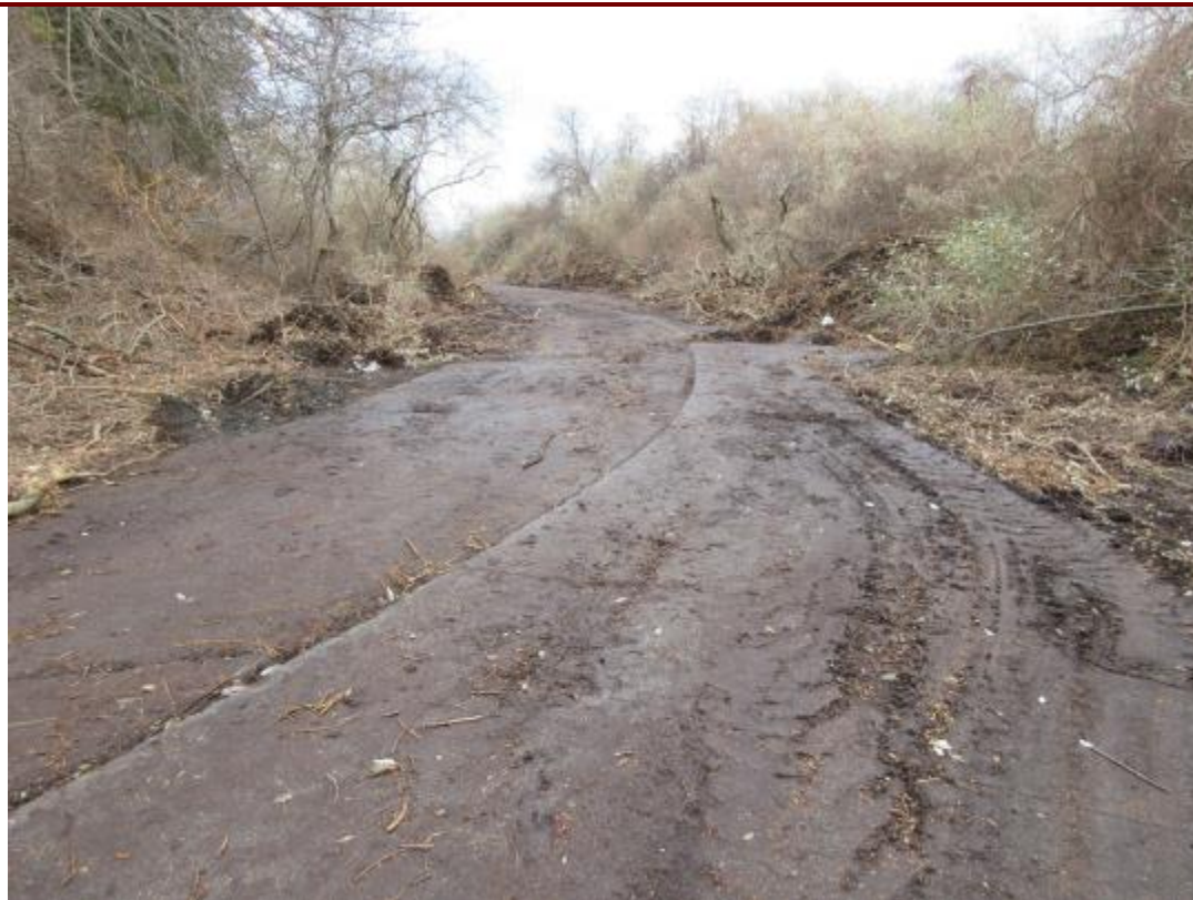
81. Typical concrete roads used for access throughout the island.
