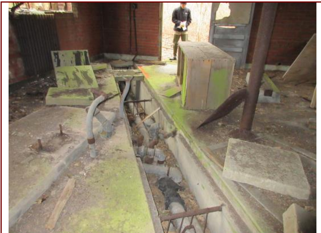
61. Pipe chase inside NED Site 37 Misc. Storage Building.
