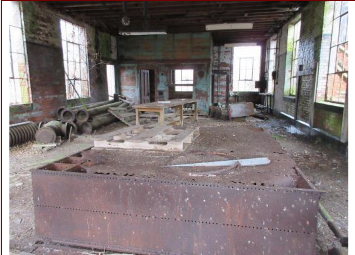
23. NED Site No. 12 Maintenance Shop/Garage/Fire Station, inside garage or maintenance bay.
