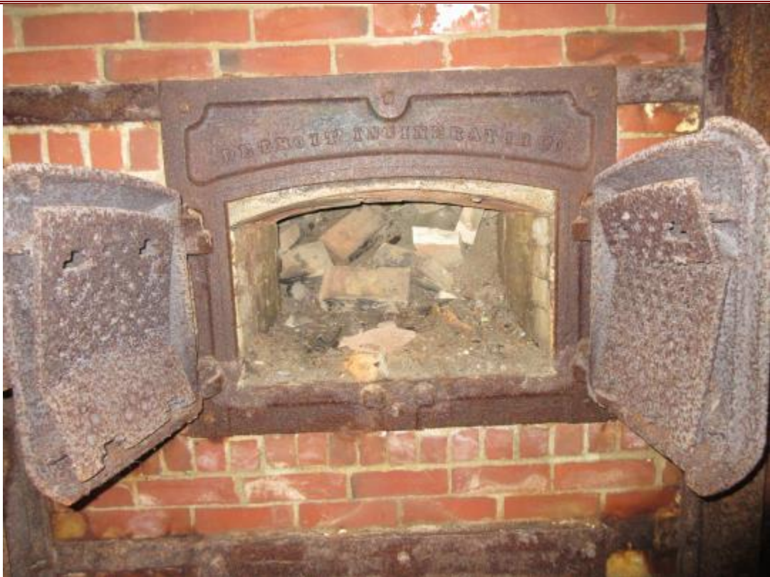
6. Fire boxes on bottom floor of Incinerator (NED Site No. 8).
