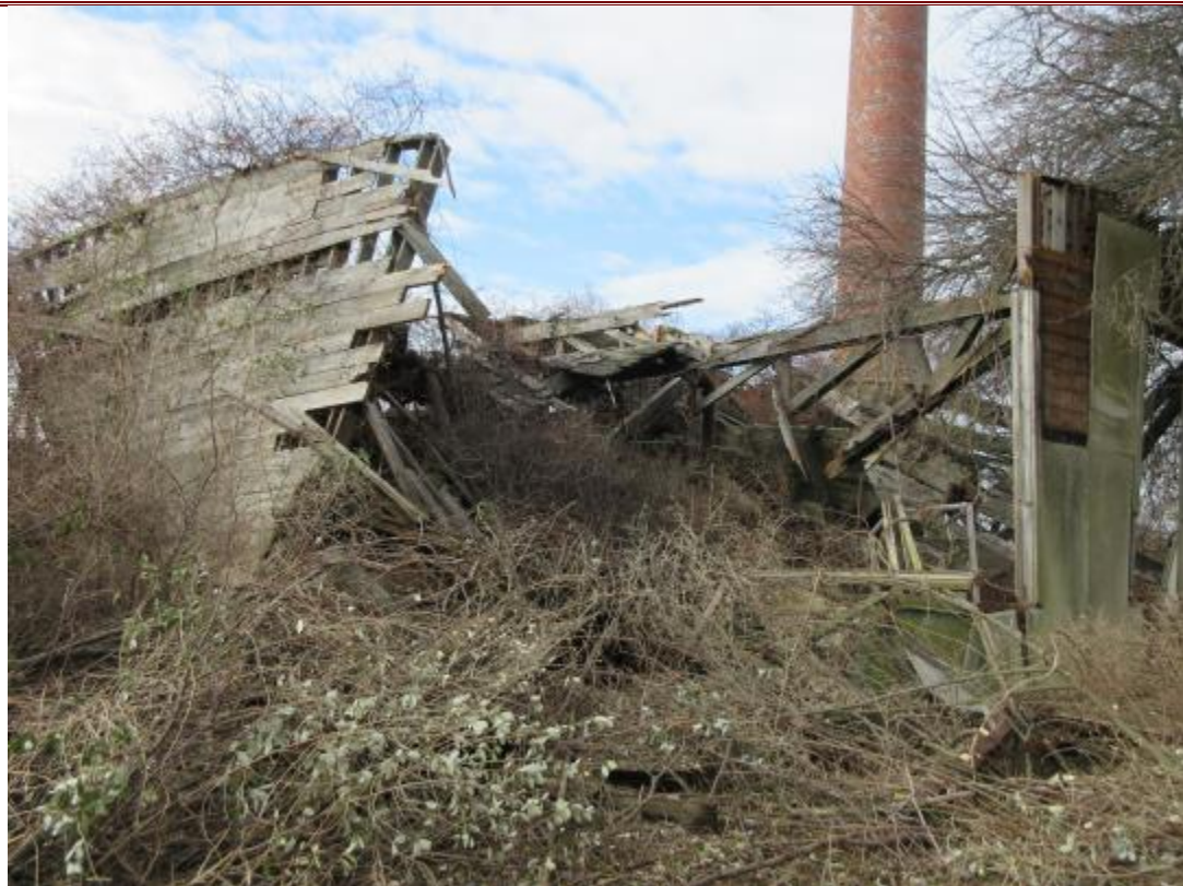
56. NED Site No. 35 Boiler House.
