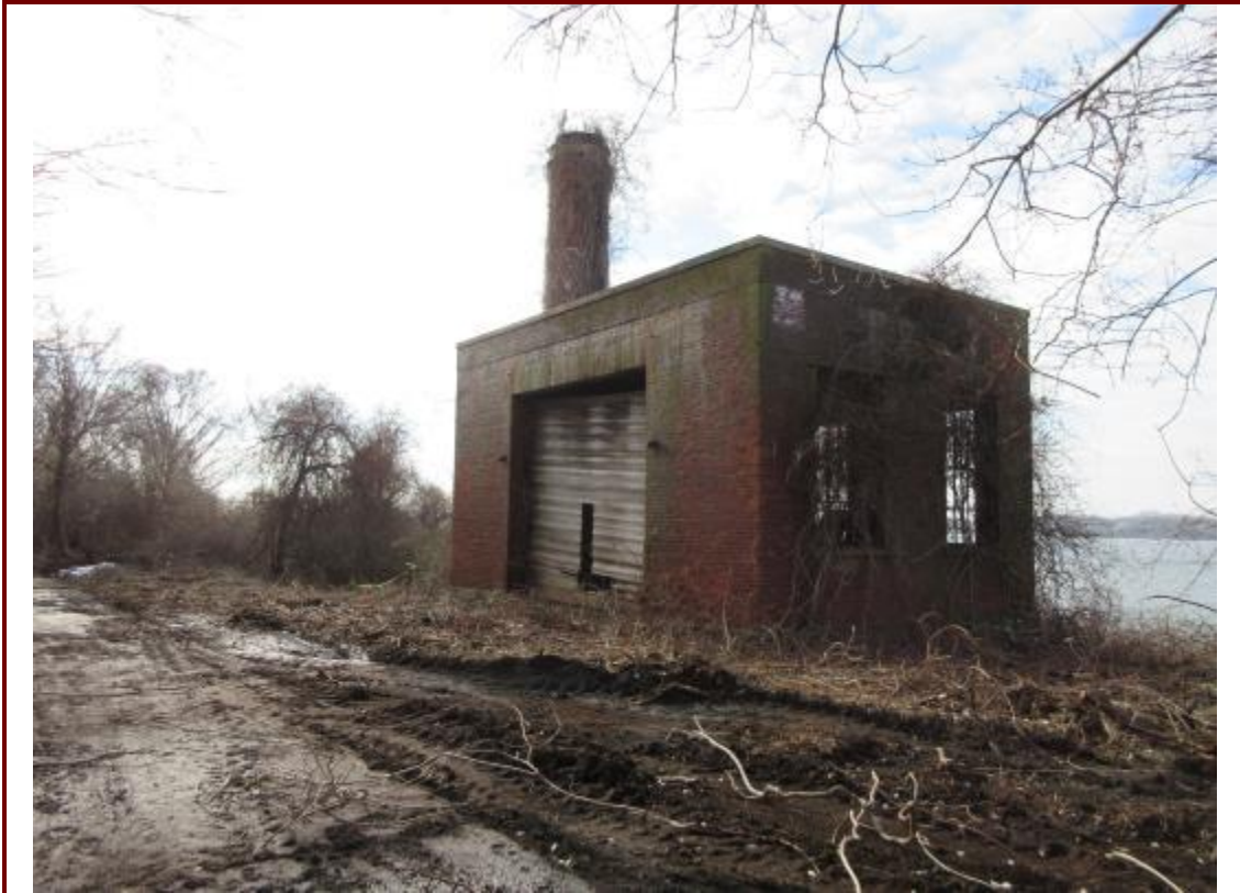
3. NED Site 8 Incinerator.
