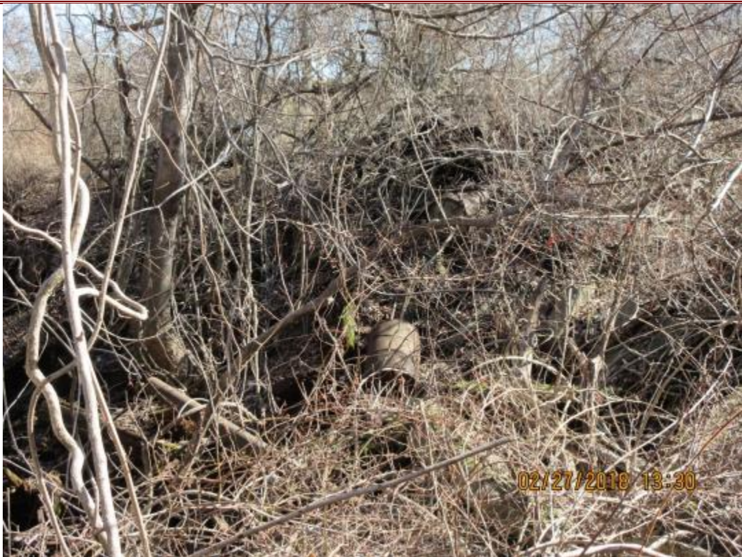
42. Drums and debris in bunkers.
