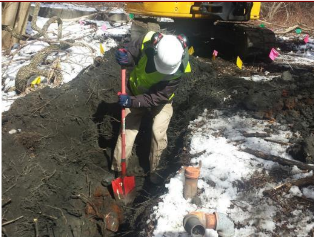
96. Test pit to located suspect UST between buildings 37 and 38.
