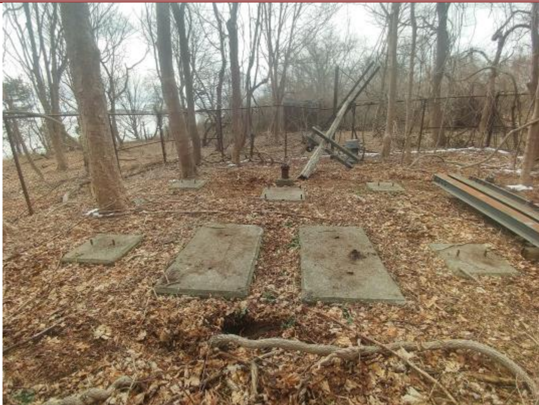
138. Concrete pad layout in NED Site 13 substation/transformer pen.
