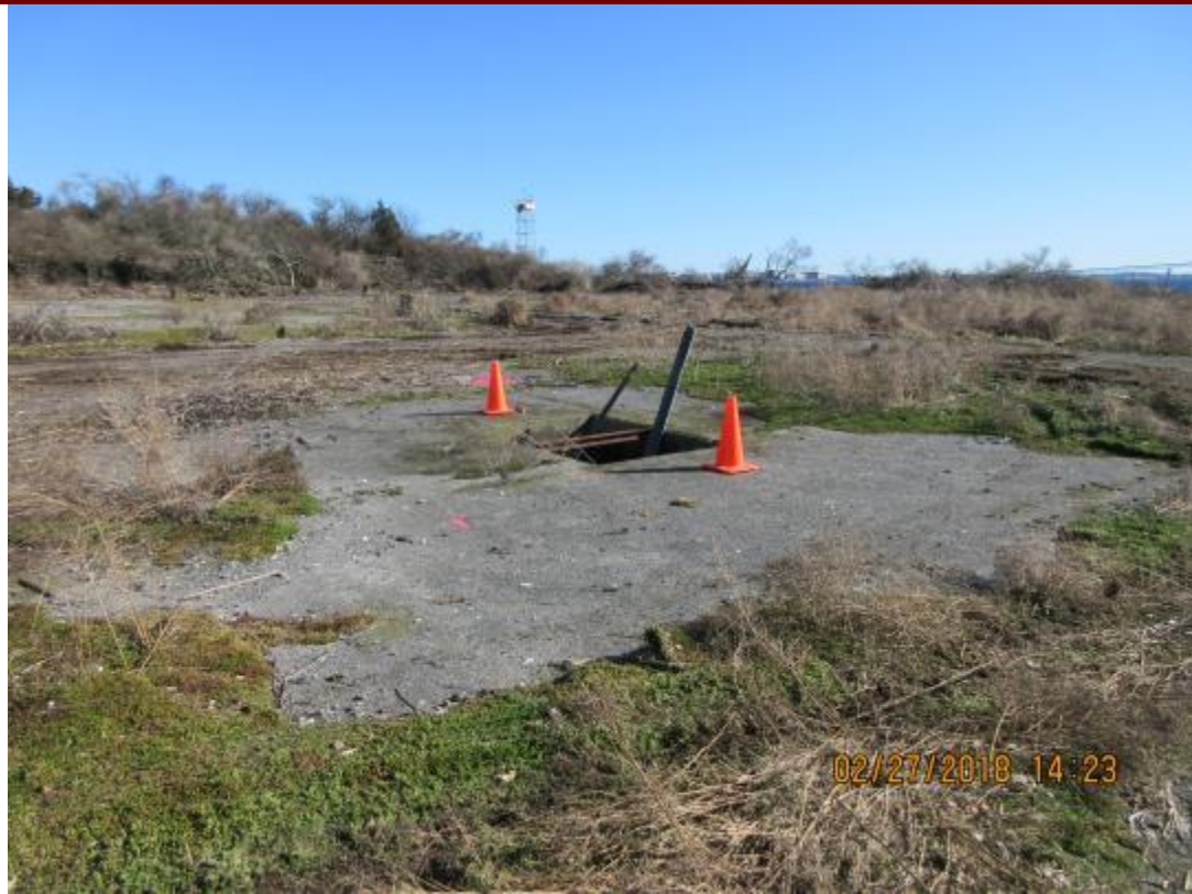
55. NED Site No. 43 Boiler House and Ordnance Test Facility location prior to construction of existing aviation pad.
