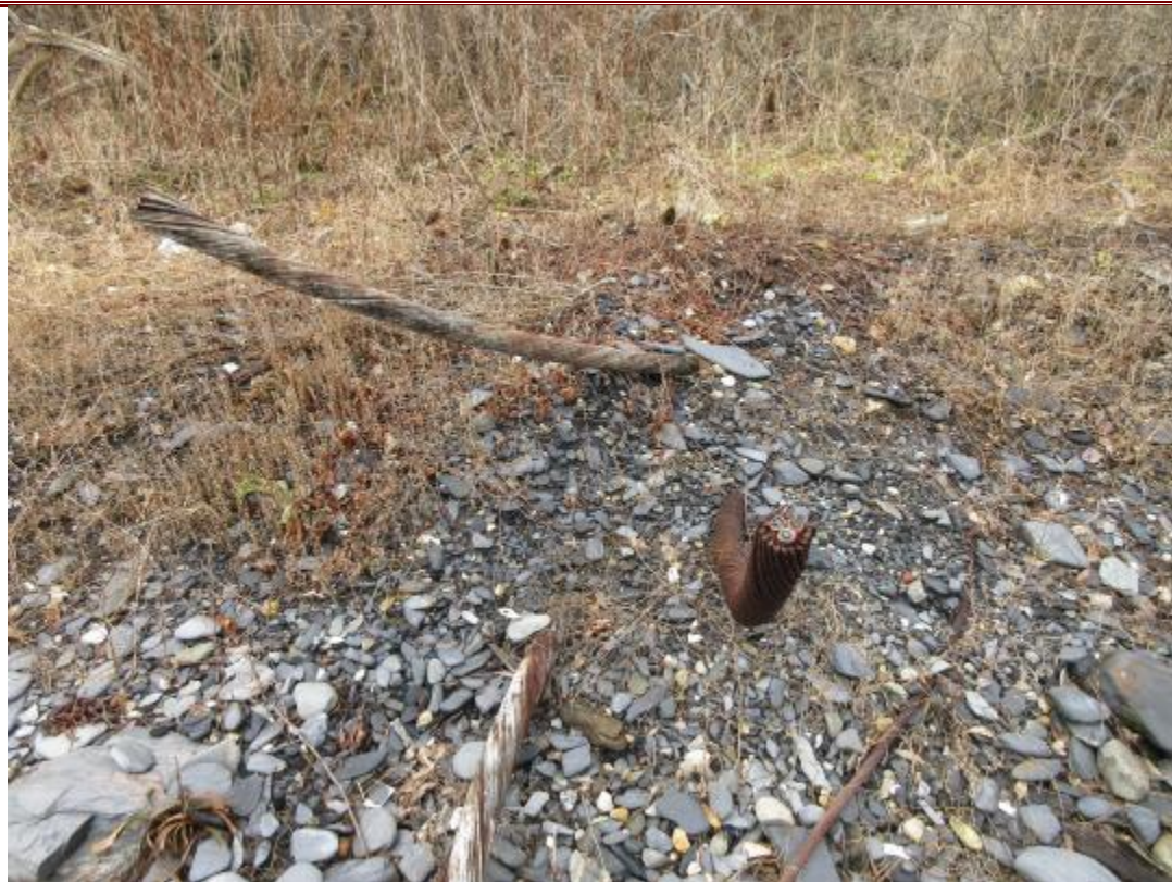
46. Cables that extent to Cable Terminal Building extending east from island.
