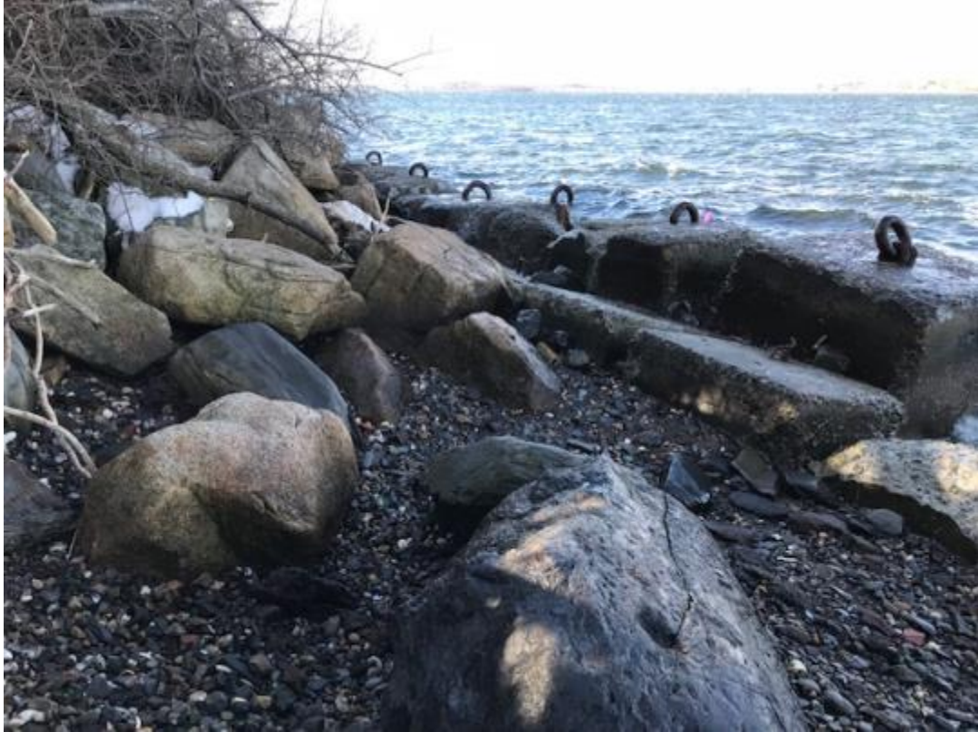
89. Large concrete blocks limiting access to central portion of Disposal Area 14. Note tide level relative to blocks.
