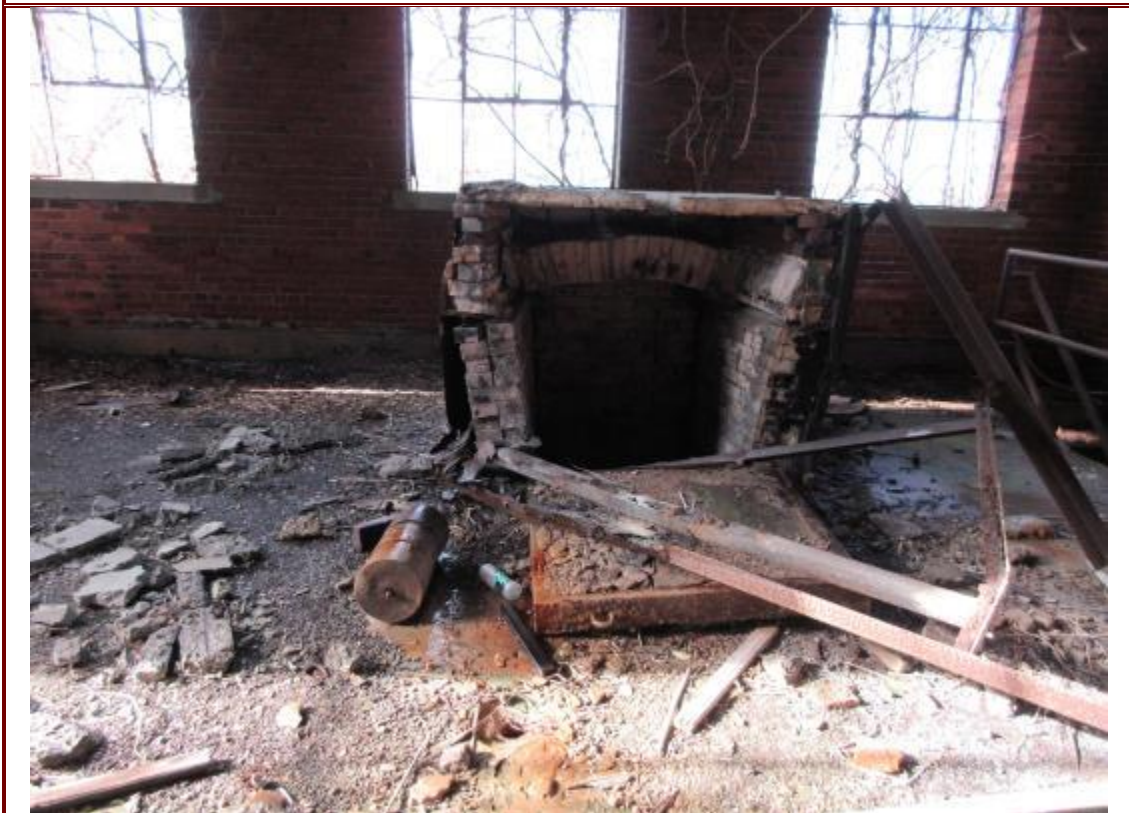
4. Incinerator box on entry floor of incinerator (NED Site No. 8).
