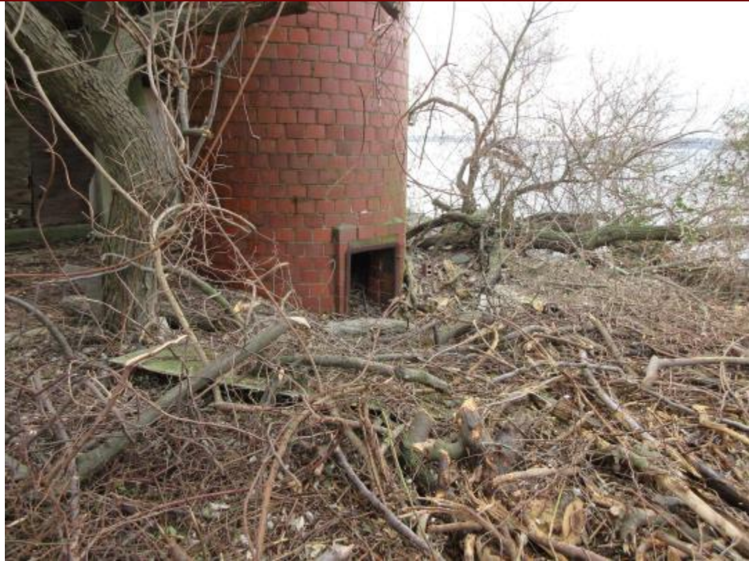
57. NED Site No. 35 Boiler House stack.
