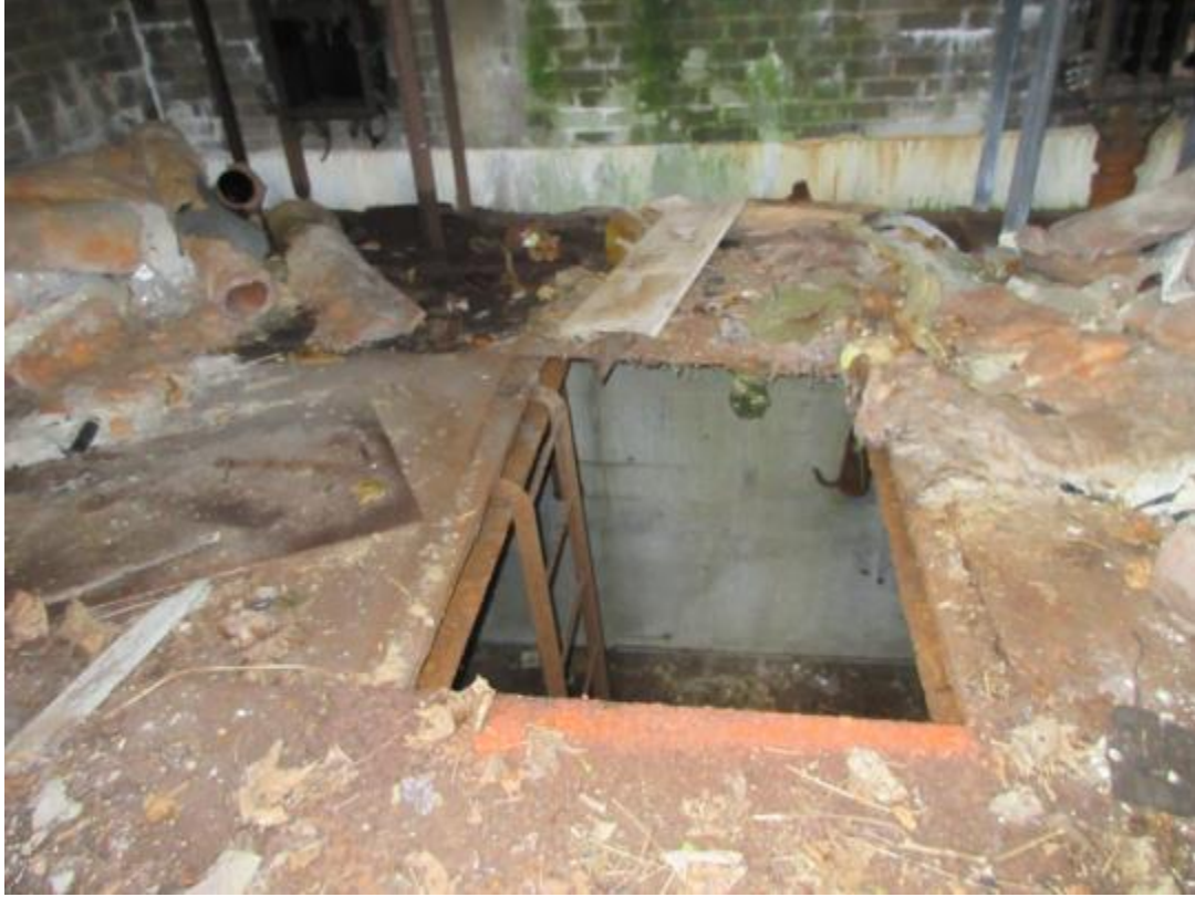
73. Pit in NED Site No. 39 Well House.
