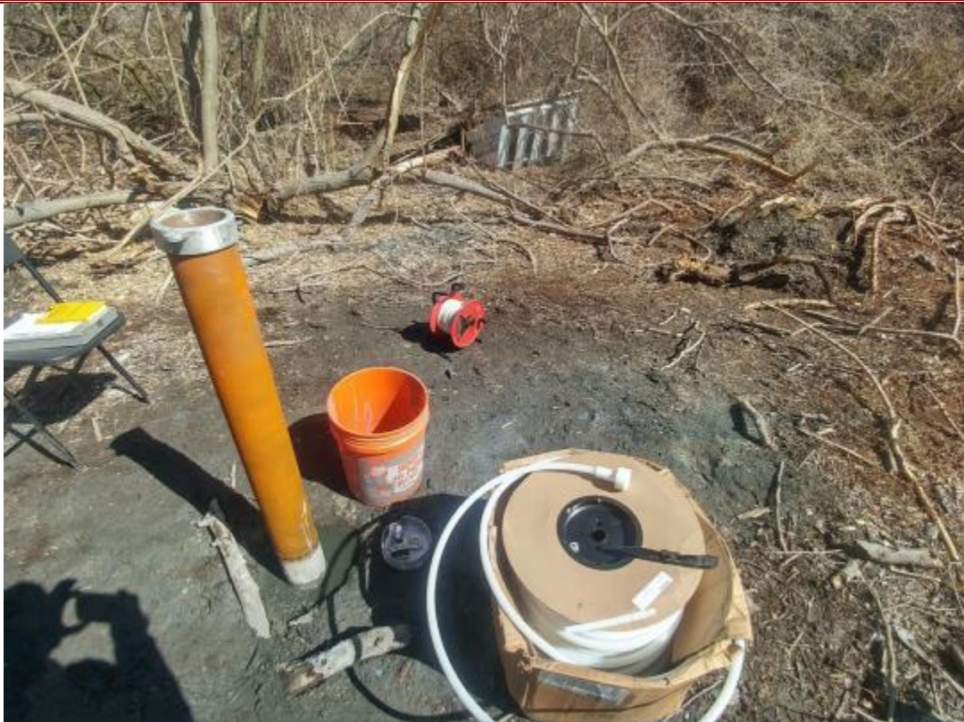
100. BMW-3 during setup for well development activities.
