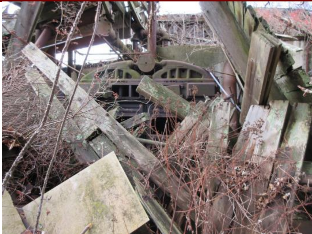
58. NED Site No. 35 Boiler House fire boxes.
