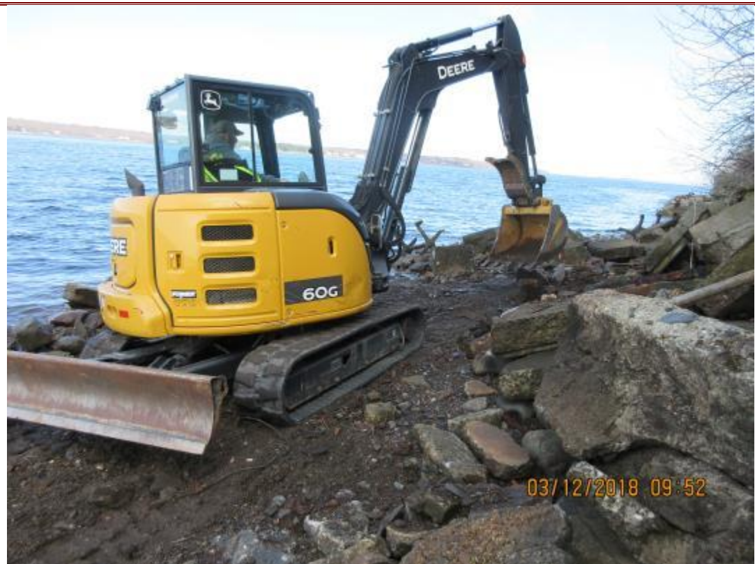
122. Location of 10TP6 at northernmost accessible extent with the excavator. Note water adjacent at low tide.
