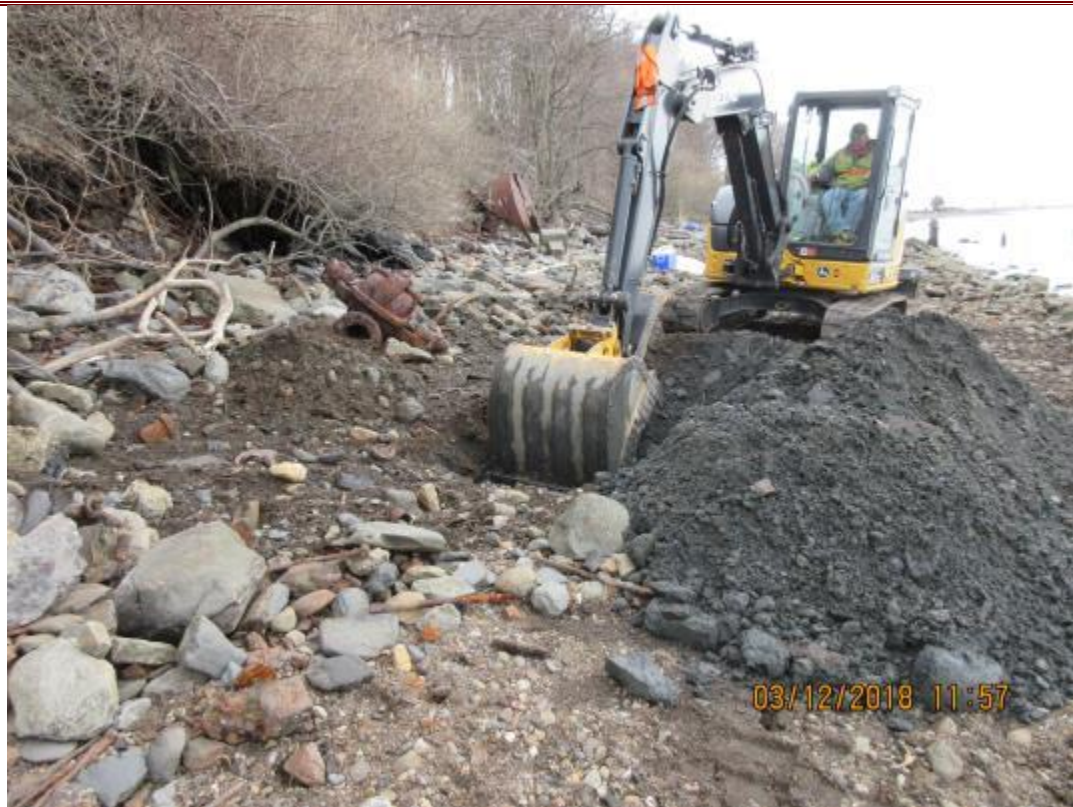
128. Location of 10TP8 facing south.
