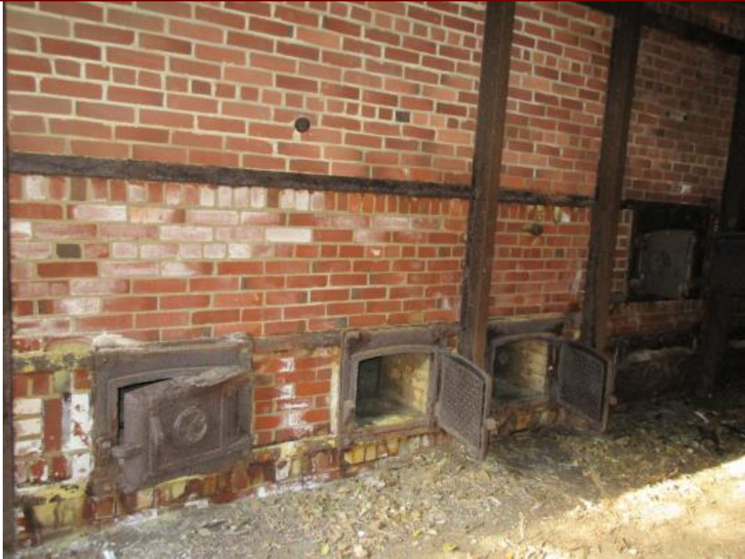
5. Fire boxes on bottom floor of Incinerator (NED Site No. 8).
