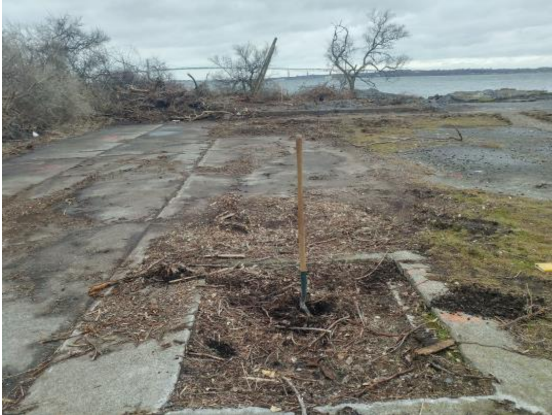
49. NED Site No. 27, presumed gas pit structure. Second pit associated with NED Site No. 27 is in background.
