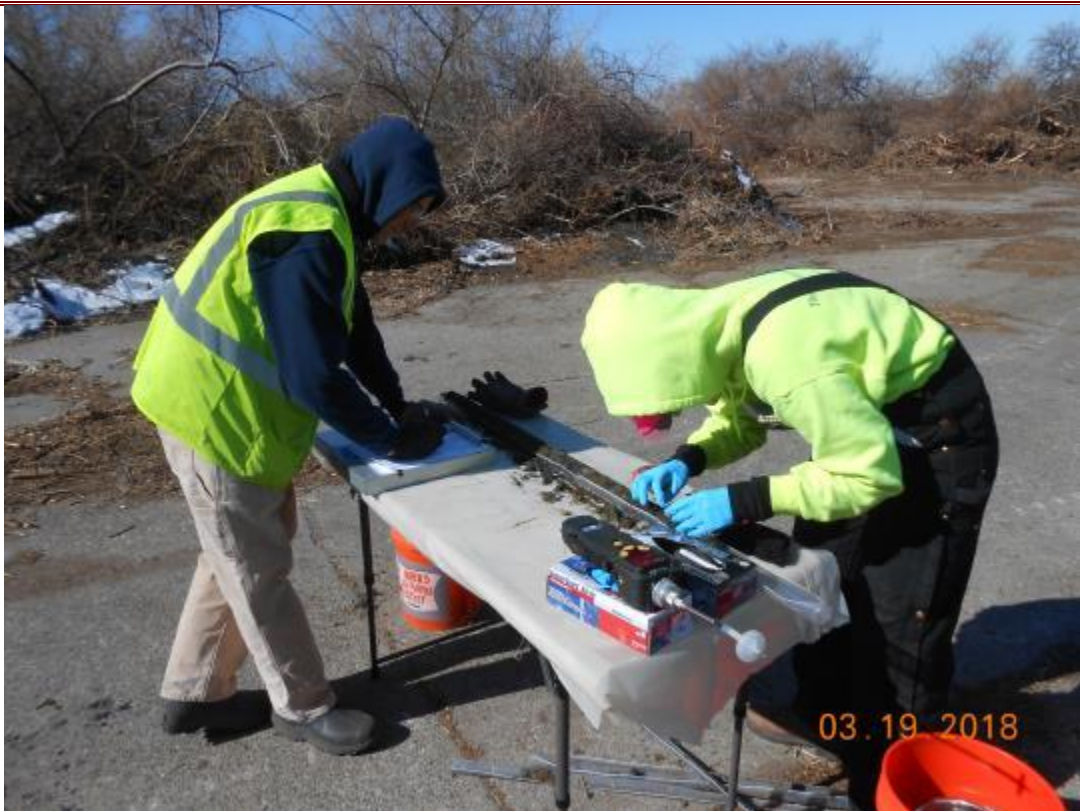
110. Credere staff characterizing soil during boring at NED Site 1.
