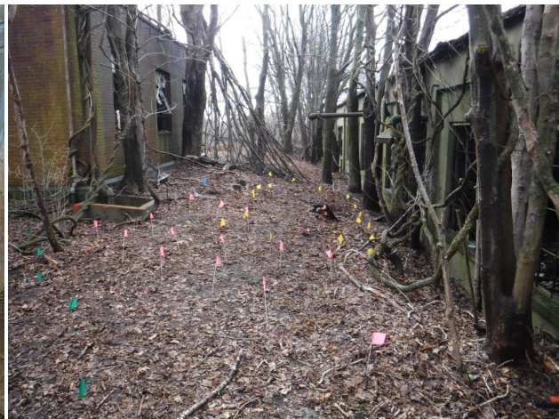
Photograph 4. Between Buildings 37 and 38, view to the south. Buildings 37 and 38 are on the left and right of the photograph, respectively. The probable UST detected in the area of interest is marked with yellow pin flags in the center of the photograph. The green flags in the bottom left of the photograph mark the limit of a septic vault, and the pink flags mark possible utilities.
