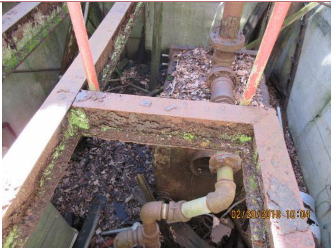
22. Boiler inside northeast corner of building associated with UST.
