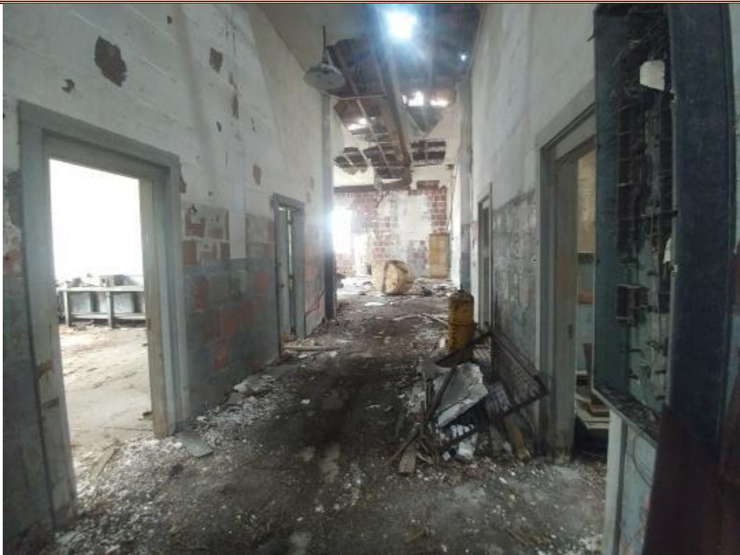
66. Interior of NED Site No. 38 Torpedo Storage building.
