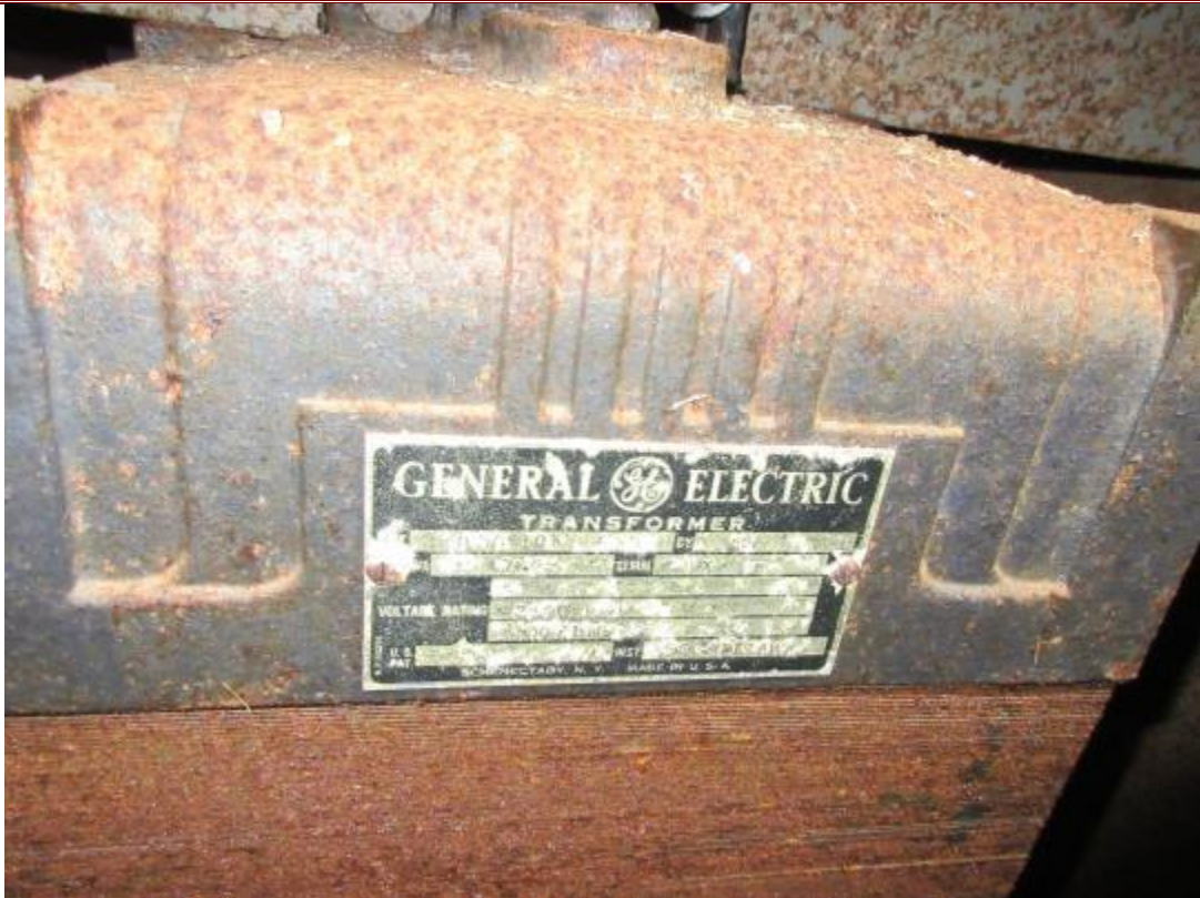
28. Transformers inside NED Site No. 13 building.
