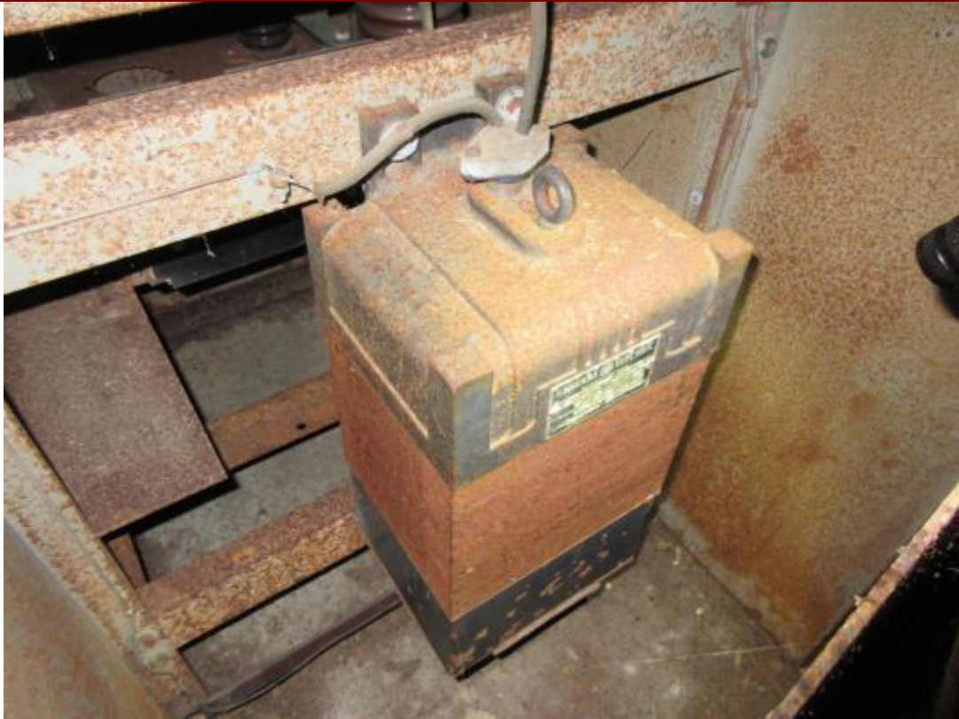
27. Transformers inside NED Site No. 13 building.
