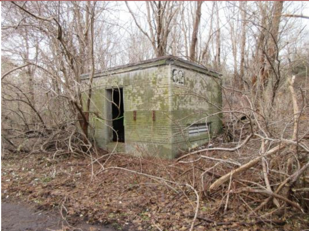
72. NED Site No. 39 Well House (Building 62).
