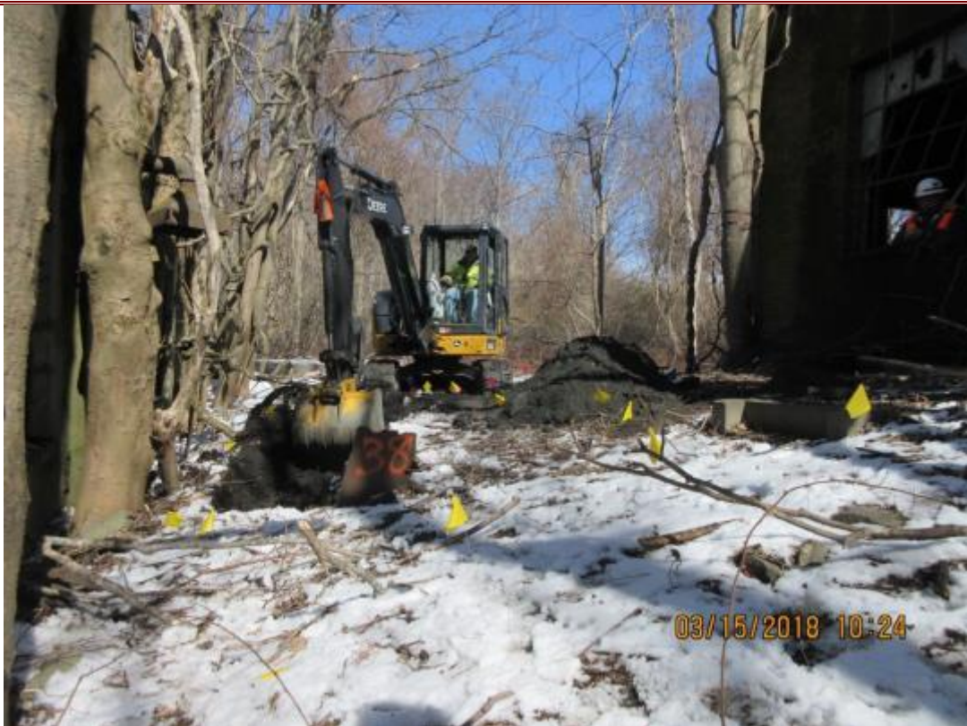
94. Excavation of suspect UST between buildings 34 and 38.
