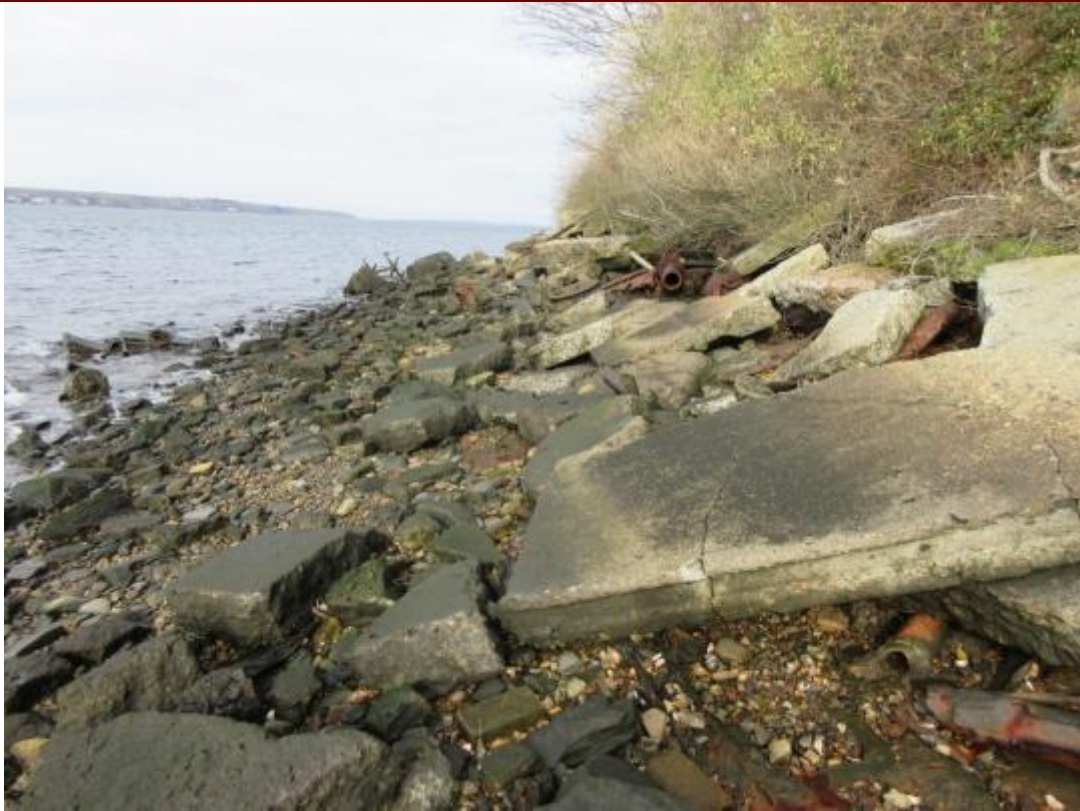
87. Large concrete slabs and blocks on west beach
