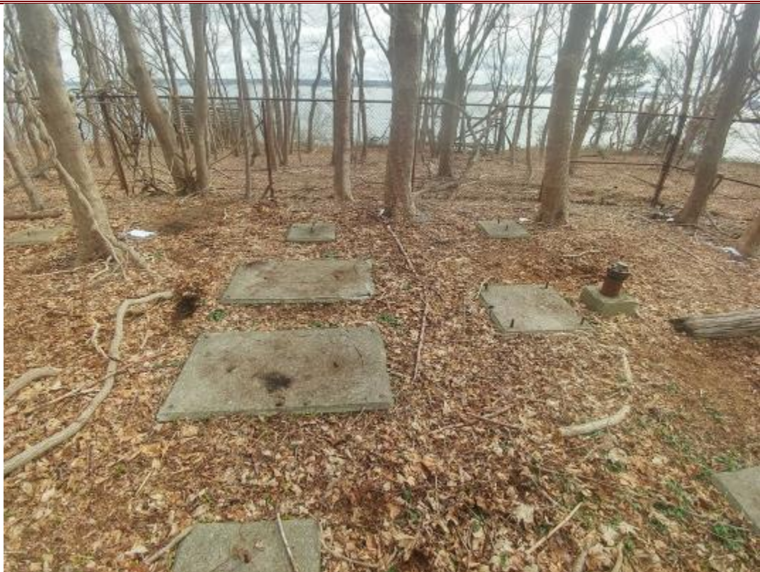
142. Concrete pad layout in NED Site 13 substation/transformer pen.
