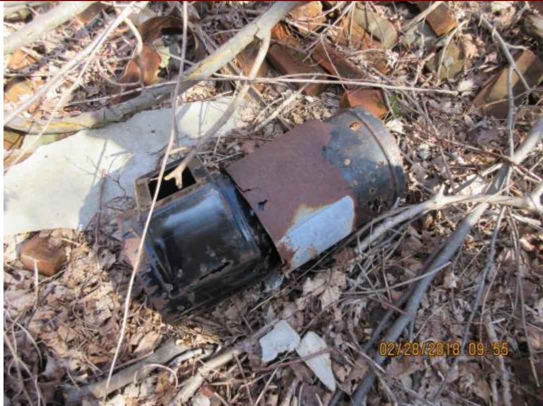
79. NED Site No. 49 Water Tower Pump House, boiler transformer.
