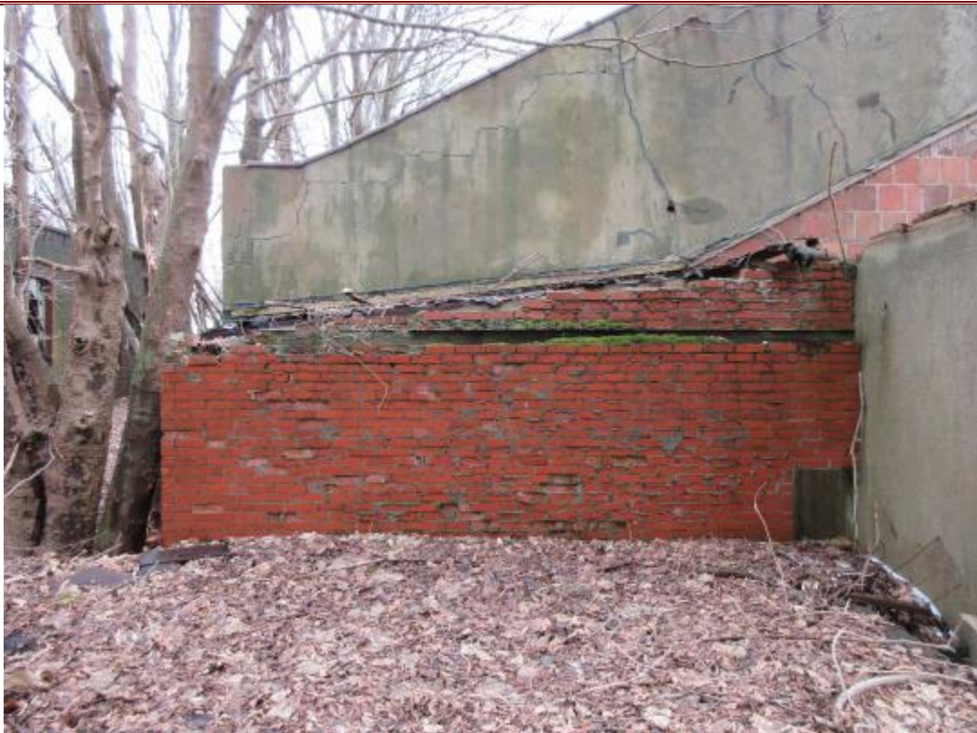
68. Transformer house on north end of NED Site No. 38 Torpedo Storage building.
