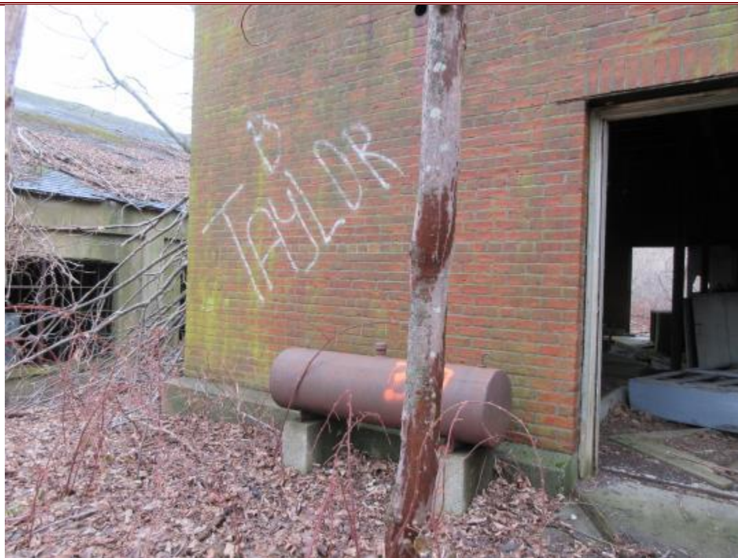
60. Tank (1 of 2) outside NED Site 37 Misc. Storage Building.
