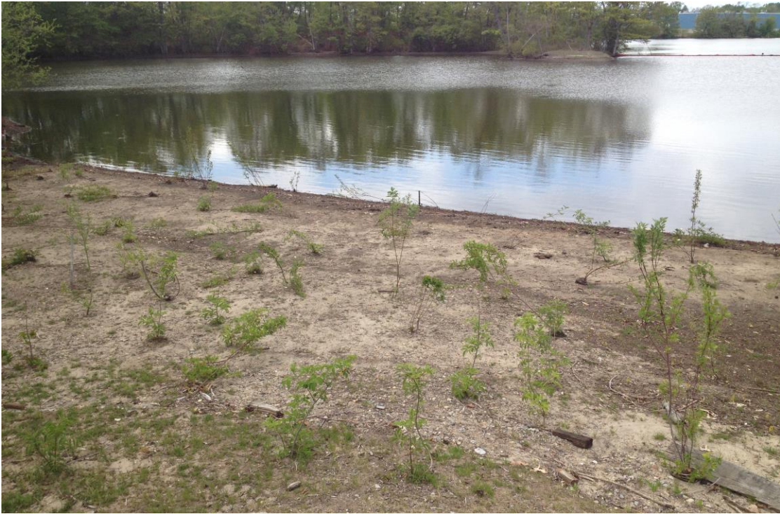
Photo #3: Phase I Area Fringe Wetland requires reseeding with Wetland Mix, facing Northeast
