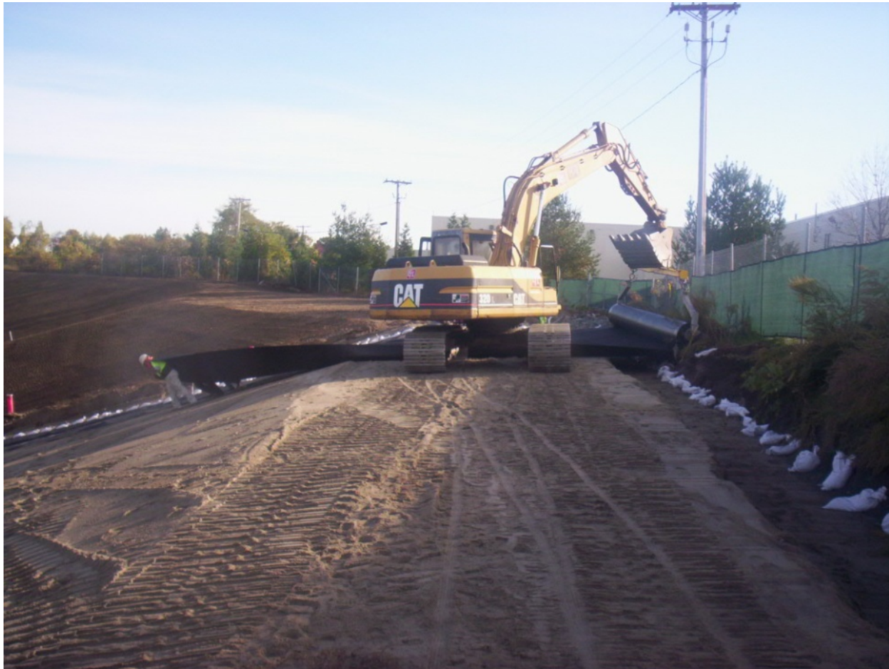
Date Photo ID Description 10/23/12 1578 Begin installing geomembrane at Area 4, looking east
