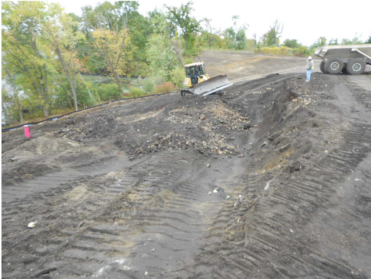
Date Photo ID Description 10/09/12 1031 Re-grading industrial fill at Area 5 with dozer, looking northeast
