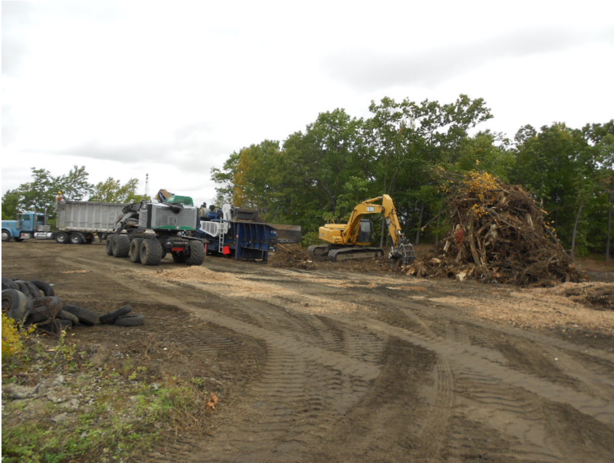
Date Photo ID Description 09/28/12 0963 Wagner Wood shearing stumps for chipping, looking west
