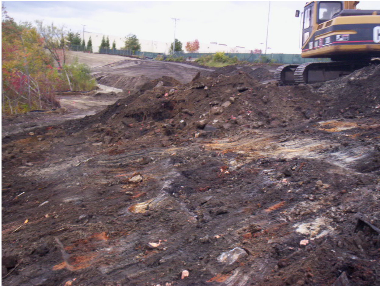
Date Photo ID Description 10/12/12 1044 Grading industrial debris with the excavator at Area 3, looking east
