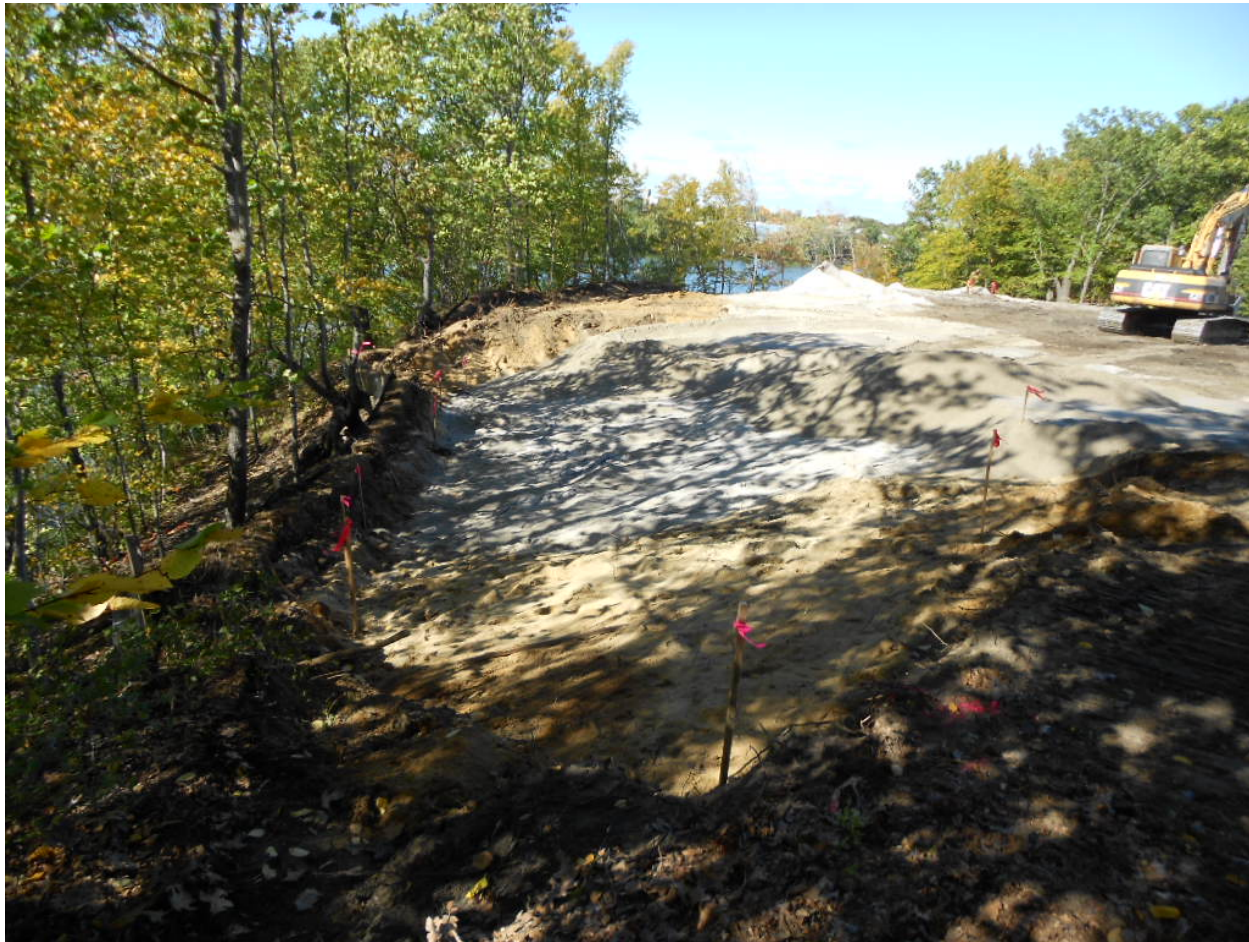
Date Photo ID Description 10/01/12 0976 Backfilling Area 2 with cover soil, looking northwest
