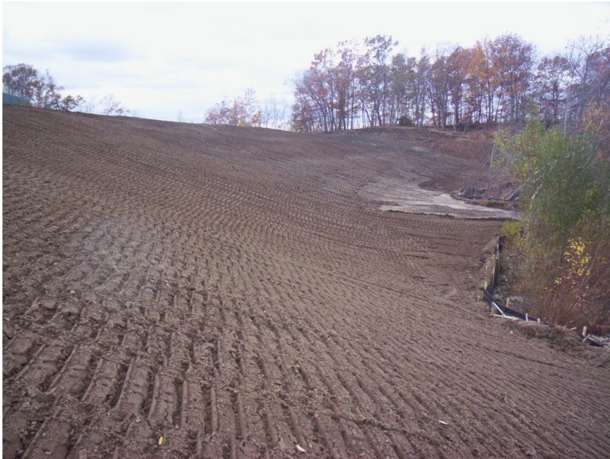
Date Photo ID Description 11/02/12 1656 Looking southwest at Areas 3 and 4. Final grading achieved.
