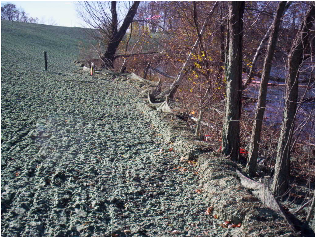
Date Photo ID Description 11/09/12 1682 Toe of slope at Area 5 after Nor'easter, looking southwest
