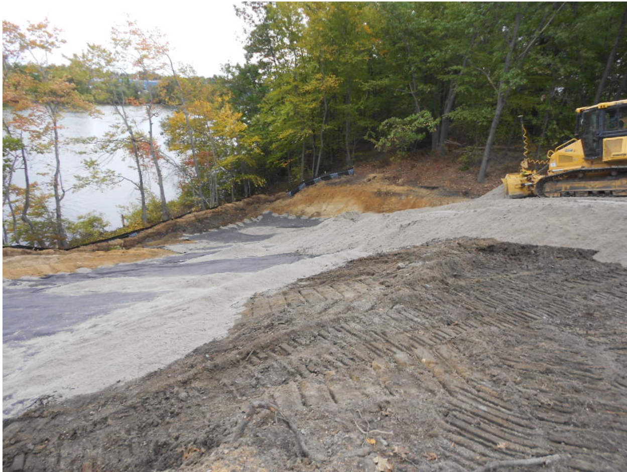
Date Photo ID Description 09/28/12 0965 Placing cover soil at Area 2, looking west
