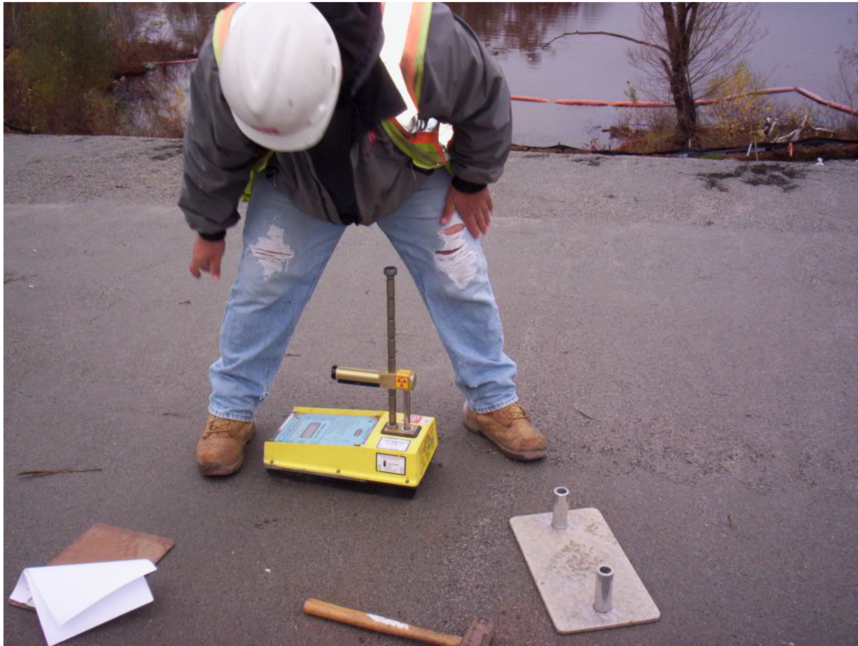
Date Photo ID Description 10/31/12 1630 Compaction testing on the protective soil at the top of the slope at Area 4
