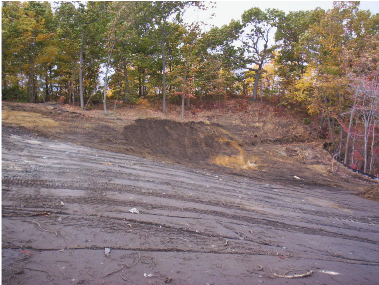
Date Photo ID Description 10/19/12 1566 Sub-grading at Area 3, looking west
