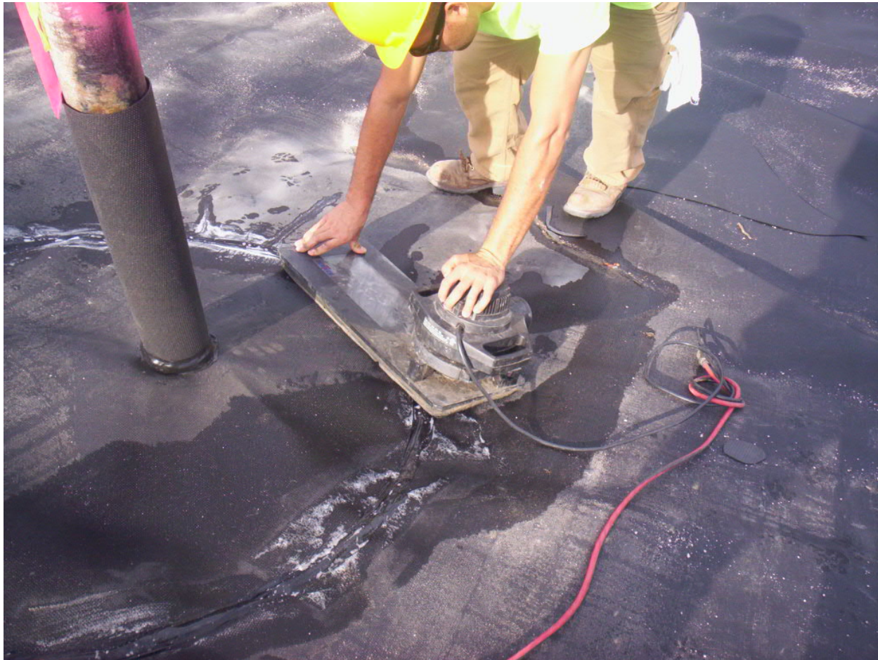
Date Photo ID Description 10/23/12 1593 Vacuum test for extrusion weld for boot at monitoring well
