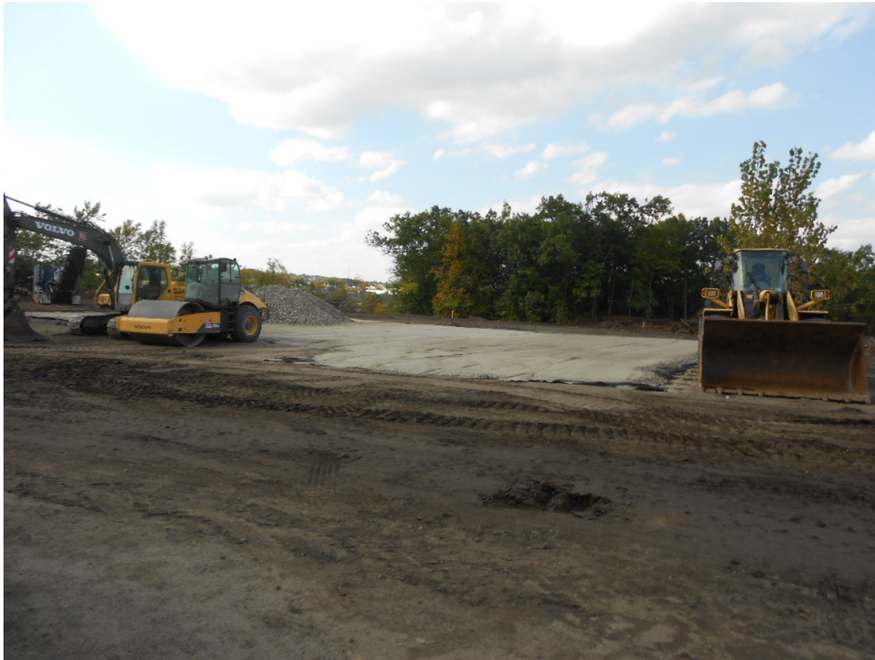
Date Photo ID Description 09/27/12 0962 Lay down area extended, looking south
