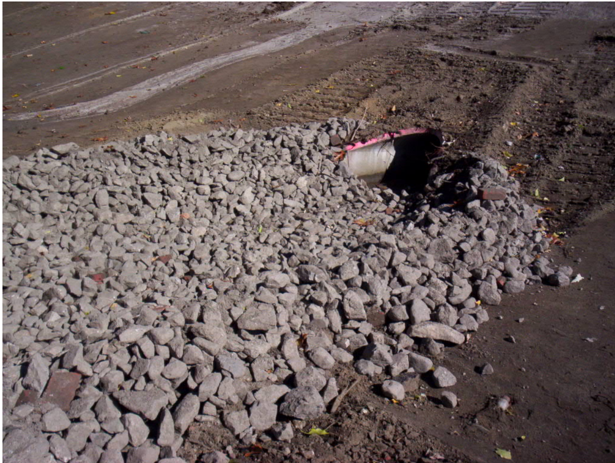
Date Photo ID Description 10/16/12 1555 Rip rap placed at the storm drain (from the detention basin) outlet
