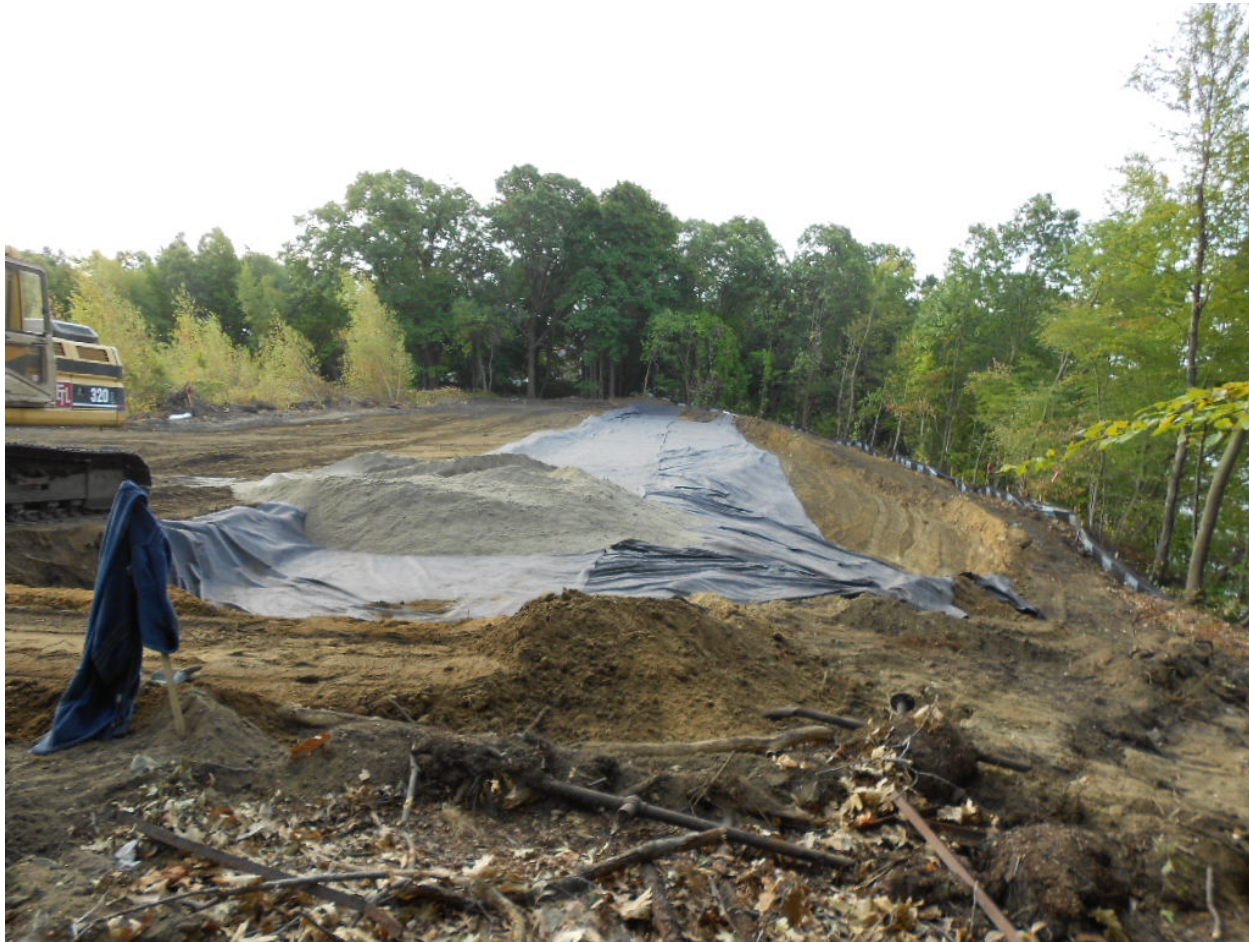
Date Photo ID Description 09/26/12 0947 Cover soil and geotextile installed at Area 1, looking south
