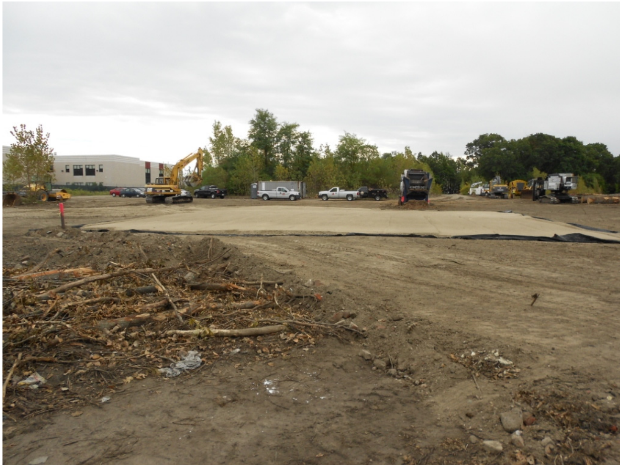
Date Photo ID Description 09/24/12 0921 Looking southeast at the lay down area
