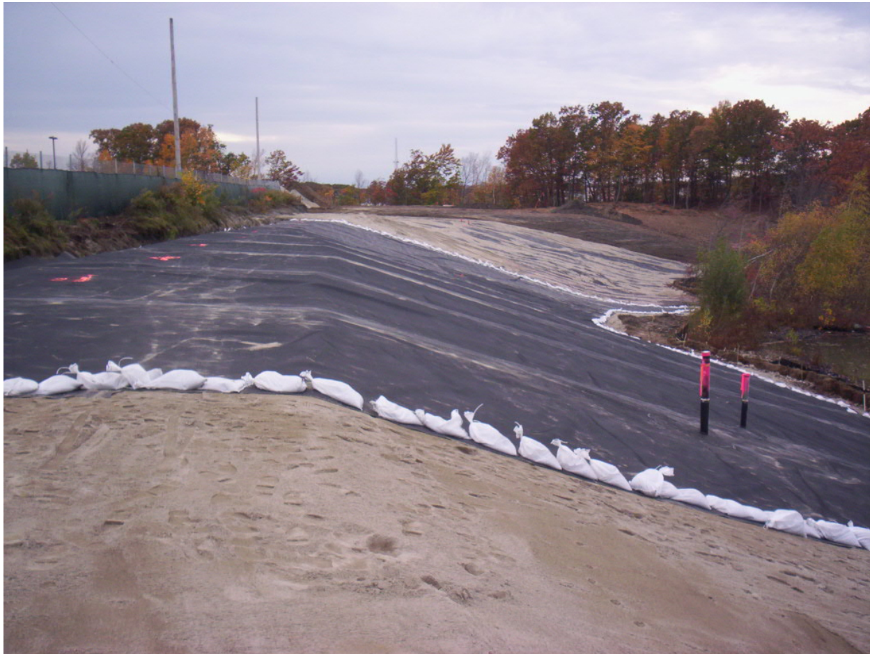
Date Photo ID Description 10/23/12 1597 Looking southwest at the installed geomembrane at Area 4
