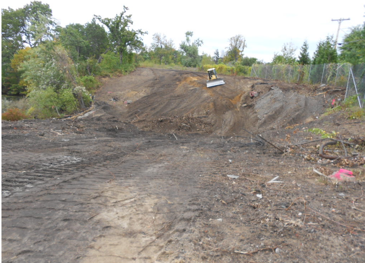
Date Photo ID Description 09/28/12 0966 Dozer grading sub-grade at Area 5, looking northeast
