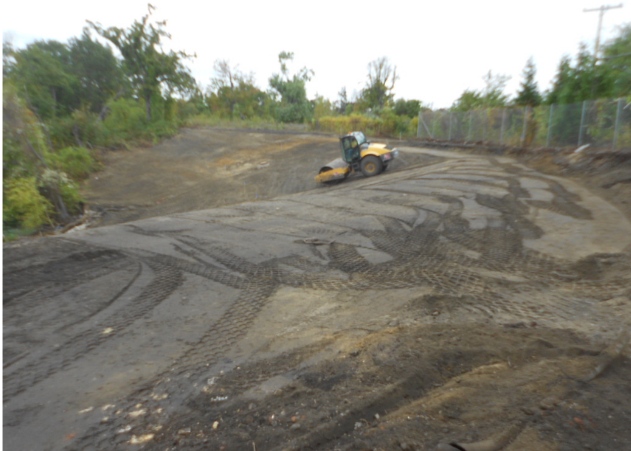
Date Photo ID Description 10/09/12 1029 Roller compacting sub-grade at Area 5, looking northeast
