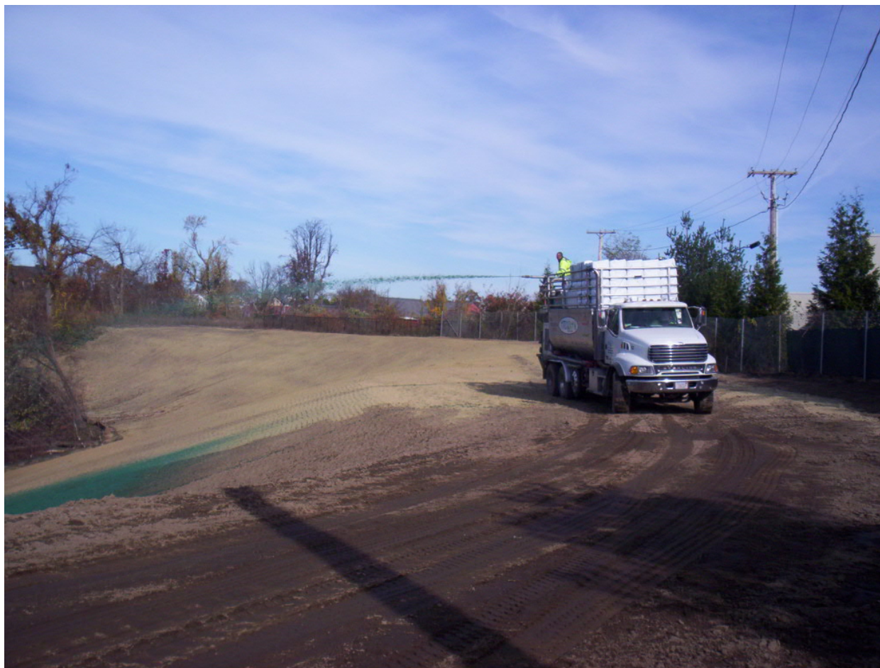
Date Photo ID Description 11/06/12 1662 Hydrograss hydroseeding Area 4, looking northeast
