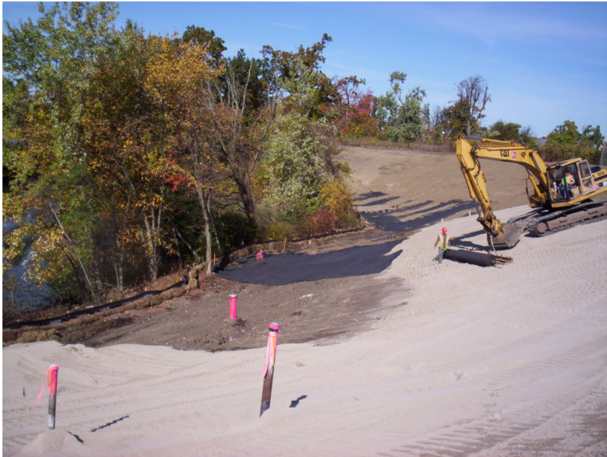
Date Photo ID Description 10/17/12 1562 Installing geotextile at the wetland buffer cap at Area 5, looking northeast
