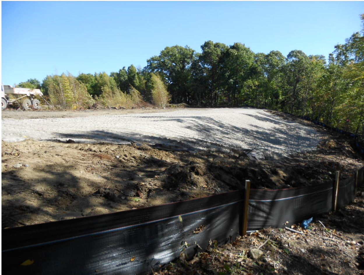
Date Photo ID Description 10/01/12 0977 Area 1 backfilled with cover soil, looking southeast
