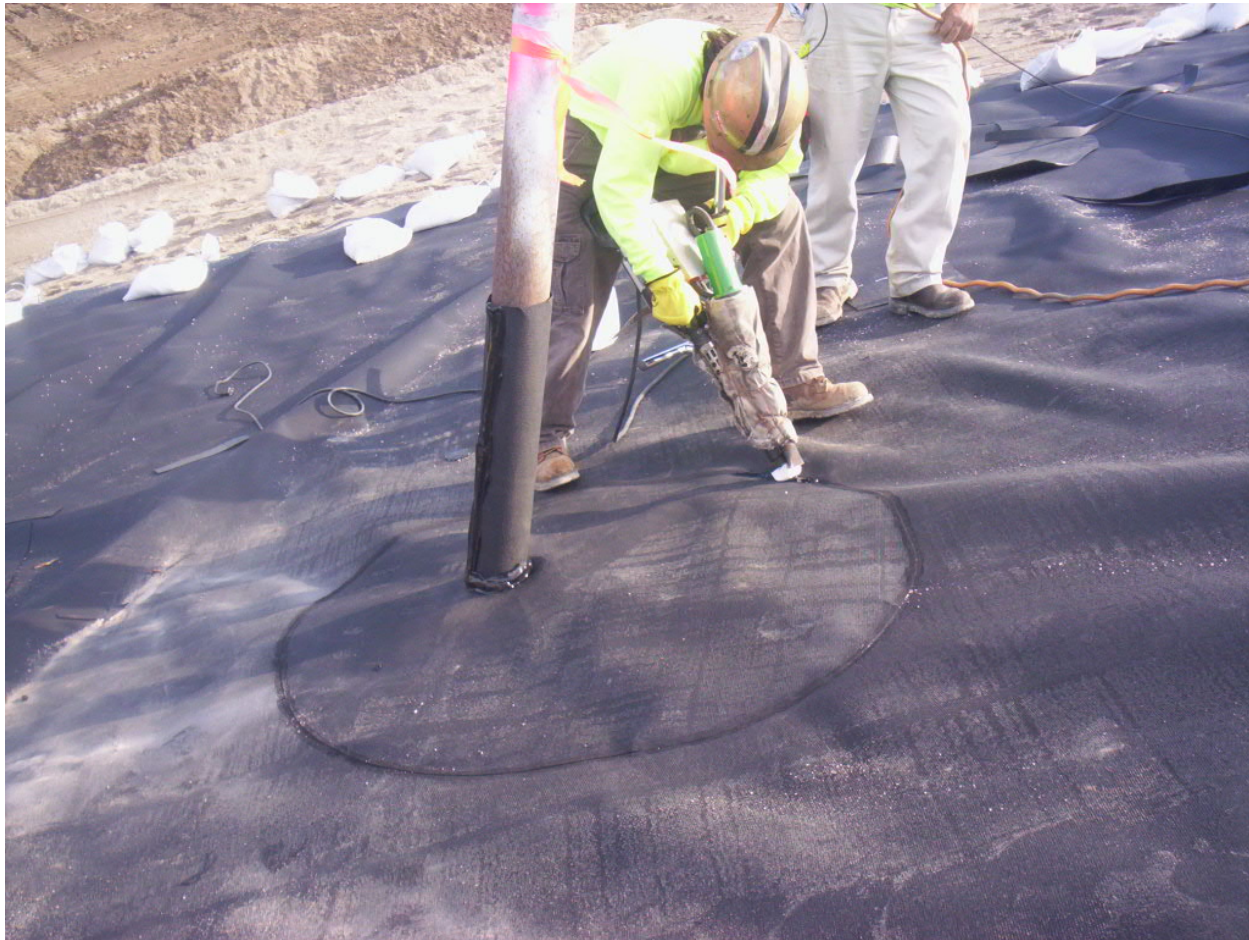
Date Photo ID Description 10/23/12 1586 Extrusion welding boot for monitoring well
