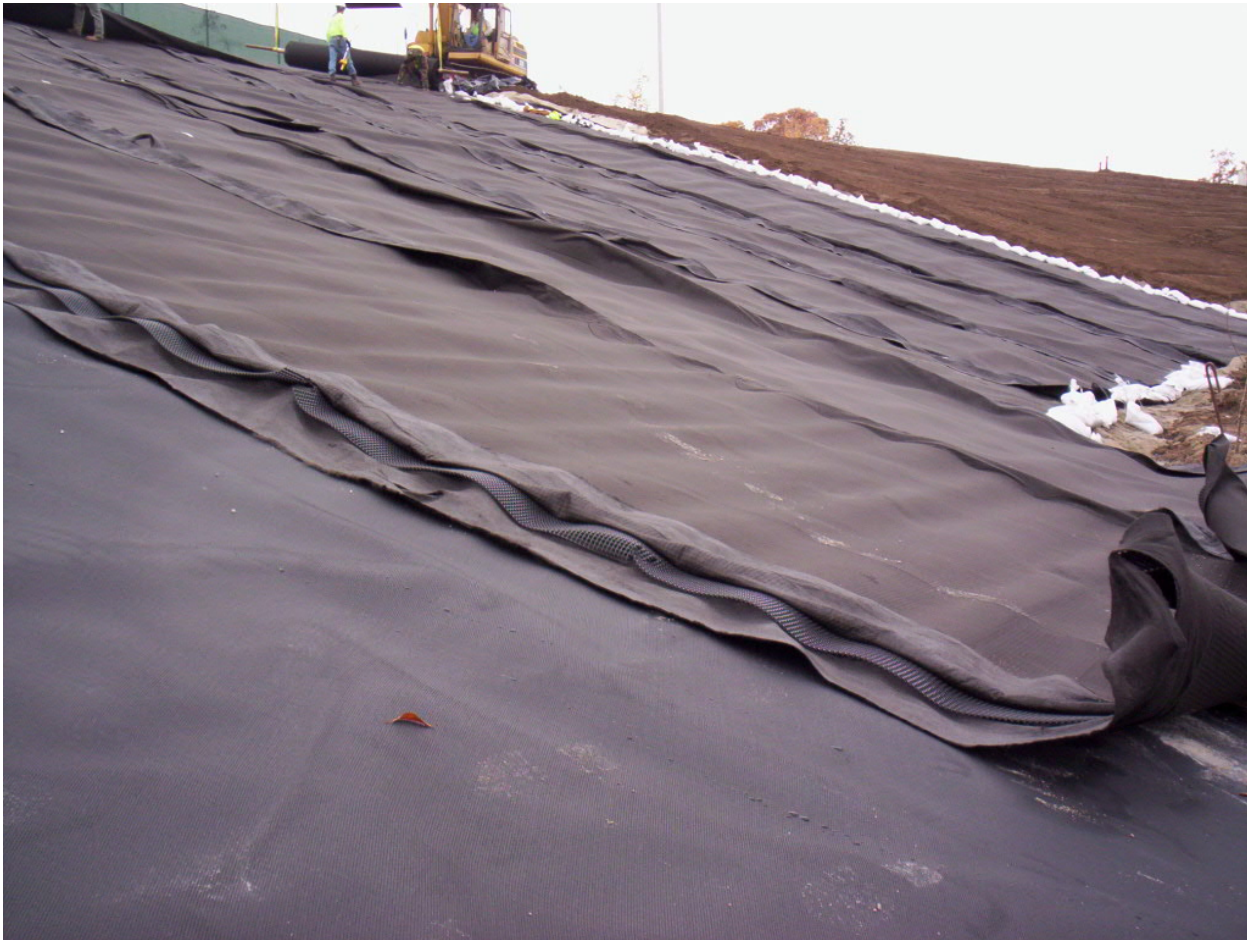
Date Photo ID Description 10/26/12 1606 Drainage geocomposite installation at Area 4, looking southwest
