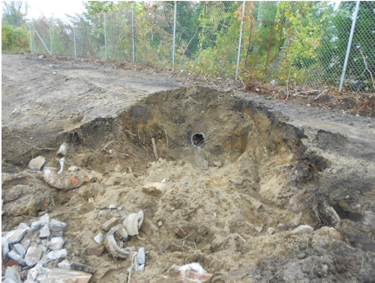
Date Photo ID Description 10/03/12 1001 Storm drain to be plugged at the top of the bank in Area 5, looking east
