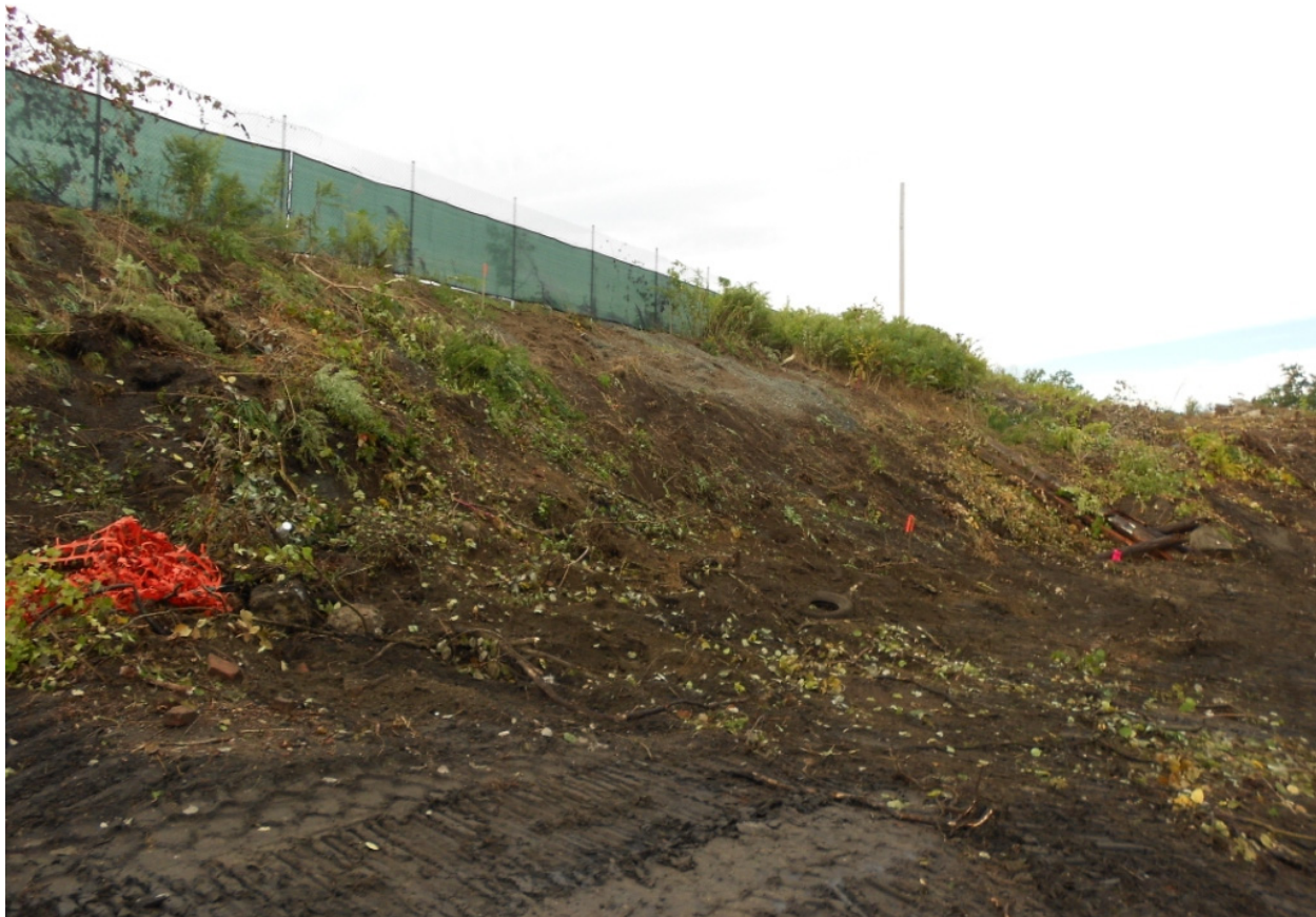
Date Photo ID Description 09/21/12 0895 Looking southwest at the cleared slopes north of the HS
