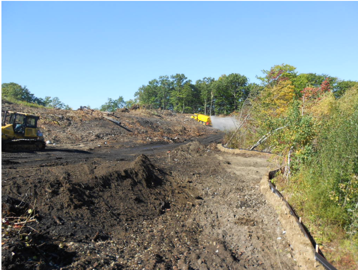
Date Photo ID Description 09/25/12 0940 Water truck applying dust control at Areas 3 and 4, looking south
