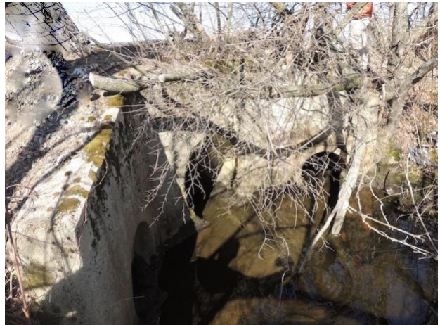
Culverts along west bank of river near site of DV-01b
