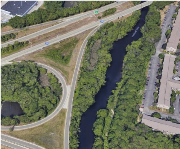
Site of DV-01a near Villa Del Rio Apartments looking upriver
