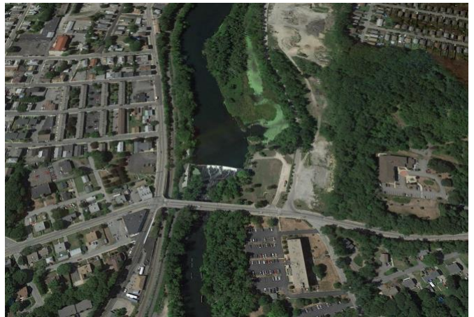
Manville Landing and Dam at site of DV-01 looking upriver
