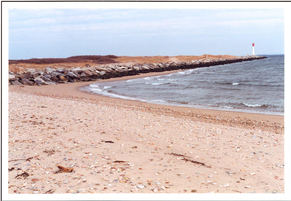
Looking NNW from CP-1 at low tide on 24 March 1999, Great Salt Pond (#1), Block Island.
