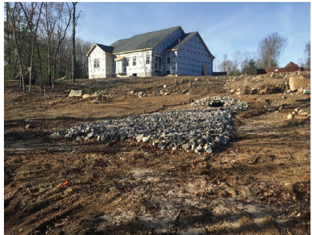
IMAGE TAKEN DURING INSPECTION OF A CONSTRUCTION PROJECT IN COVENTRY WITH INSUFFICIENT DRAINAGE STRUCTURES NEAR WETLANDS.
