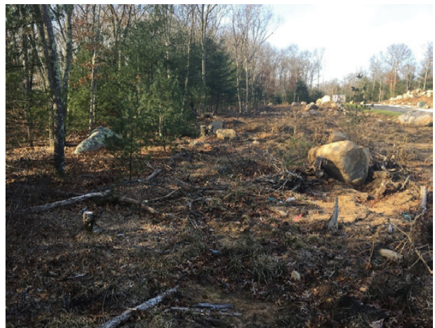
IMAGE TAKEN DURING INSPECTION OF A CONSTRUCTION PROJECT IN COVENTRY THAT DID NOT INCLUDE REQUIRED EROSION AND SEDIMENT CONTROLS.
