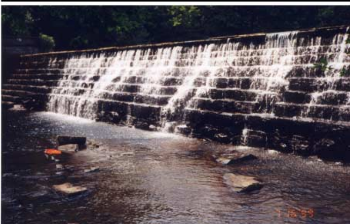
Dam No. 157 - Harris, Coventry
