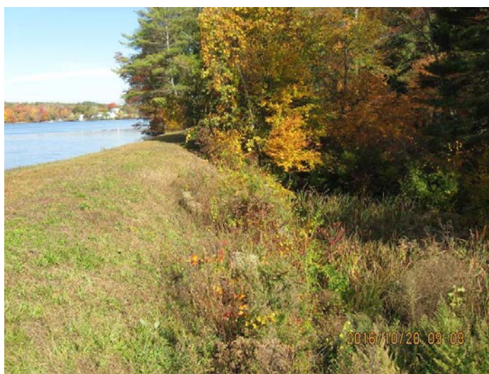
Improper vegetation at Waterman Dam (No. 111) in Gloucester
