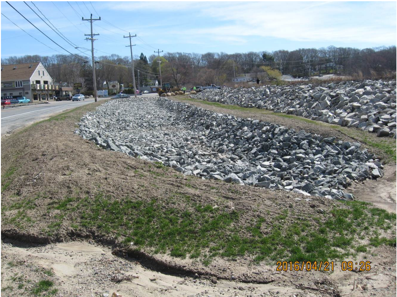
Restored Spillway Channel at Tiogue Lake Dam (No. 177) in Coventry
