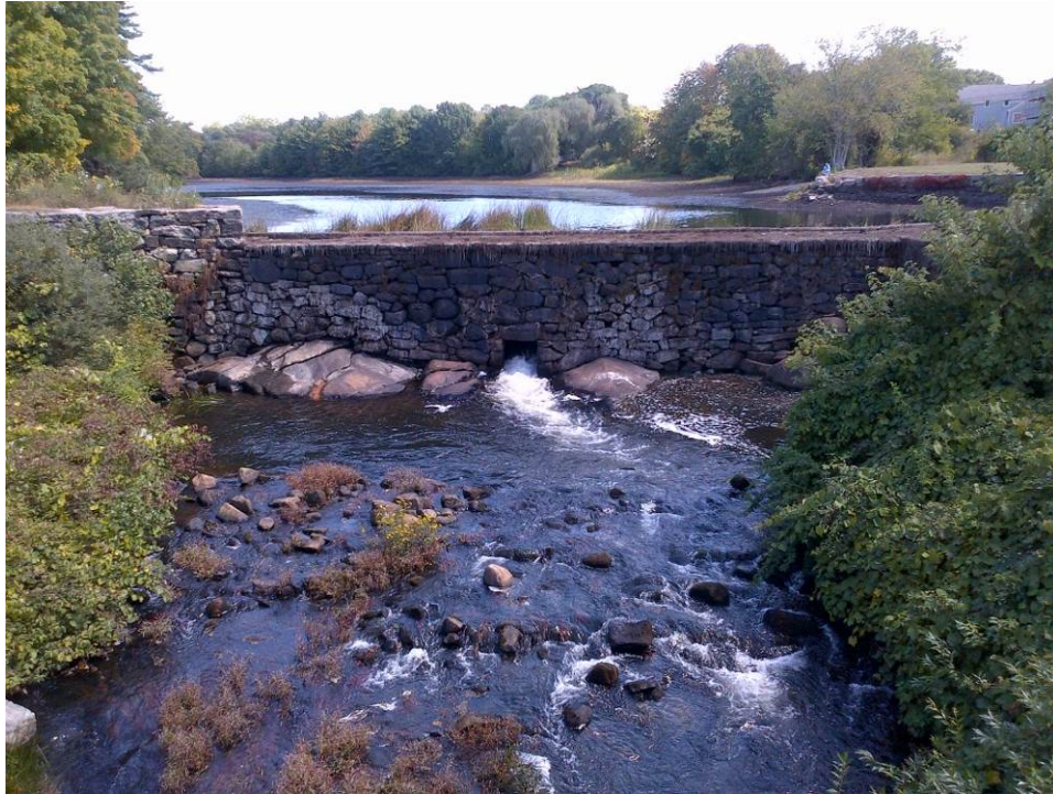
Spillway & leaking low level outlet at Wyoming Upper Dam (No. 216) in Hopkinton/Richmond
