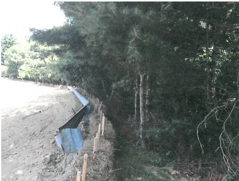
Overgrown downstream side of dike at Gainer Dam (No. 161) in Scituate
