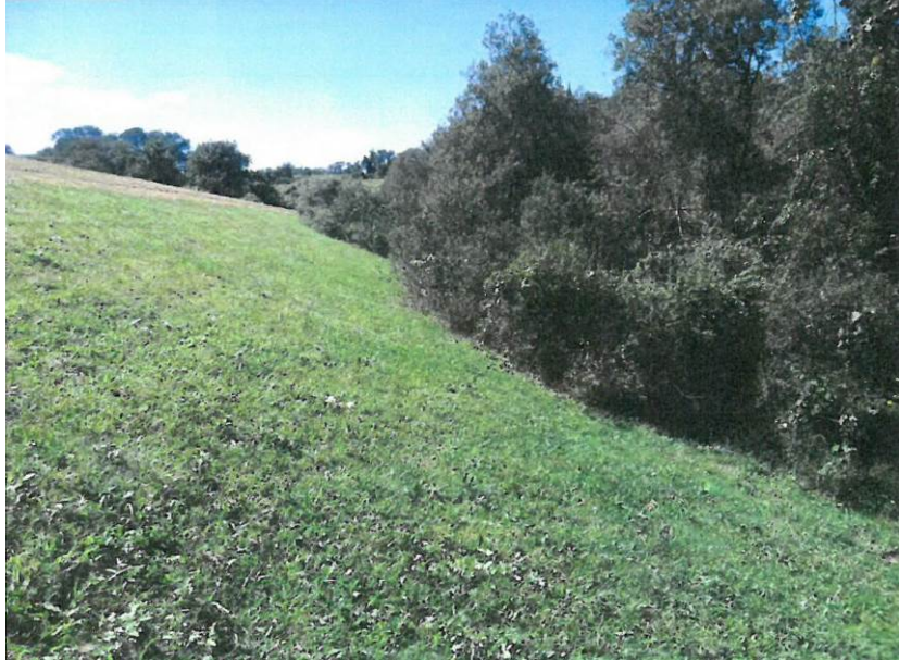
Overgrown downstream slope of Watson Dam (No. 485) in Little Compton
