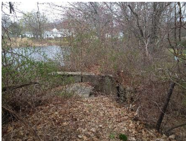
Overgrown Stone Dam (No. 320) in Cranston
