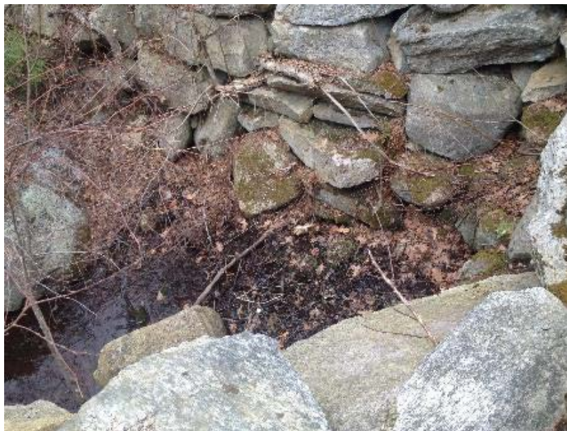
Seepage at base of Wilbur Dam (No. 572) in Burrillville
