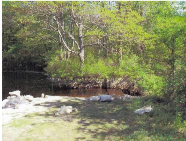
Sand-bagged section (foreground) and overgrown section (background) of the Wincheck Pond Dam (#225) in Hopkinton
