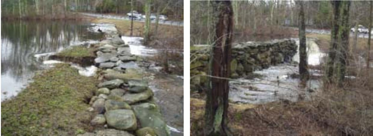
**Breached embankment at Burton Dam (No. 329), Scituate**
