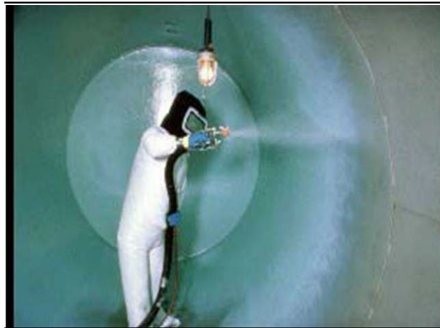
Sample of a Tank being Interior Lined
