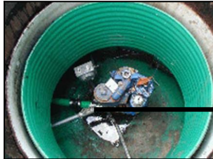
Sample Flexible Piping in a Sump
