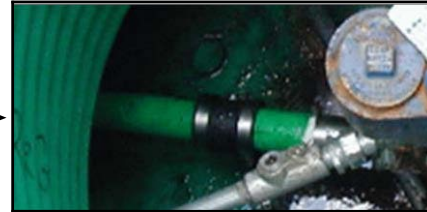
Closeup of Flexible Piping in a Sump
