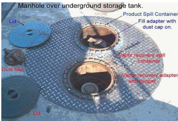
The image to the left shows the location of some Phase I Vapor Recovery System Components
