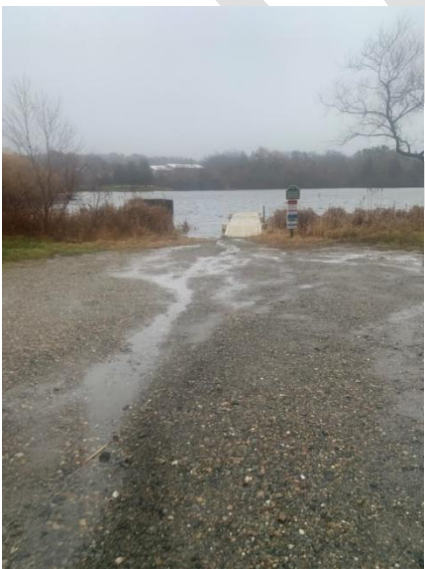
Figure 4.4. Location 2: Runoff from gravel parking area. Photo 12/07/2022.
