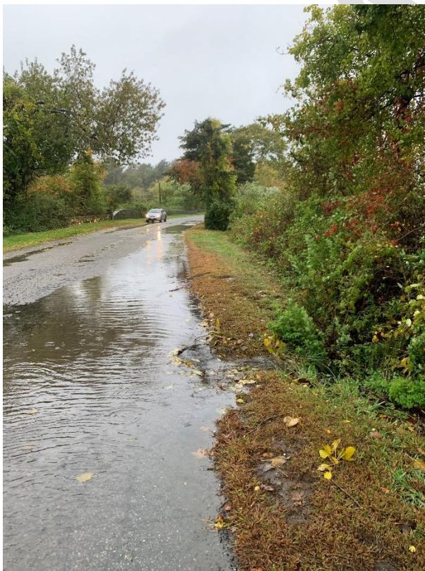
Figure 6.2. Stormwater runoff on Bradford Avenue discharging into Pond 2 via paved swale. Photo 10/14/2022.
