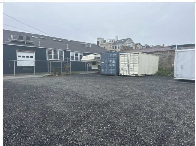
View of temporary cap area.
