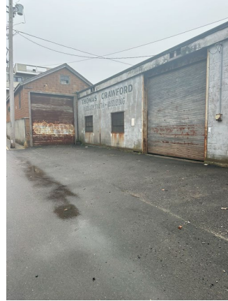
View of temporary cap area.
