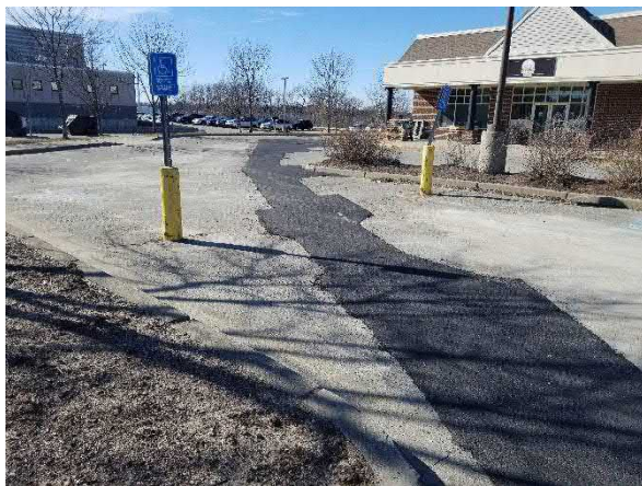
Picture 24: View showing the discharge piping trench completely paved.
