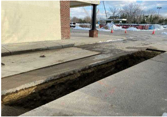
Picture 9: View of trench line west of the building.
