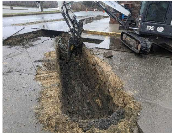
Picture 10: View of trench line south of the building.
