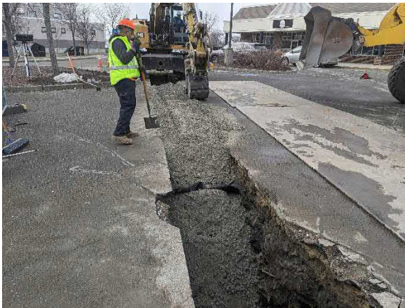
Picture 15: Strategic backfilling and compacting trench with DGA material.
