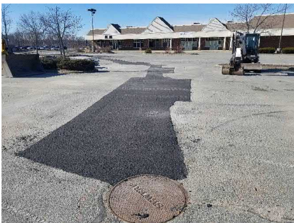
Picture 23: View showing the discharge piping trench completely paved.
