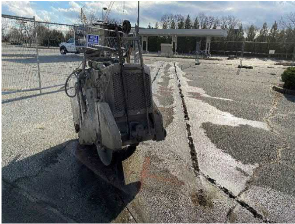
Picture 1: Strategic beginning to saw cut the asphalt.
