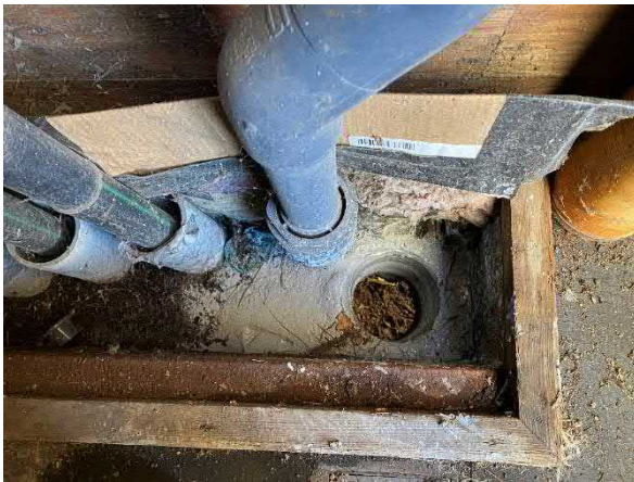
Picture 3: 5" hole in remediation trailer for the new effluent discharge line.
