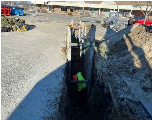
Picture 17: Strategic prepping bottom of trench with pea gravel.
