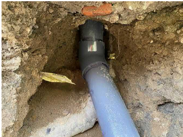
Picture 4: New effluent discharge line connection underneath the concrete slab.
