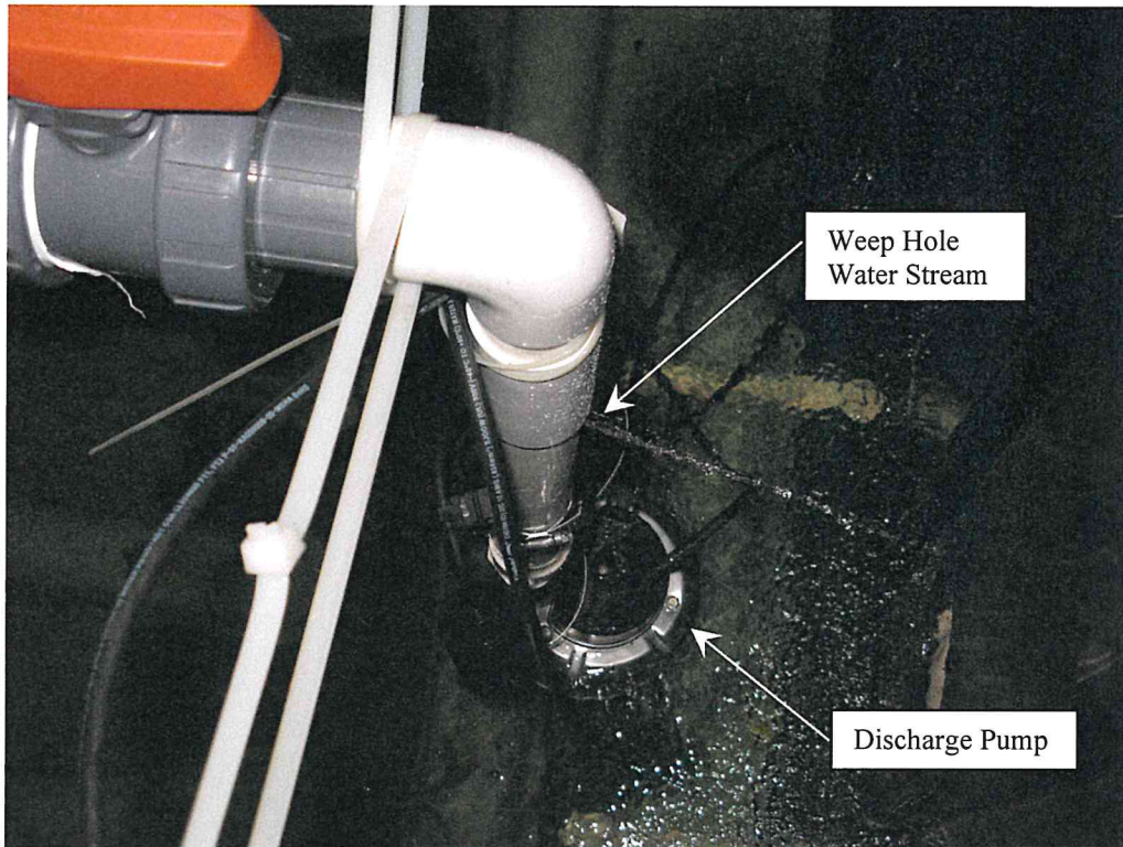
Figure 9: Discharge Pump Assembly
