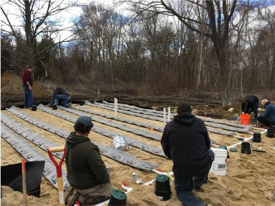
Installing GeoMat above aerobic zone
