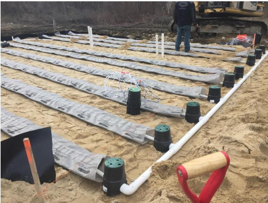
Installing GeoMat above aerobic zone
