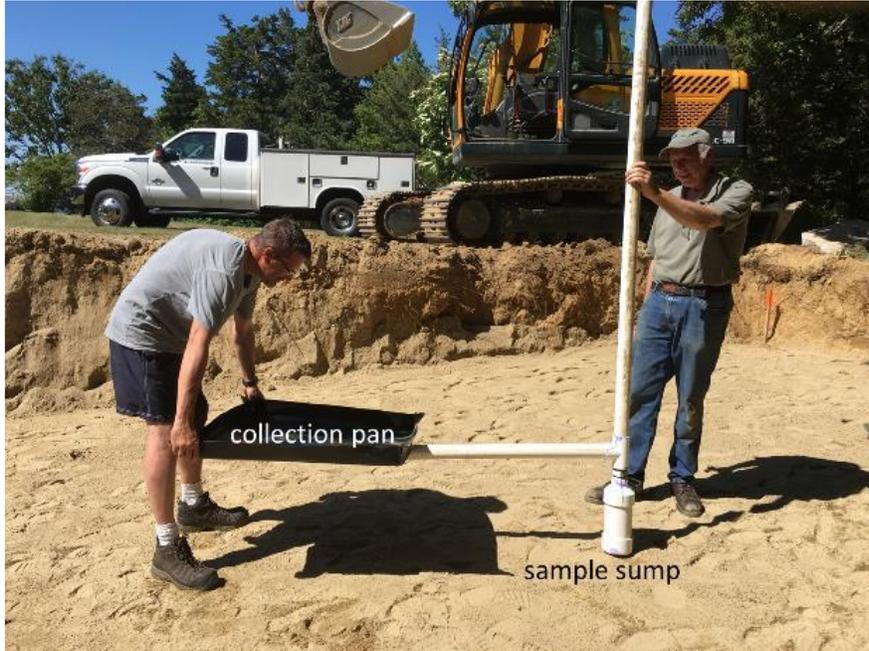
Installing pan lysimeter final effluent sample collection equipment before installation of LSTA
