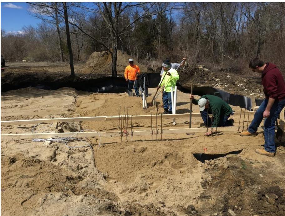
“Walking in” lifts of aerobic zone sand, sampling equipment visible
