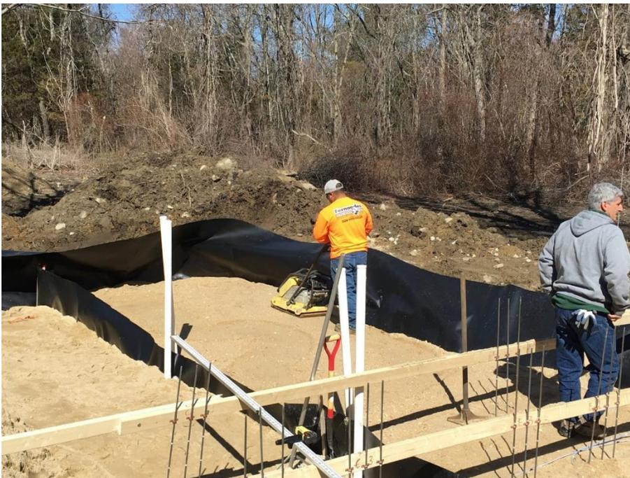
Compacting in first layer of 1:1 mixture, see liner. Note: this demonstration project also used a control STA with sand only as shown on the left of the LSTA
