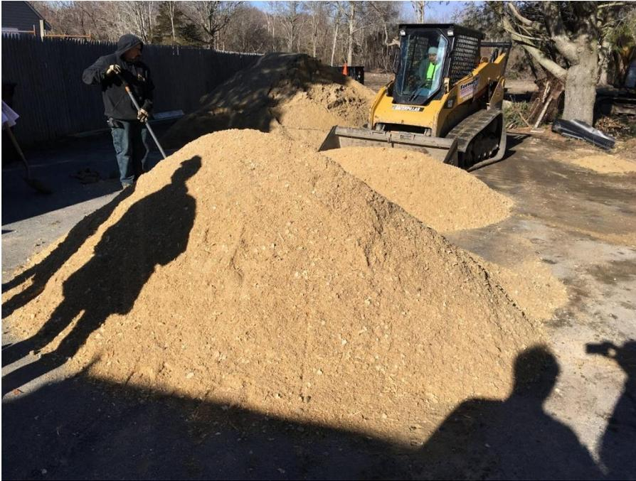
Mixing sand and sawdust 1:1 ration on a clean paved staging area
