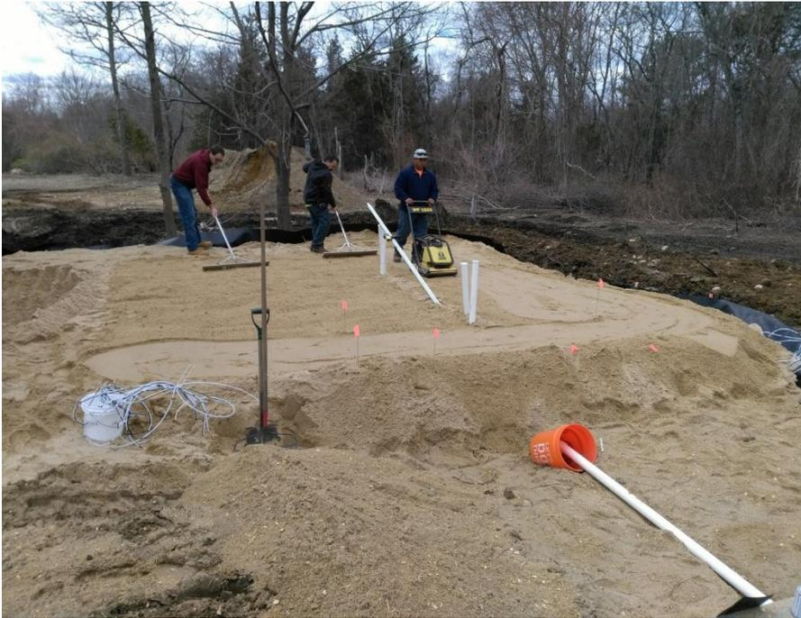
Compacting and finishing the grade of lifts of aerobic zone sand, sampling equipment visible
