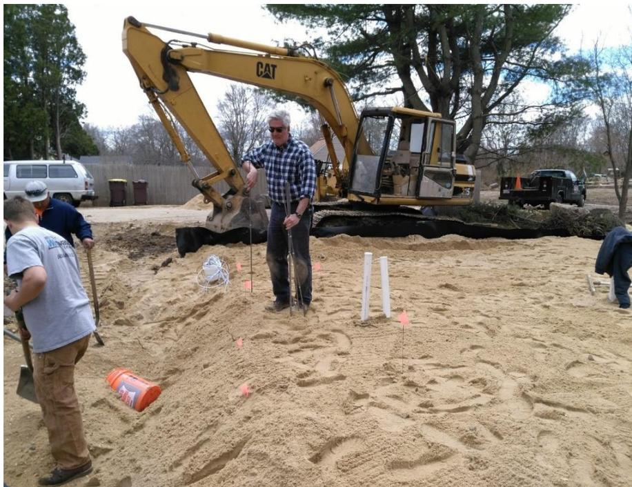
Finishing the grade of lifts of aerobic zone sand, sampling equipment visible
