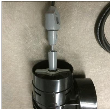
Installing float switch in effluent screen
