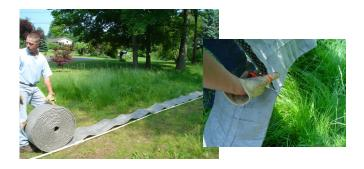
3a. Roll out GeoMat 1200. Cut the GeoMat using shears to desired length.
