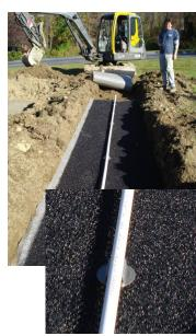
5b. Carefully cover the GeoMat 3900 with the fabric Provided. Fold the top fabric under bottom flaps and staple using an Arrow P22 stapler to keep dirt out of the mat while backfilling the system.
