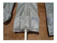
Carefully slide mat along ground and place in the trench. Care should be taken to prevent damage to the solvent weld joints in the distribution pipe when placing the fully assembled GeoMat 1200 in the trench.
