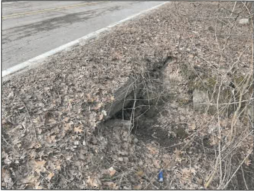
Photo No. 11.: Upstream end of the Central Avenue culvert crossing.
