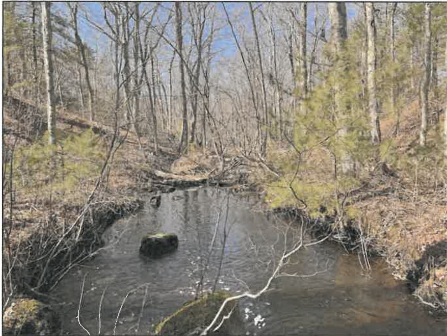
Photo No. 3.: View of the channel through the former dam from 50 feet upstream of former dam centerline looking downstream.
