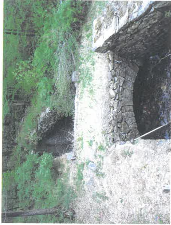
Photo 5. View from top of dam of primary spillway discharge Channel with stone arch bridge.
