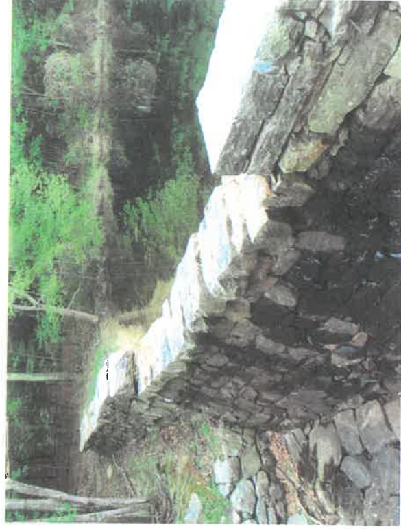
Photo 4. View of emergency spillway on right side of dam.
