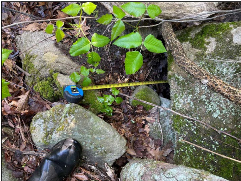
Photo No. 12.: View of one of the many voids within the large boulders that extend as far as 4 feet in the upstream direction.
