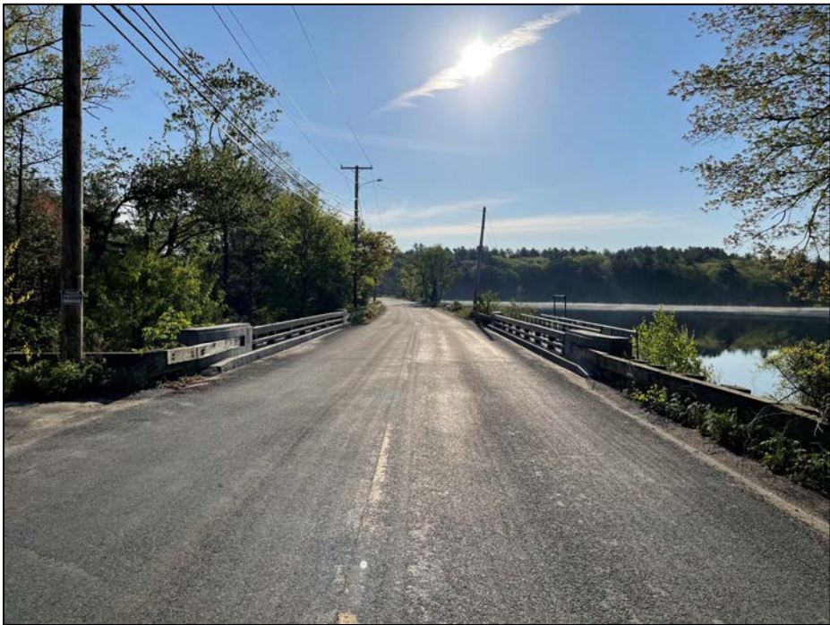
Photo No. 5.: Crest from the left abutment looking right.
