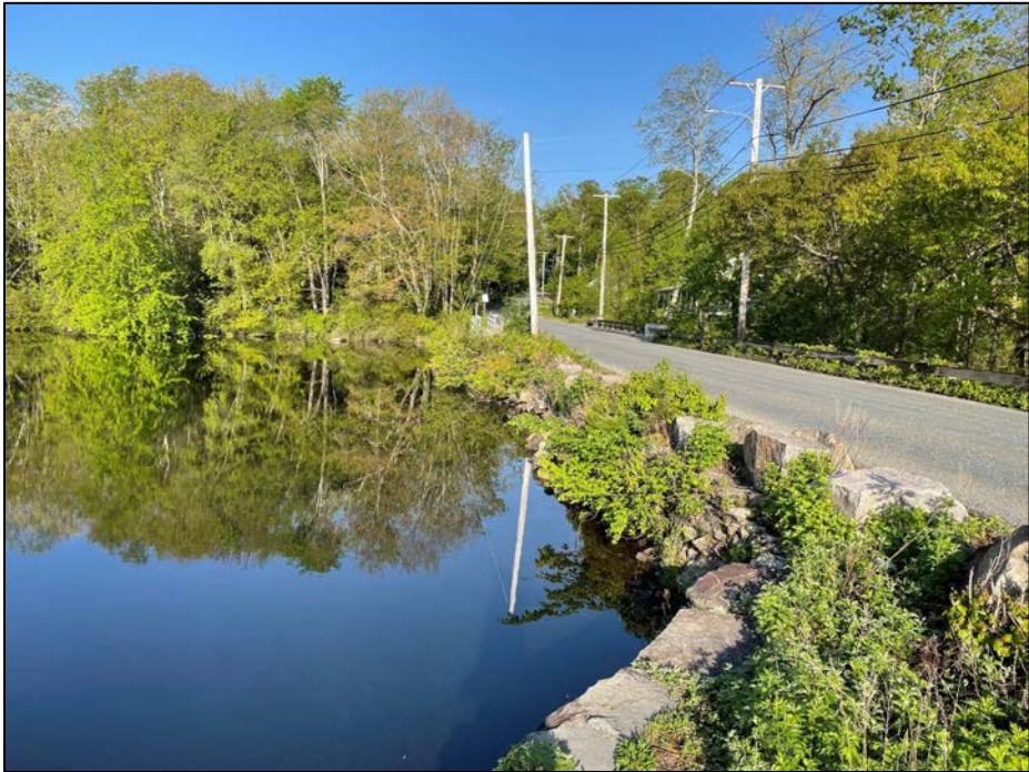
Photo No. 3.: Upstream slope from the LLO intake structure looking left.
