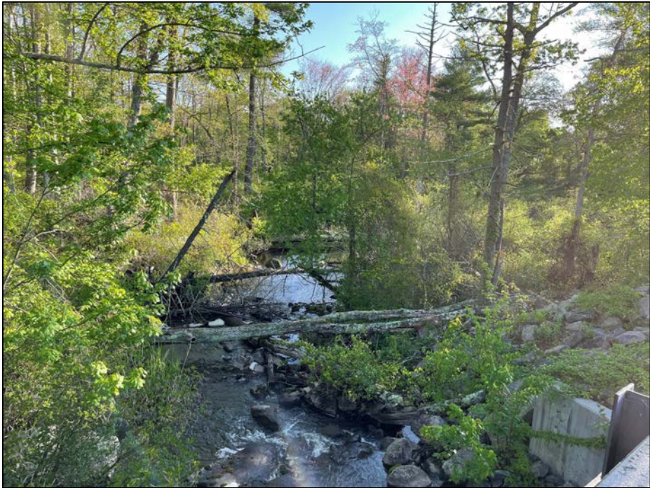
Photo No. 23.: Downstream channel of the spillway.
