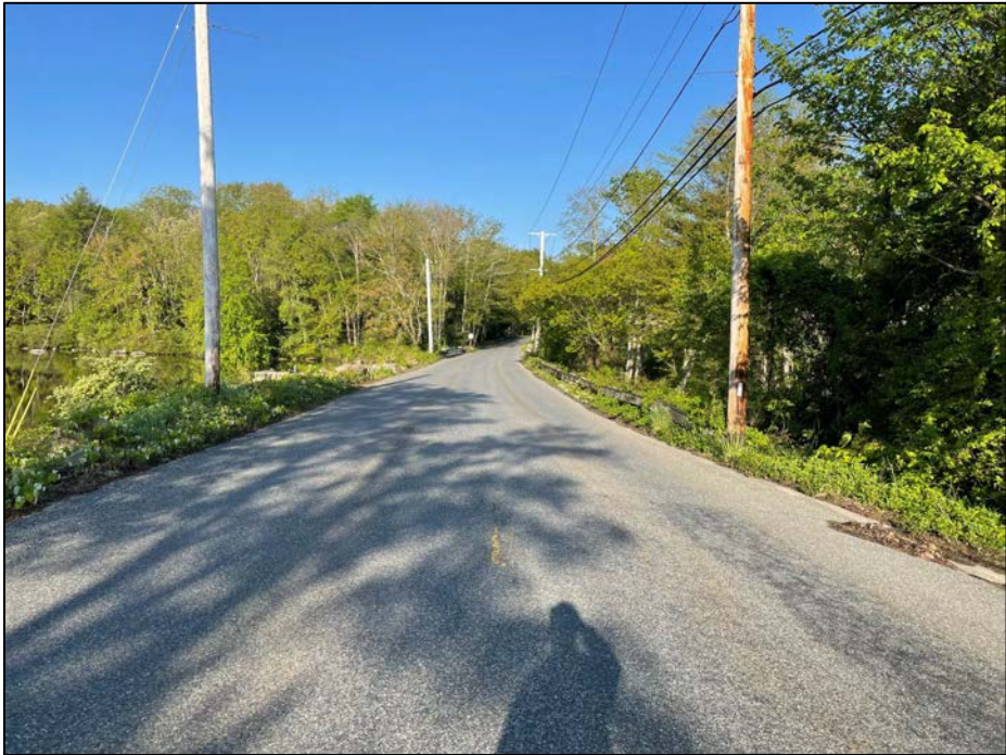
Photo No. 7.: Crest from the right abutment looking left.
