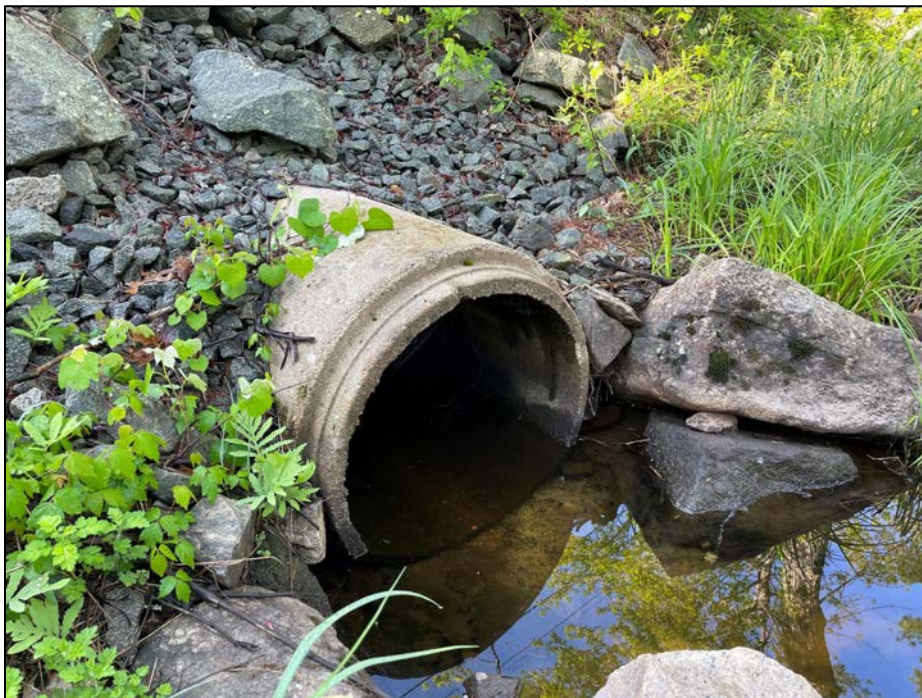
Photo No. 26.: Outlet end of the LLO outlet pipe.
