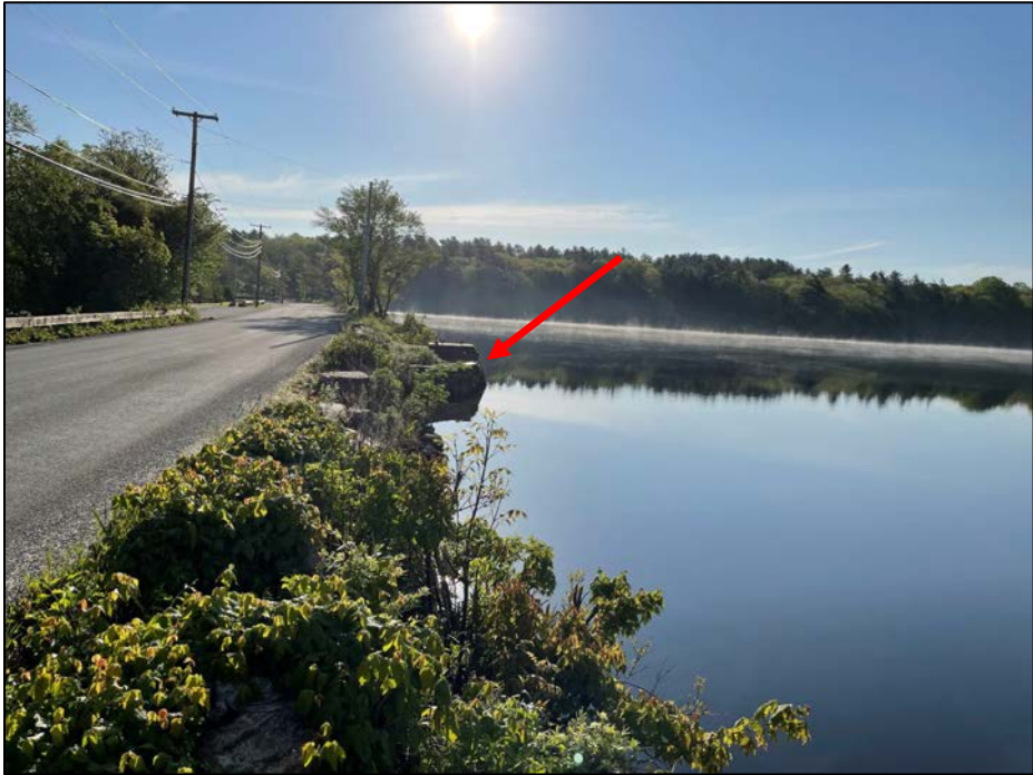
Photo No. 24.: View of the LLO intake structure (red arrow).
