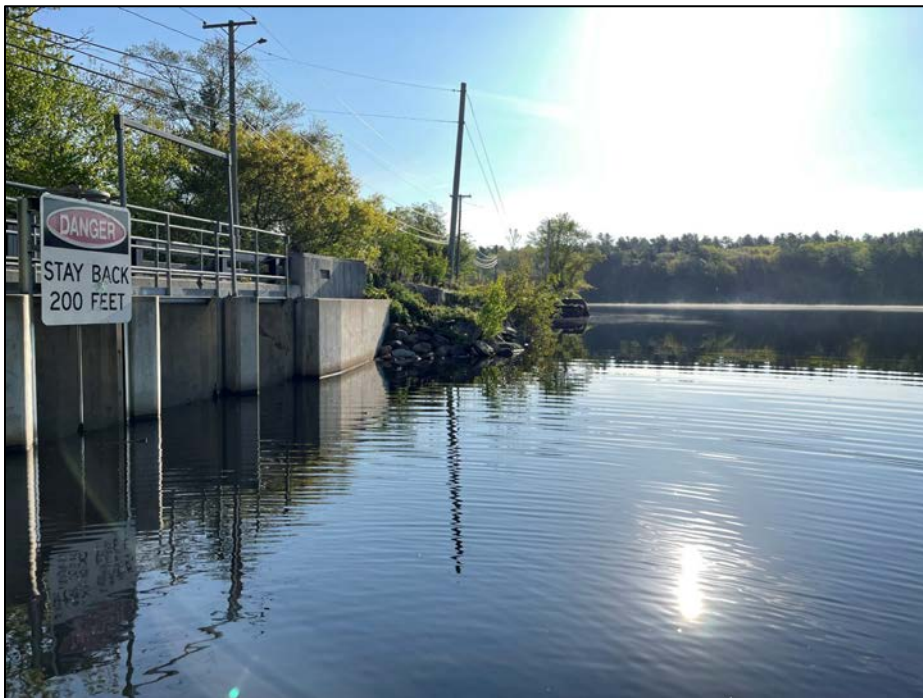
Photo No. 2.: Upstream slope from the left abutment looking right.
