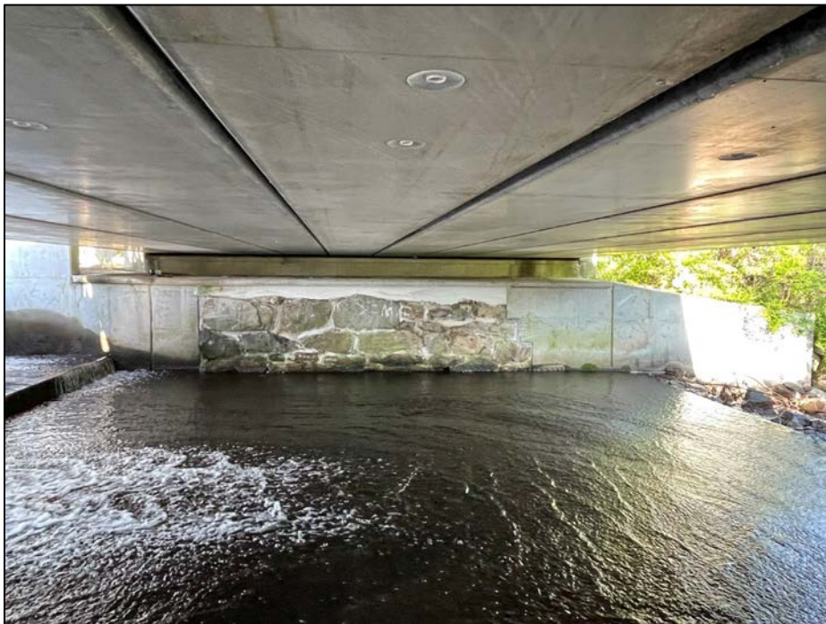
Photo No. 20.: Left training wall of the spillway discharge channel.
