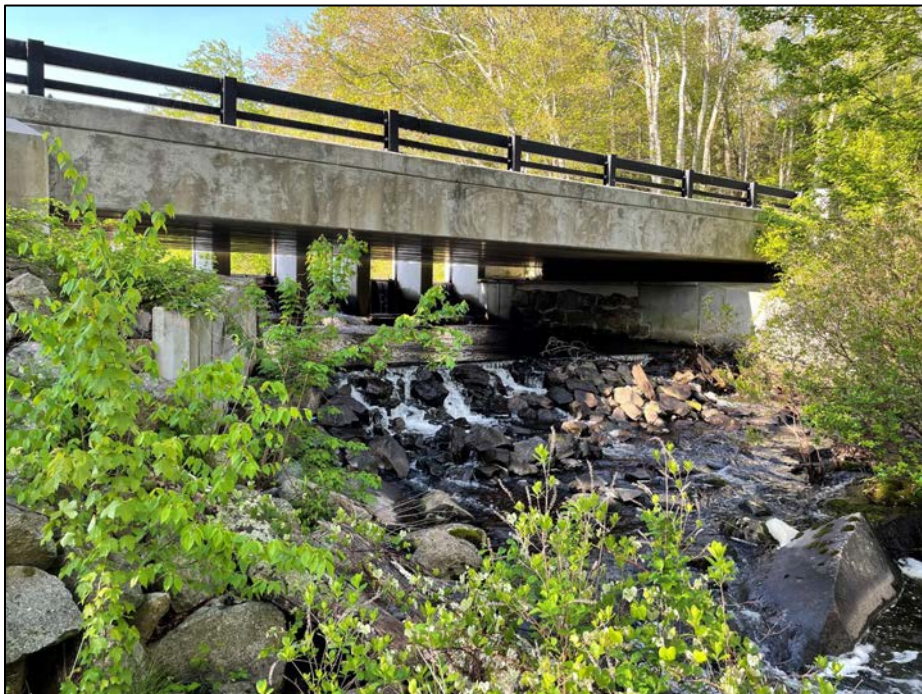
Photo No. 22.: View of the discharge channel of the spillway.
