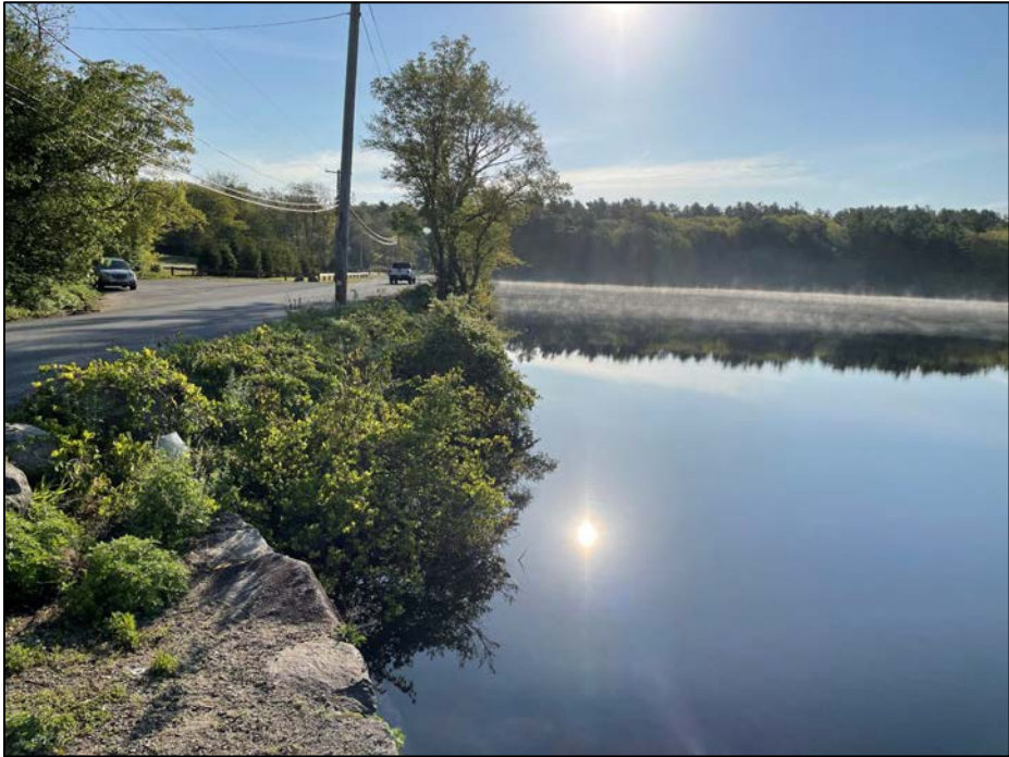
Photo No. 4.: Upstream slope from the LLO intake structure looking right.
