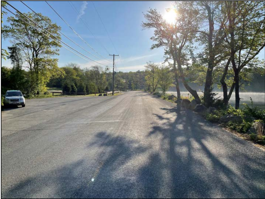
Photo No. 8.: Crest of the right abutment looking right.
