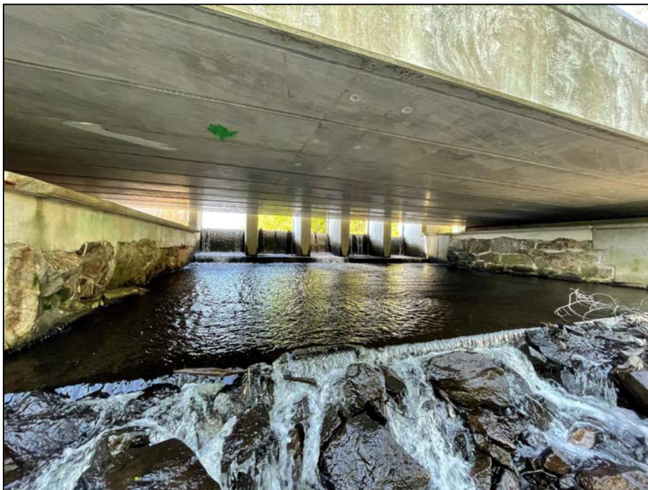
Photo No. 18.: Discharge area of the spillway looking upstream.
