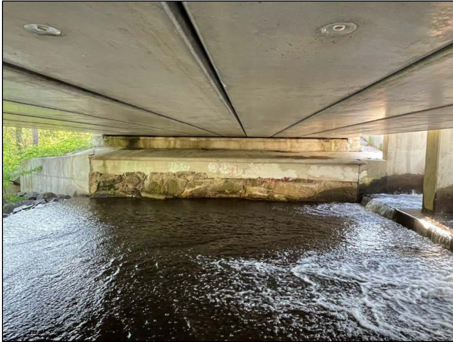
Photo No. 21.: Right training wall of the spillway discharge channel.
