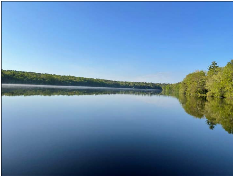
Photo No. 1.: Overview of the impoundment from the low level outlet (LLO) intake structure looking upstream.
