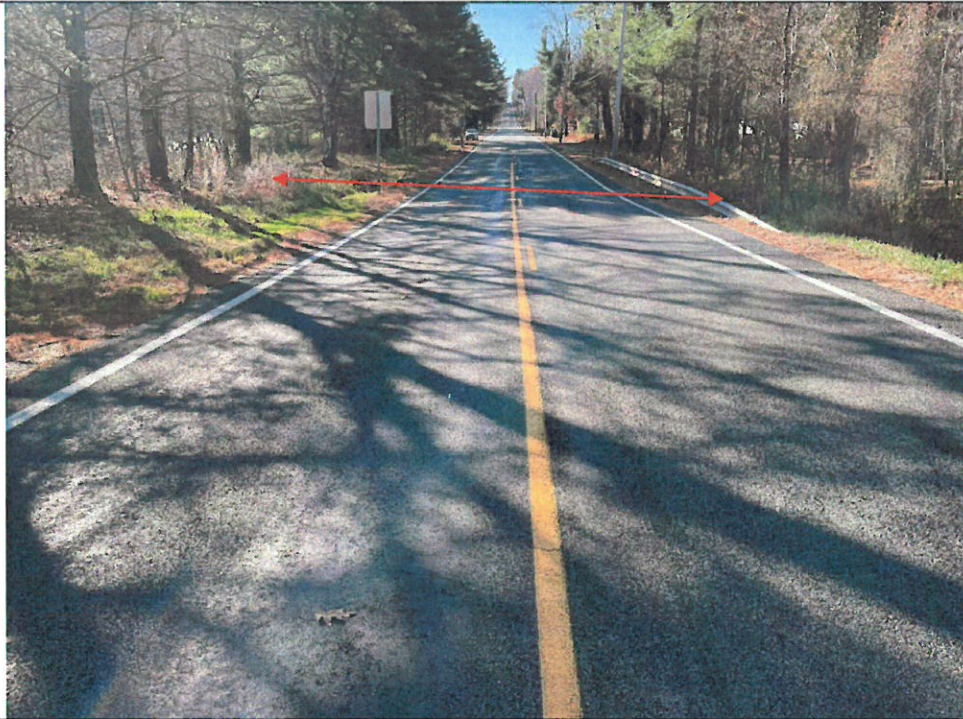
Photo 7: View of the crest and embankment from the right abutment looking left. Note the location of the primary spillway culvert (red).
