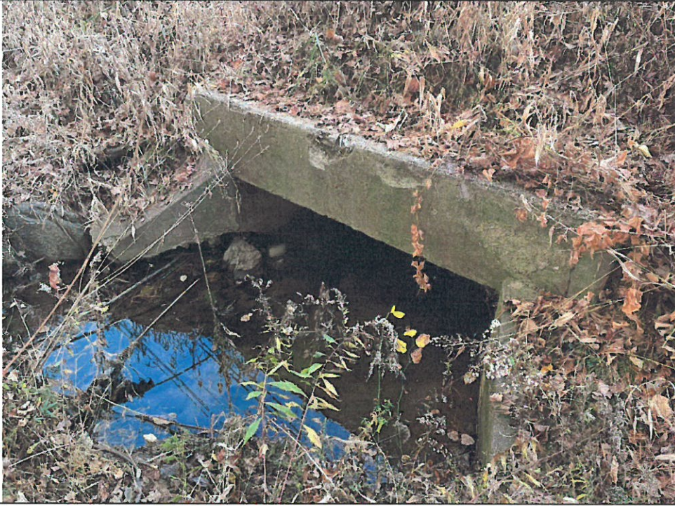
Photo 15: View of the primary spillway discharge outlet and wingwalls. Note the encroaching vegetation that would reduce spillway discharge capacity.
