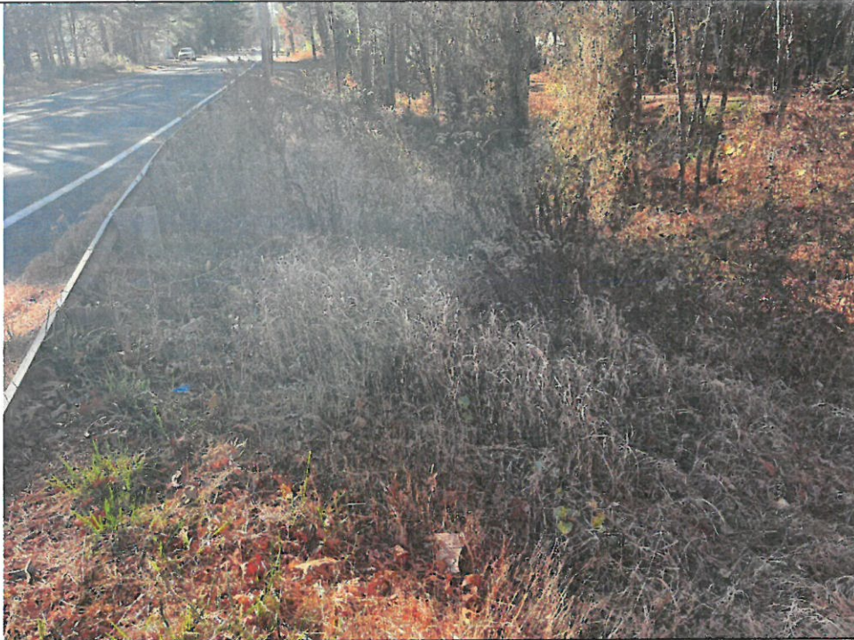
Photo 9: View of the downstream embankment from the right abutment looking downstream and left. Note the dense vegetation.
