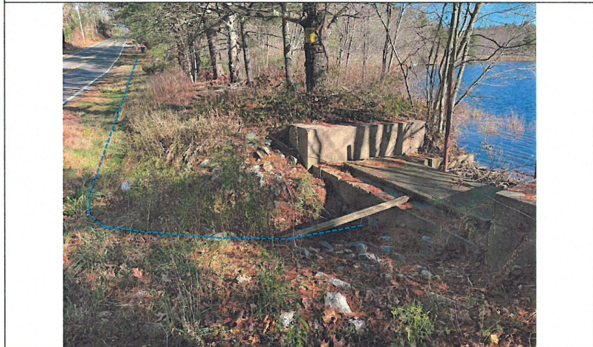
Photo 4: View of the dam crest and embankment from the primary spillway looking right. Note the drainage swale slopes into the back of the primary spillway (blue).
