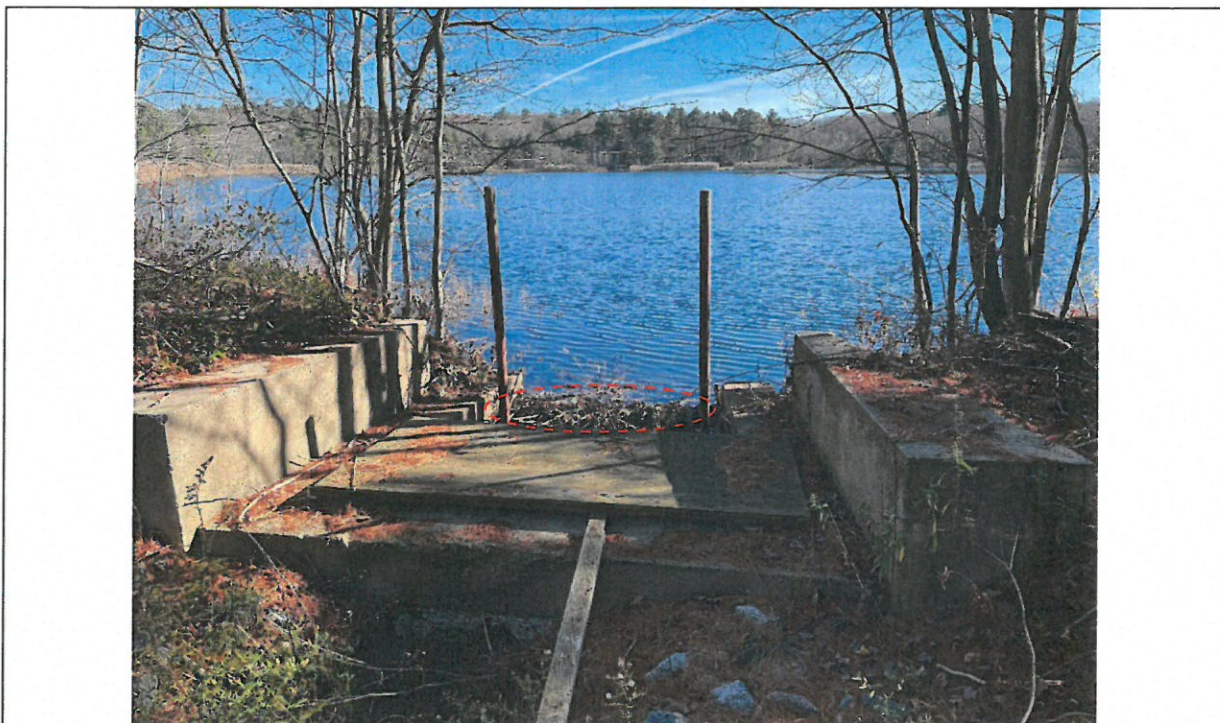
Photo 1: View of the impoundment from the primary spillway. Note the sticks/debris accumulating on the weir (circled in red).
