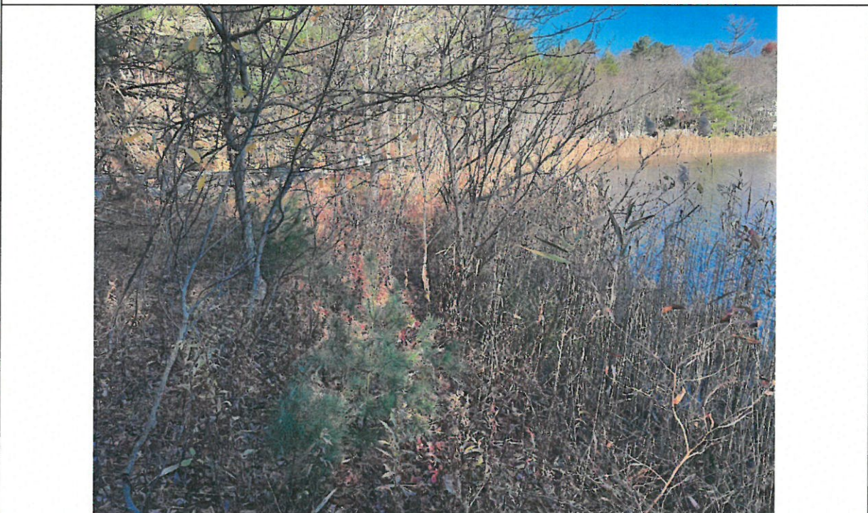
Photo 2: Upstream embankment as viewed from the left abutment looking right. Note the leaf litter and developing vegetation.
