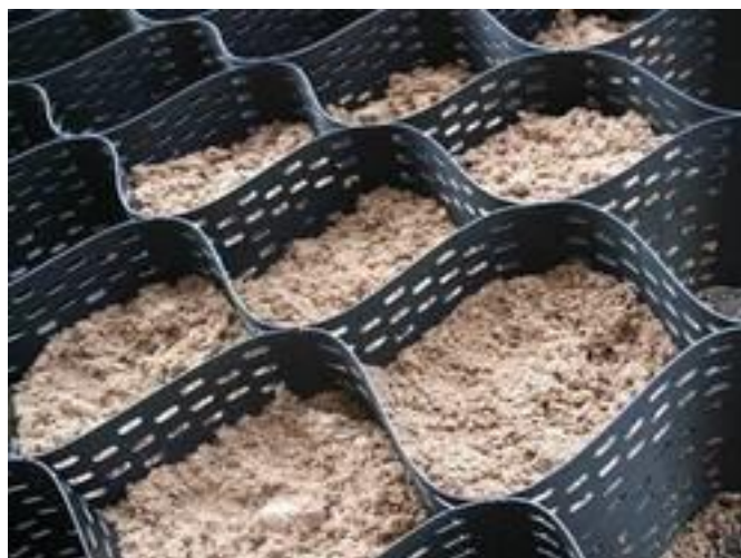
Figure 2. Typical Cellular Confinement System
