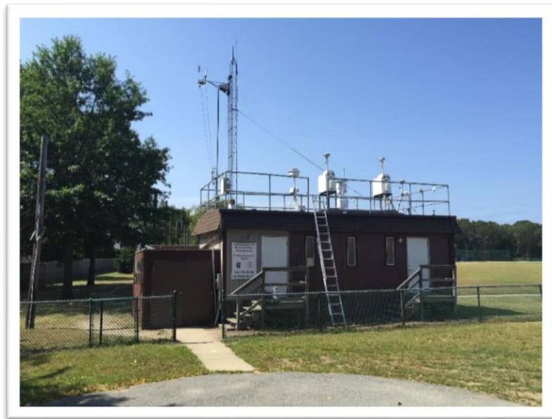
View of East Providence Trailer Facing West
