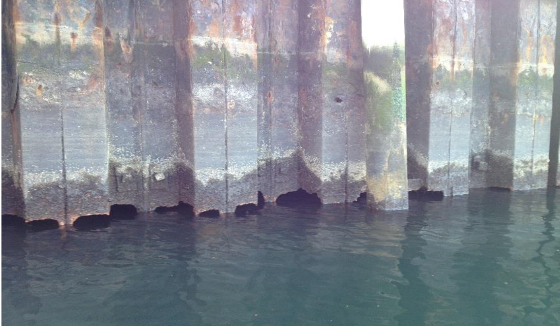
Photo 5: Existing steel sheet pile wall
