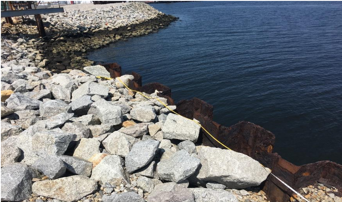
Photo 6: Existing steel sheet pile wall and riprap slope
