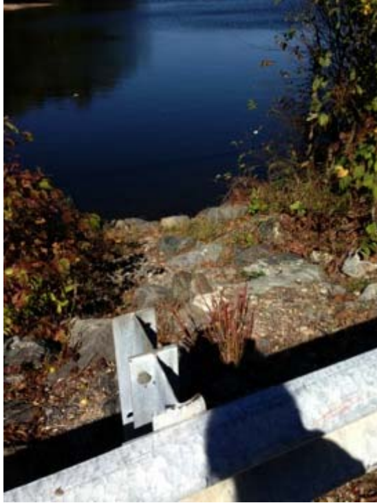
Photo 5: Overview of rip rap on upstream slope
