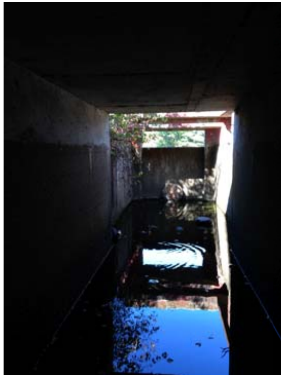
Photo 16: Primary spillway culvert
