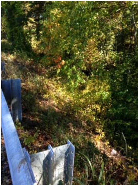
Photo 12: Overview of downstream slope
