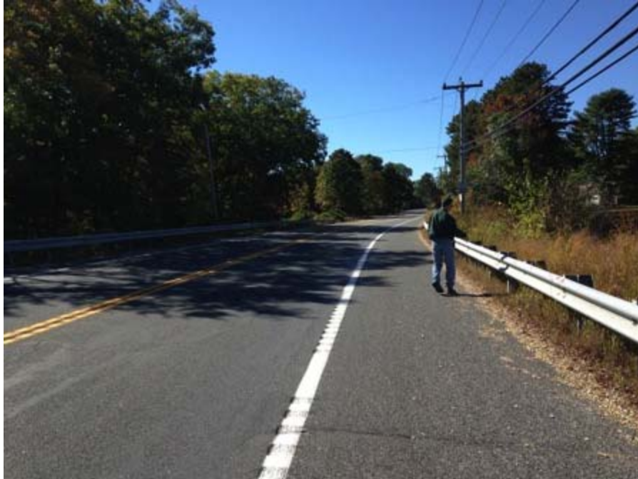
Photo 3: Overview of dam crest from left abutment looking right
