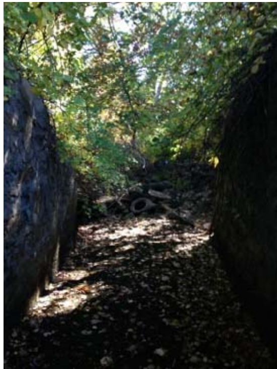
Photo 18: Primary spillway downstream channel
