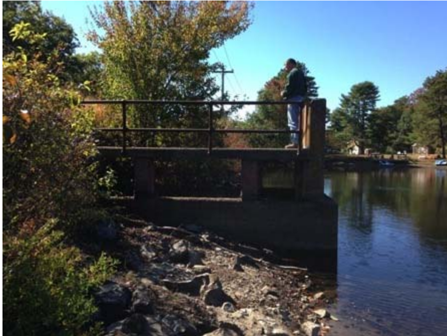
Photo 7: Overview of spillway weir
