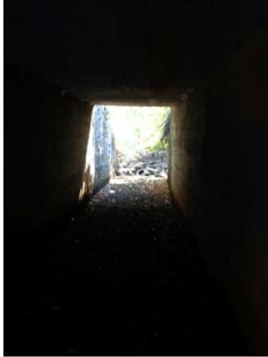
Photo 17: Primary spillway culvert
