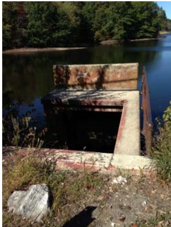
Photo 8: Overview of spillway weir
