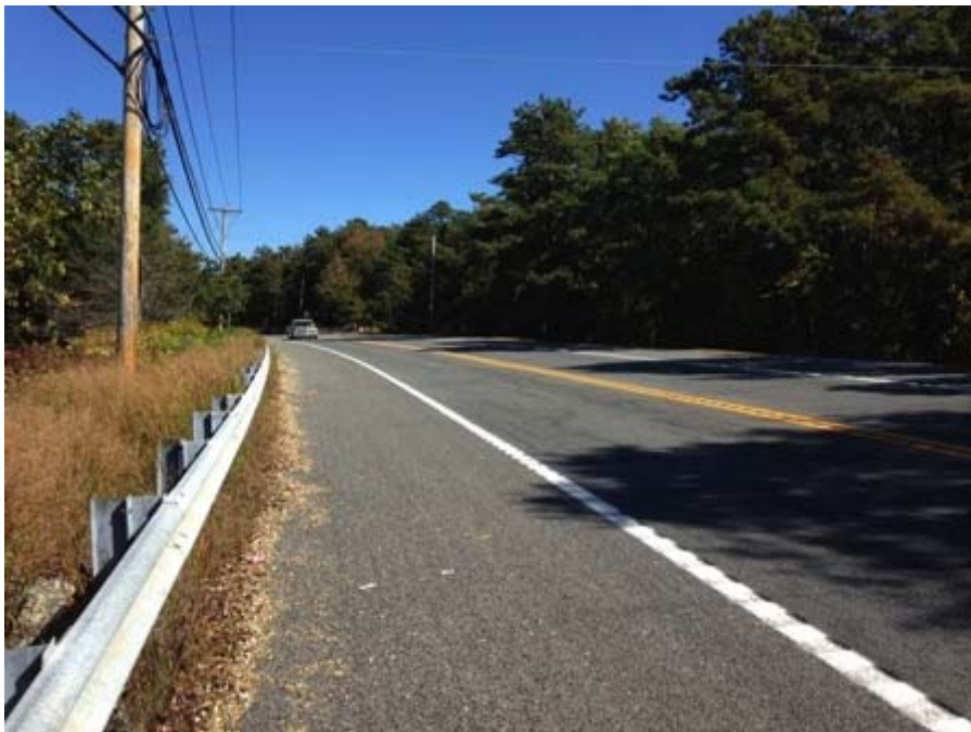
Photo 2: Overview of dam crest from right abutment looking left
