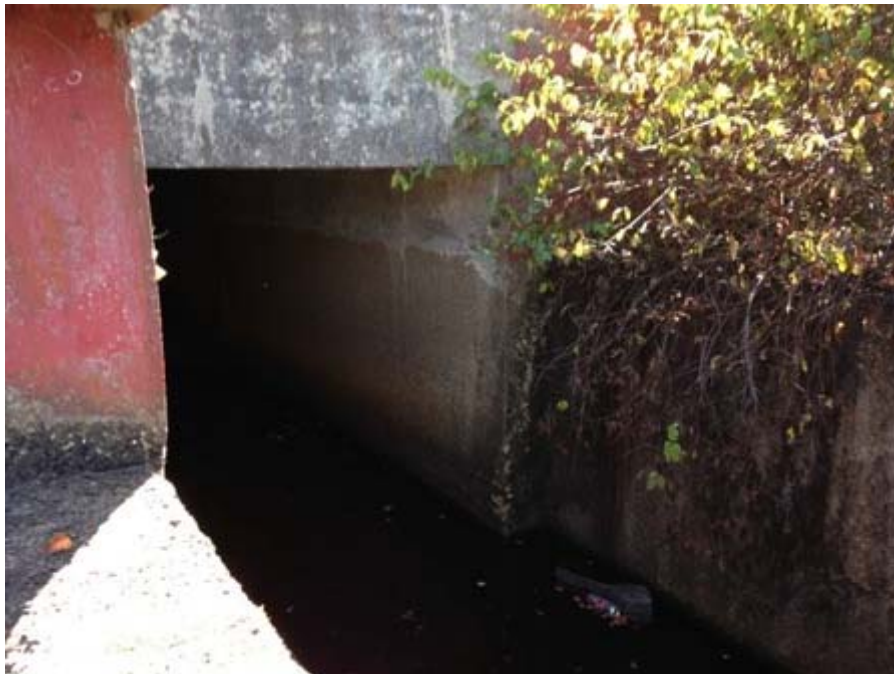
Photo 10: Spillway concrete culvert
