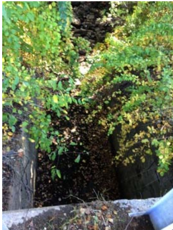
Photo 14: Overview of downstream spillway canal
