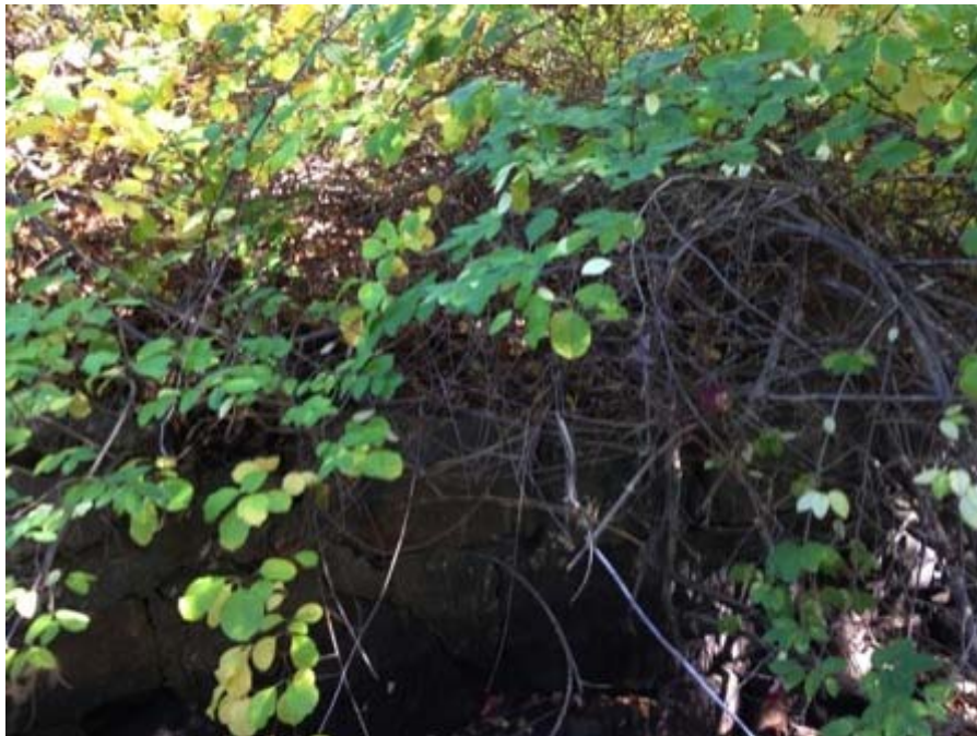
Photo 20: Downstream training walls
