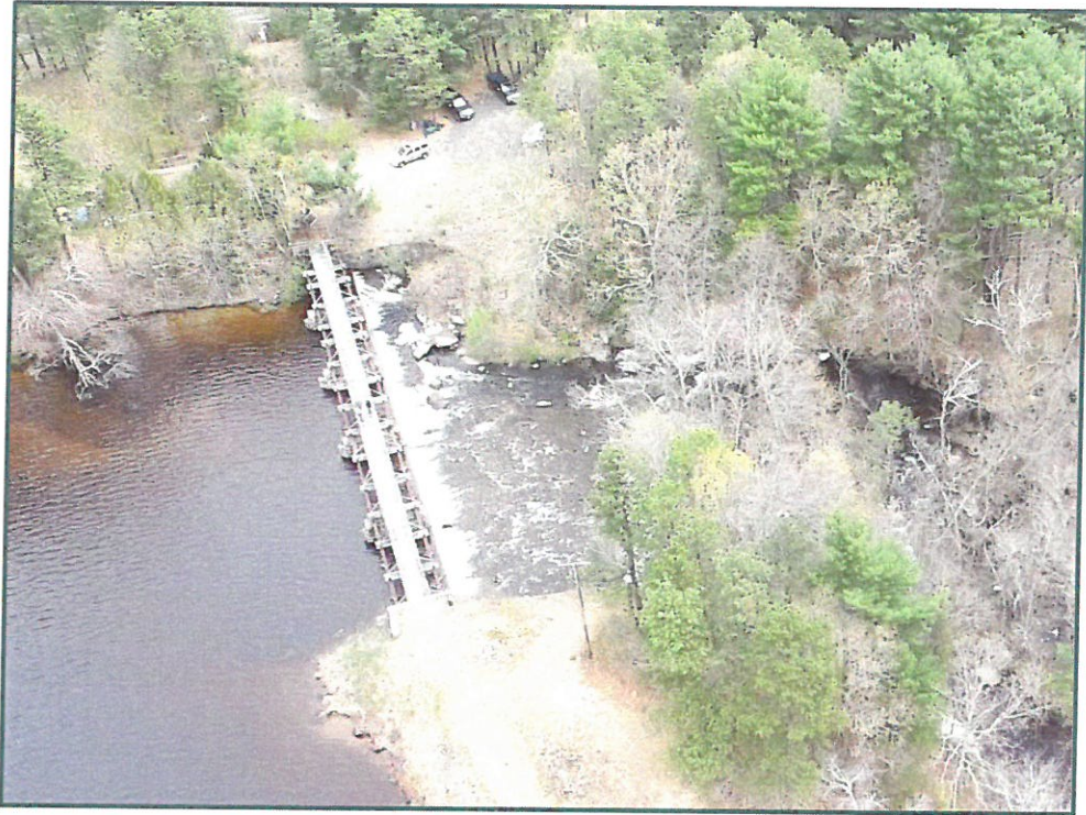
Photo No. 1: Spillway, looking northeast, photo taken on May 11, 2020.
