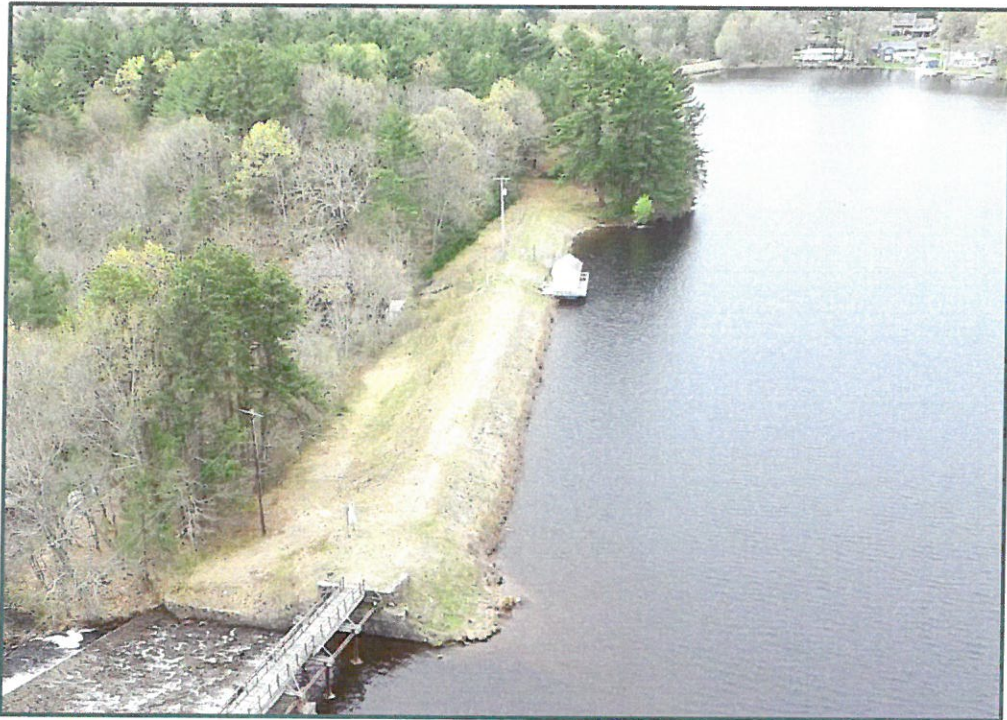
Photo No. 11: North embankment, looking south, photo taken on May 11, 2020.
