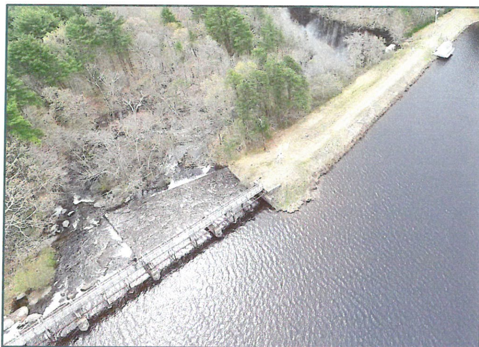
Photo No. 9: Downstream channel, looking southeast, photo taken on May 11, 2020.
