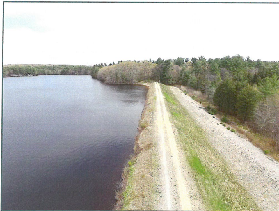
Photo No. 20: South embankment, looking northeast, photo taken on May 11, 2020.
