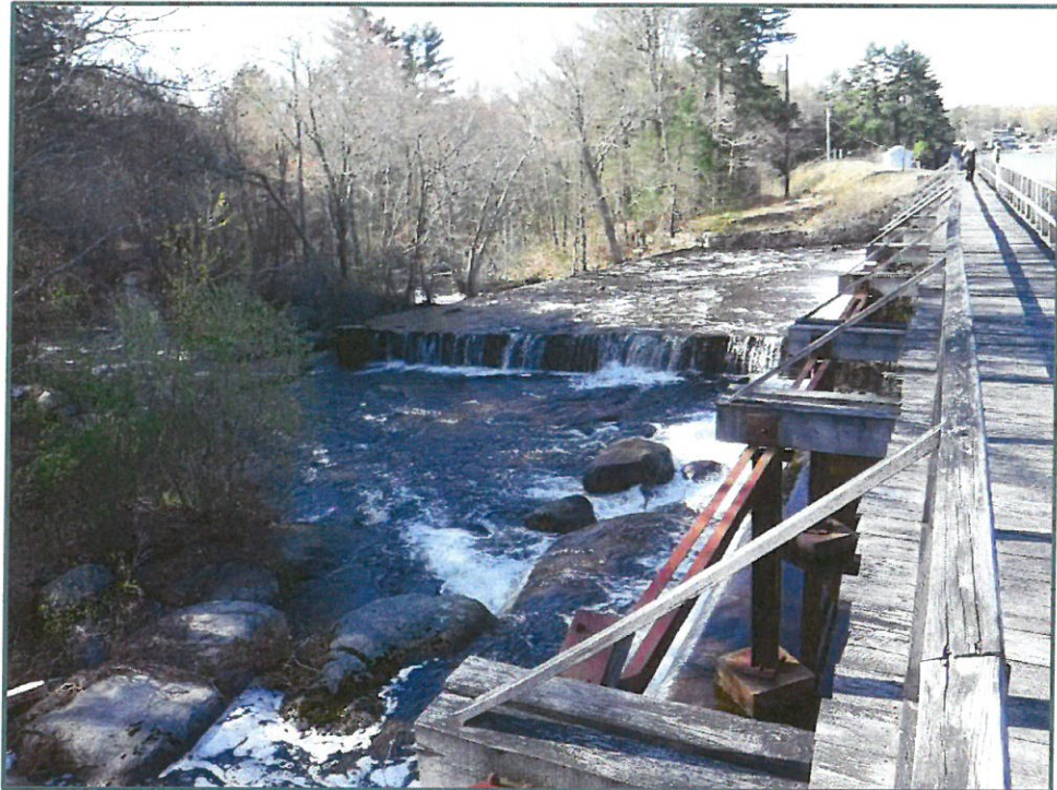
Photo No. 7: Overgrown vegetation along the left side of the downstream spillway area, looking south, photo taken on May 11, 2020.
