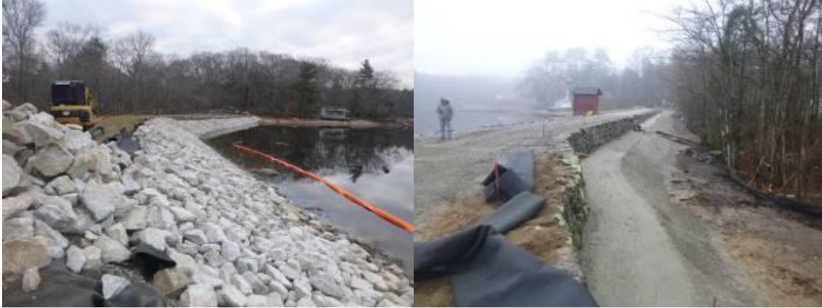
Embankment repair at Quidnick Reservoir Dam (No. 175) in Coventry
