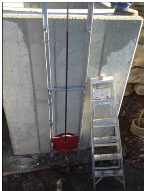
Repaired low level outlet at Slocum Dam (No. 239) in Exeter
