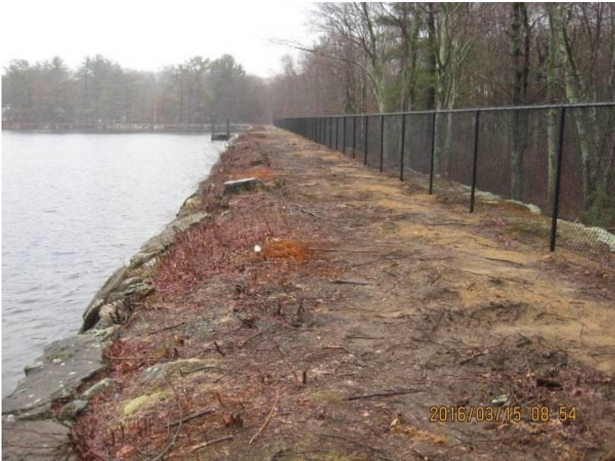
Oak Swamp Dam (No. 168) in Johnston, repaired in 2015
