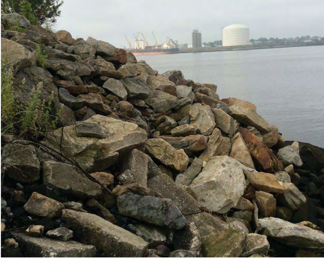
Photo 14: South face (looking south).
