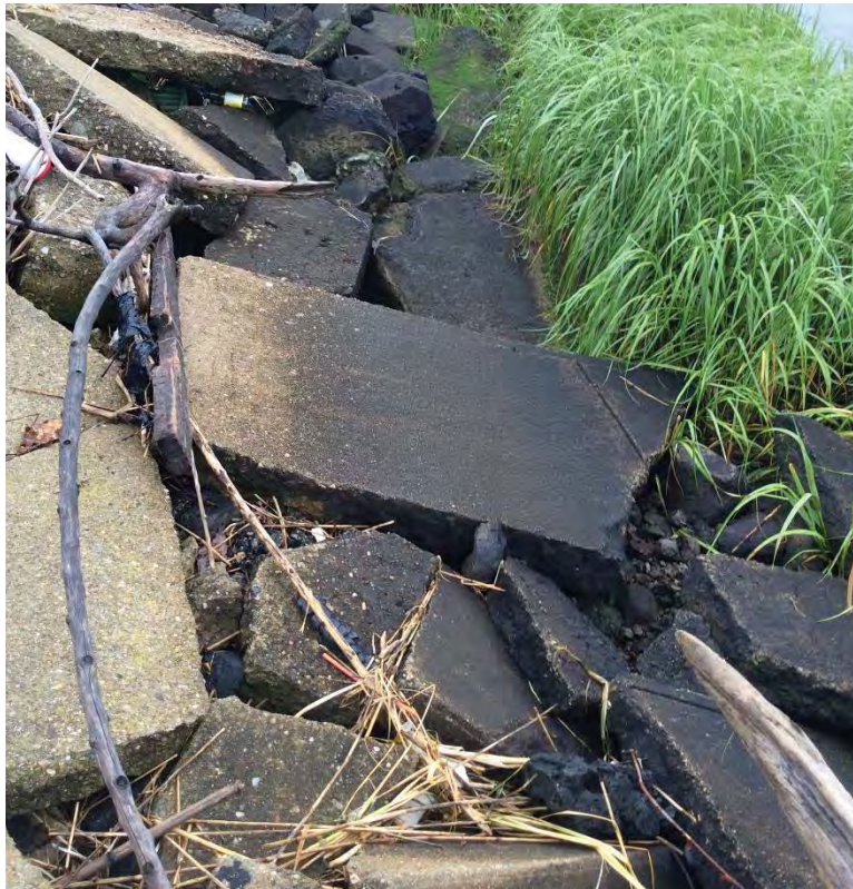
Photo 4: East face, beginning of concrete slabs (looking southeast).
