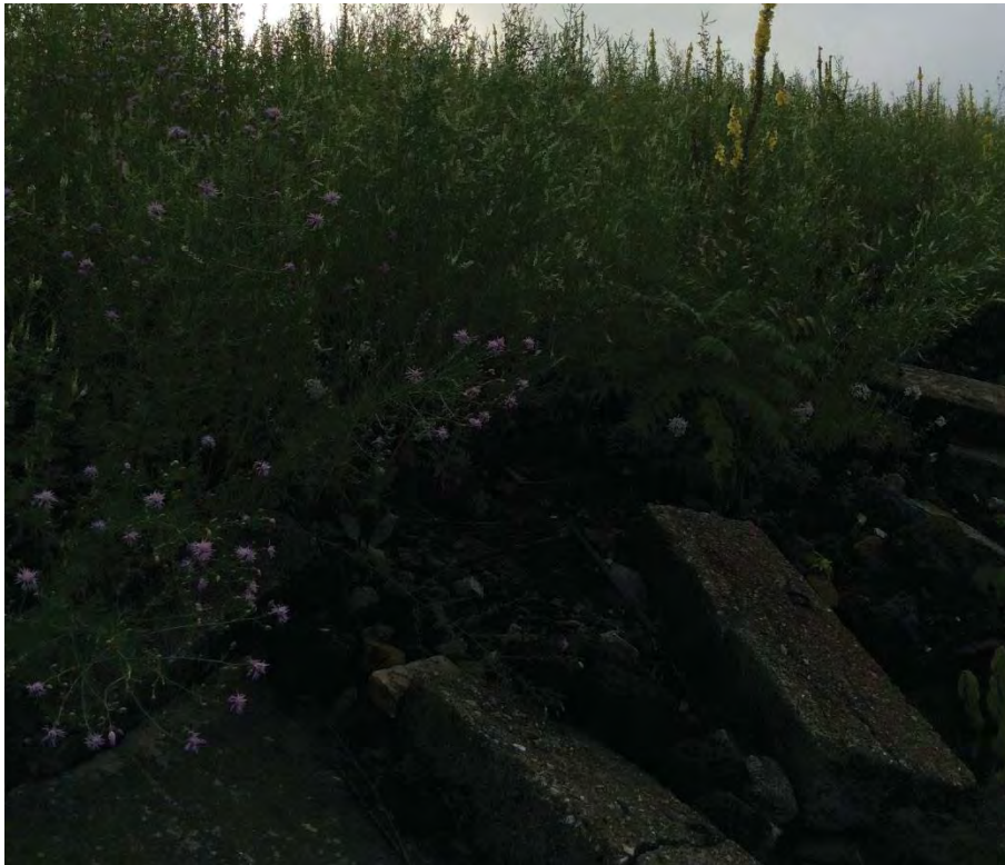
Photo 9B: East face (looking east-southeast).
