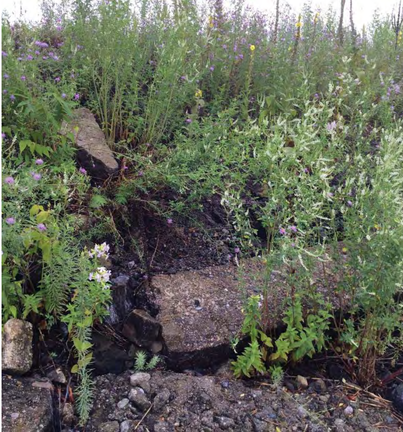
Photo 7A: East face (looking east).
