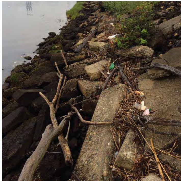
Photo 6B: East face (looking northwest).
