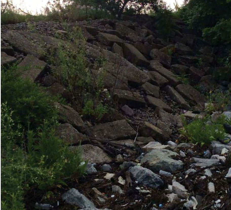
Photo 13A: Swale (looking east-southeast).
