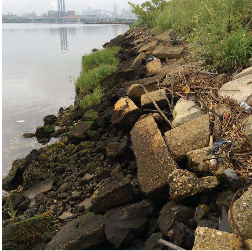
Photo 8: East face (looking northwest).
