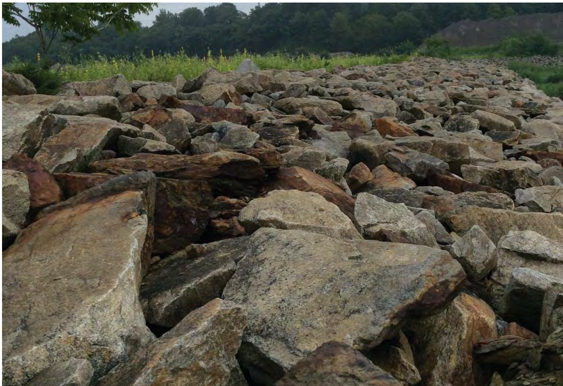
Photo 15: South face (looking east).
