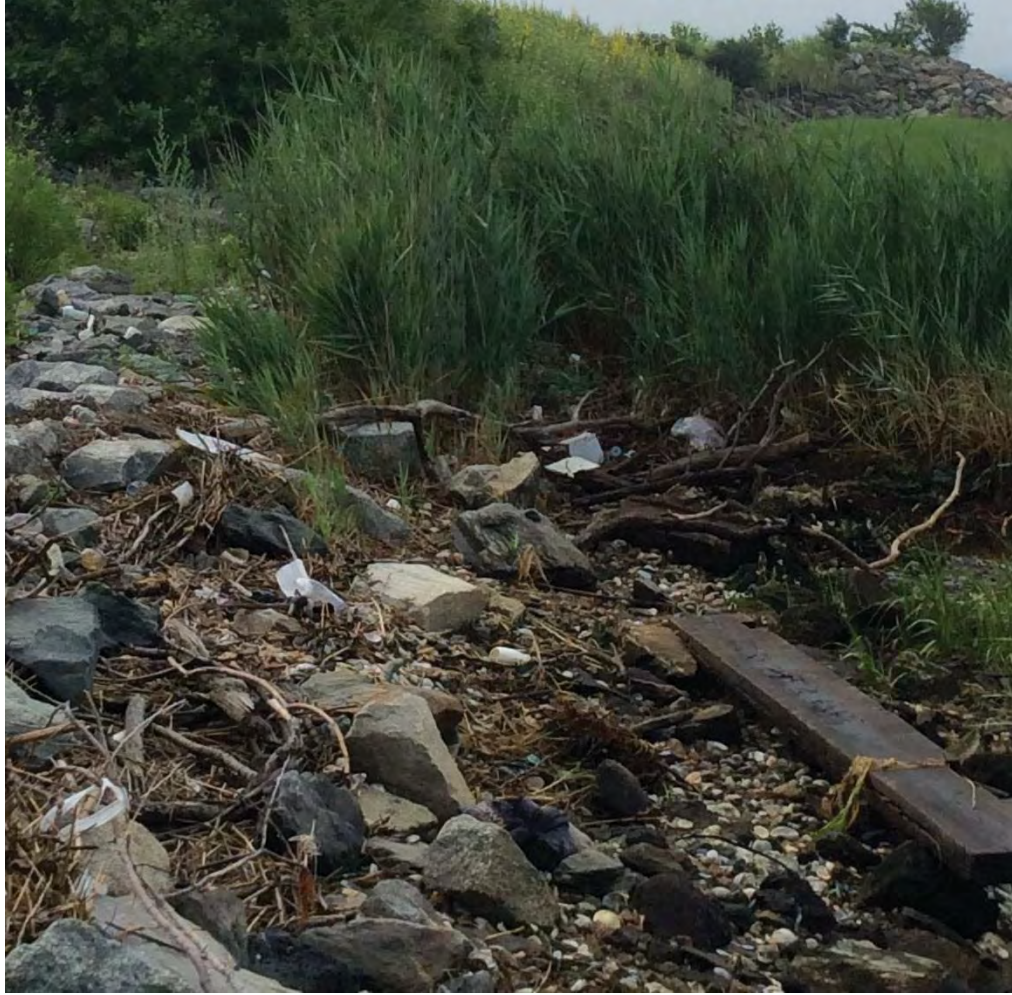
Photo 12: Swale (looking southeast).
