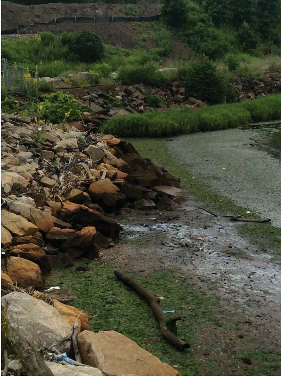
Photo 16: South face (looking east).
