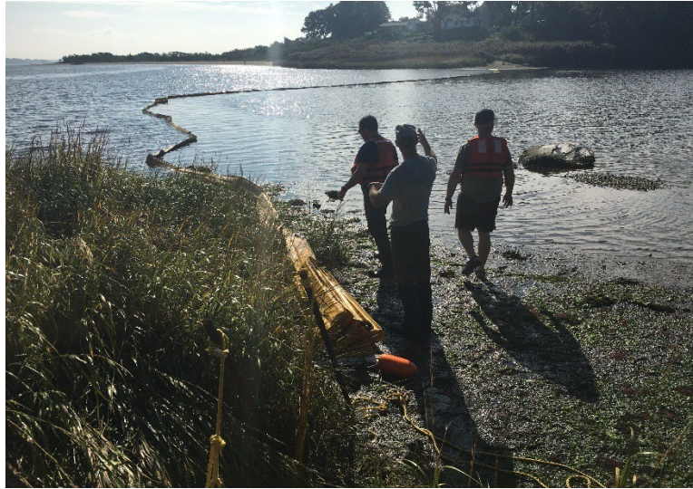
Image 6.7 - OER staff successfully deployed the curtain boom to block the inlet
