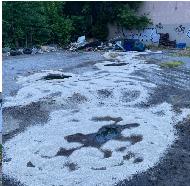
Image 6.3 - pools of waste oil gathered on the asphalt parking lot
