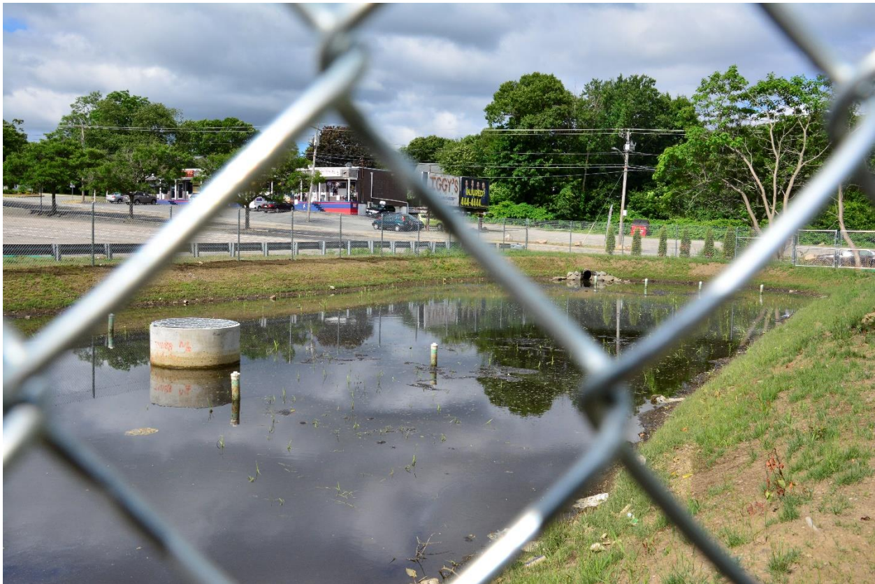
New stormwater BMP off of Warwick Avenue
