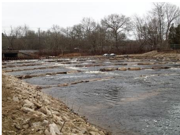
Bradford Dam finished. Photo courtesy of V. Masson.
