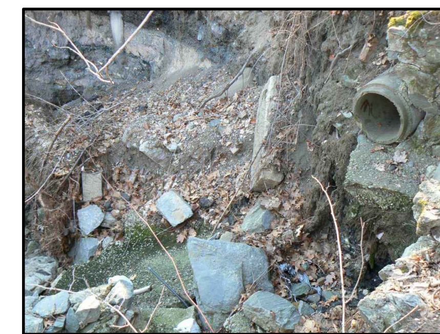
VIEW #3 EXISTING HEADWALL FROM TOP OF WASHOUT (PHOTO TAKEN FEB. 8, 2007)
