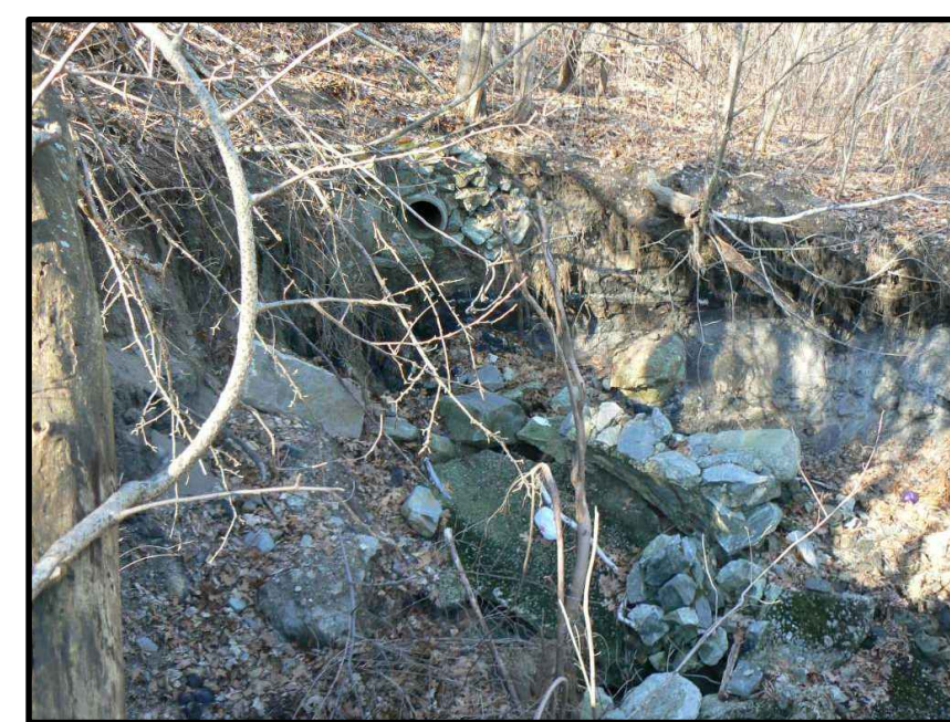
VIEW #2 EXISTING HEADWALL & WASHOUT (PHOTO TAKEN FEB. 8, 2007)
