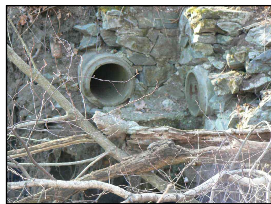
VIEW #1 EXISTING HEADWALL (PHOTO TAKEN FEB. 8, 2007)
