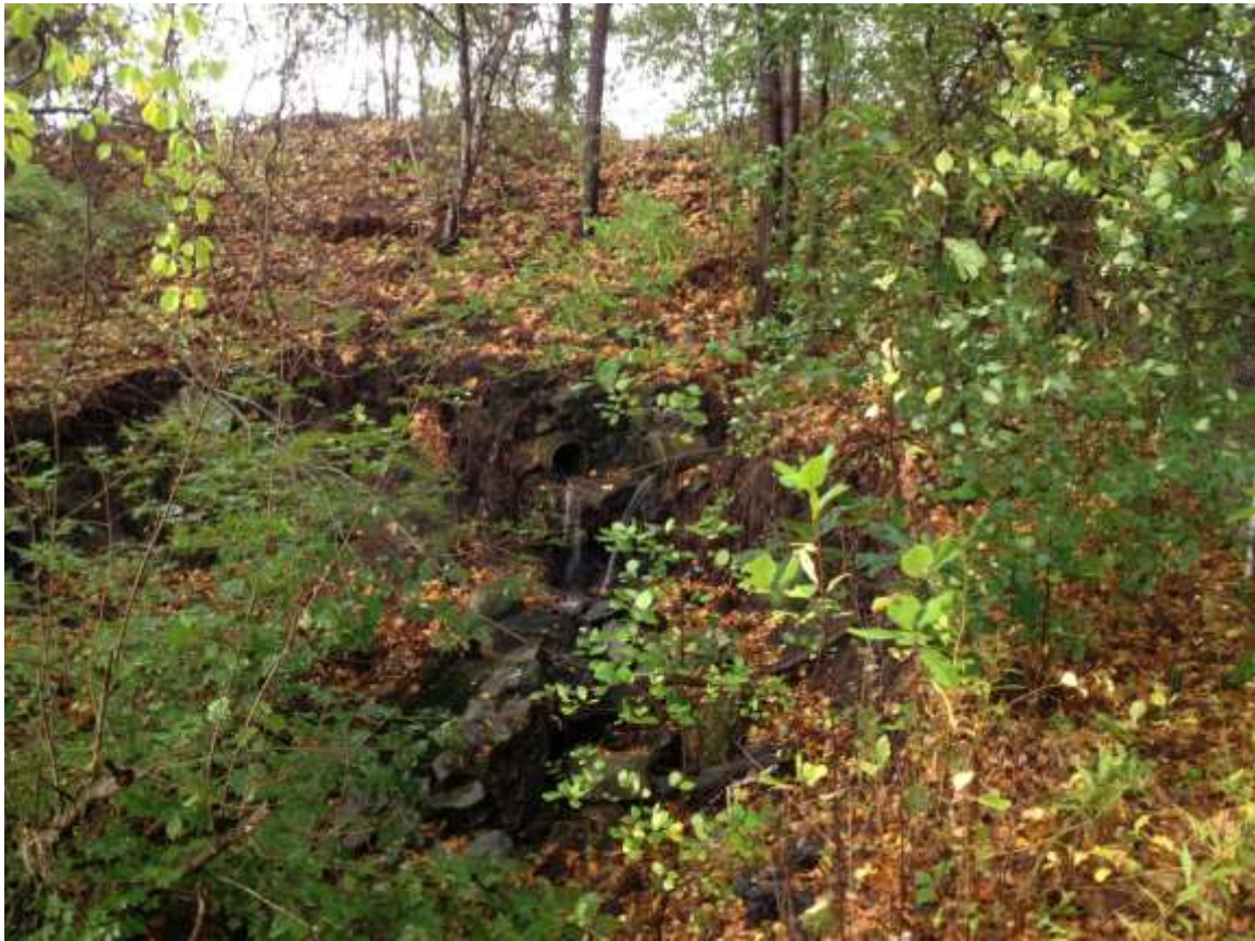
10/24/14 – View of Outfall Pipes.
