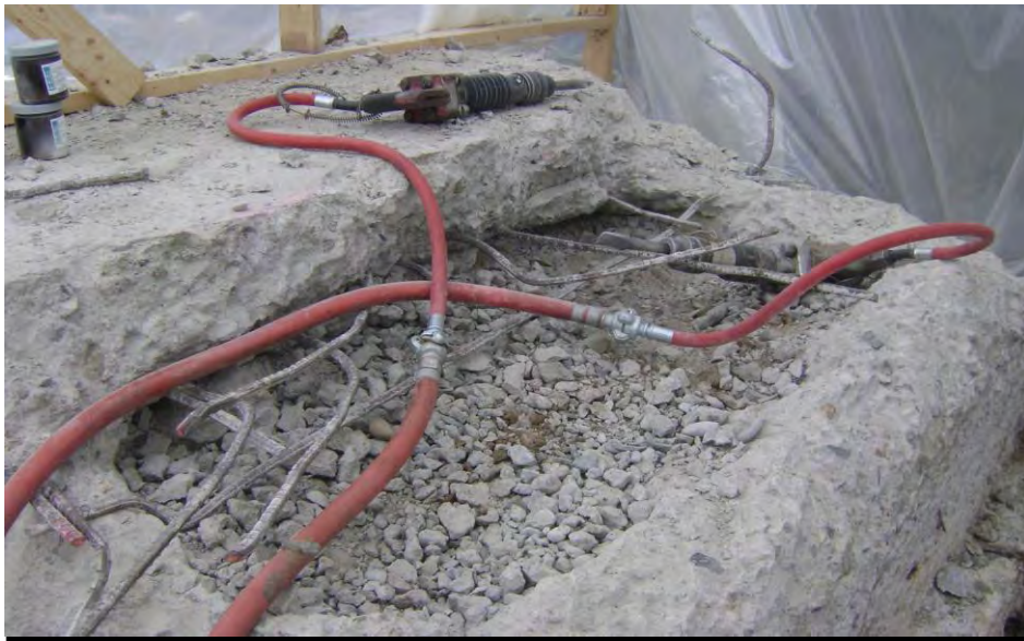
Scarified and/or removed concrete slab. August 25, 2011.
