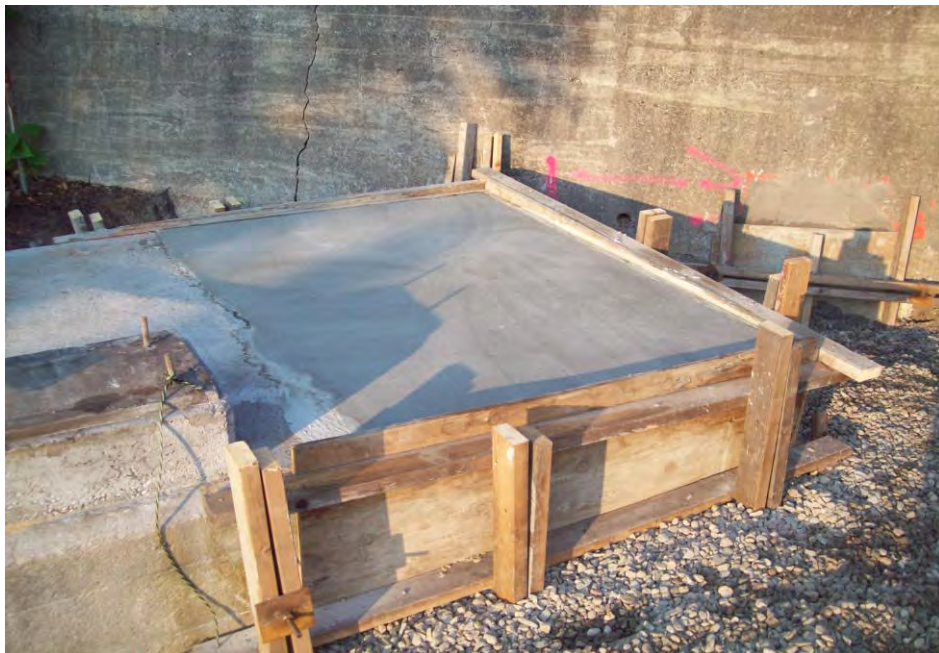
Reconstructed concrete pad. September 14, 2011.
