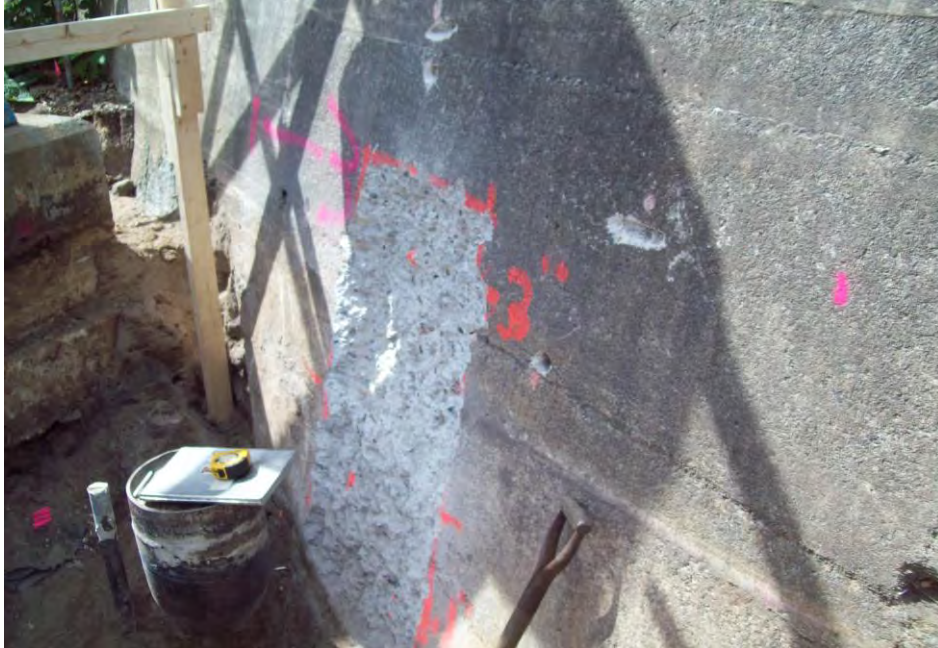
Scarified retaining wall. August 23, 2011.
