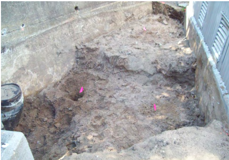
PCB impacted soil excavation and select sampling locations. August 22, 2011.
