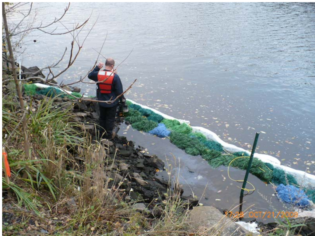
Photo 2: Containment Boom and Oil Snares Installed at Sheen Area
