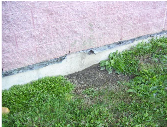
Repaired cavity adjacent to middle school foundation
