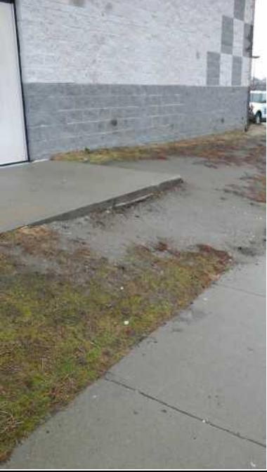
A photograph of a sidewalk and a grassy area. On the sidewalk, there is a distinct depression or erosion area where the ground has been washed away, creating a hole. The background shows a brick wall of a building. |              |
