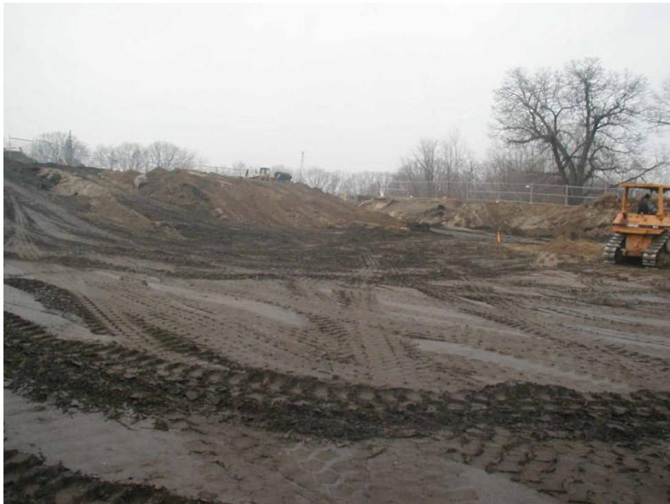
Photo 16. View west during backfilling.
