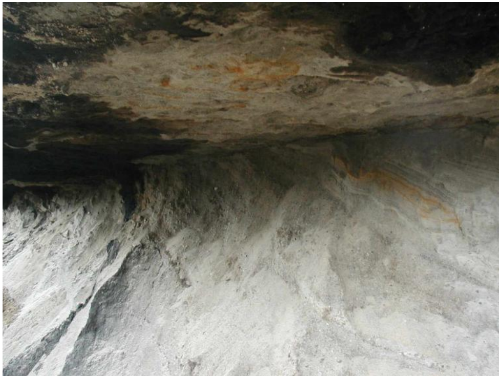
Photo 10. Clean soils directly beneath bunker. Note staining of underside of bunker floor is not continuous.
