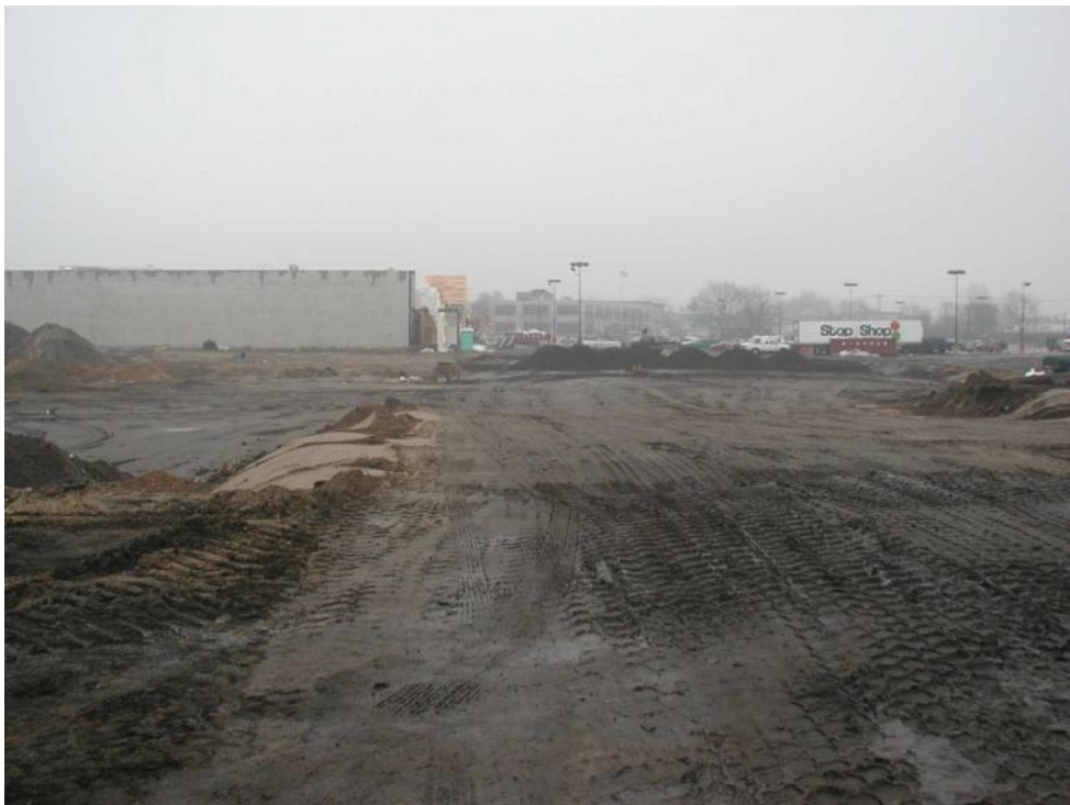
Photo 18. View east from west edge of excavation with backfilling nearly complete.
