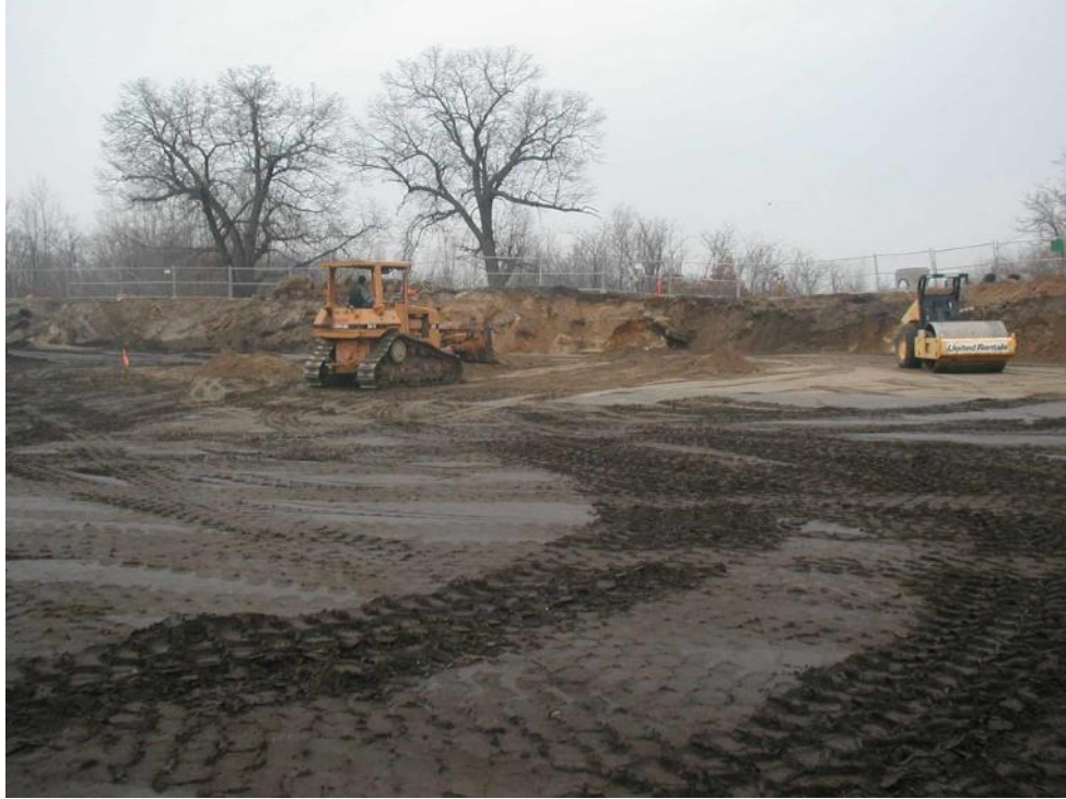
Photo 15. View northwest during backfilling.
