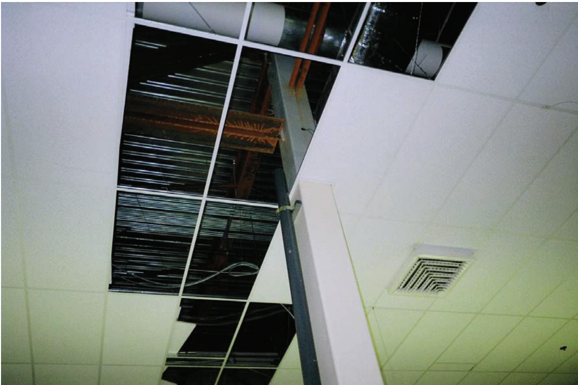
Drop Ceiling Penetration
