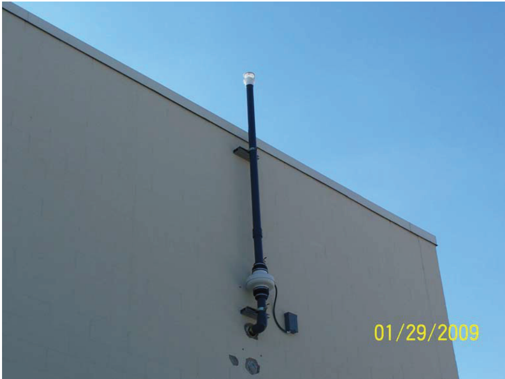
EW-7 Blower and Exhaust
