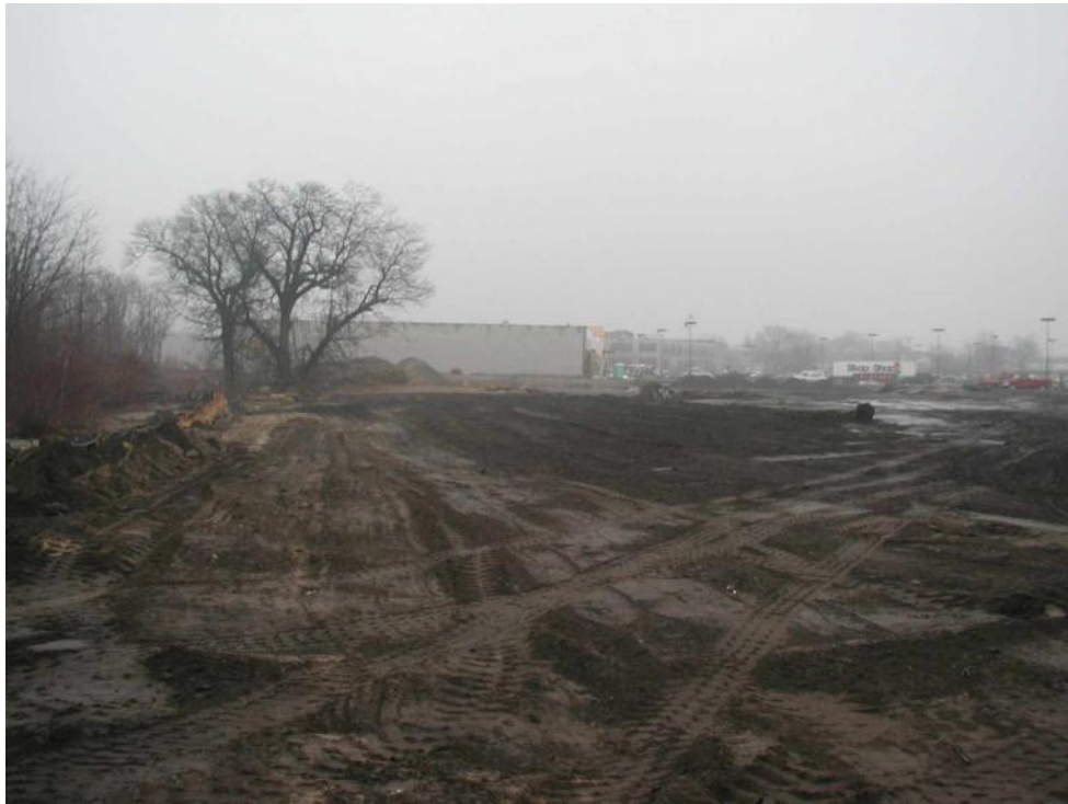
Photo 19. View east after backfilling and site cleanup.
