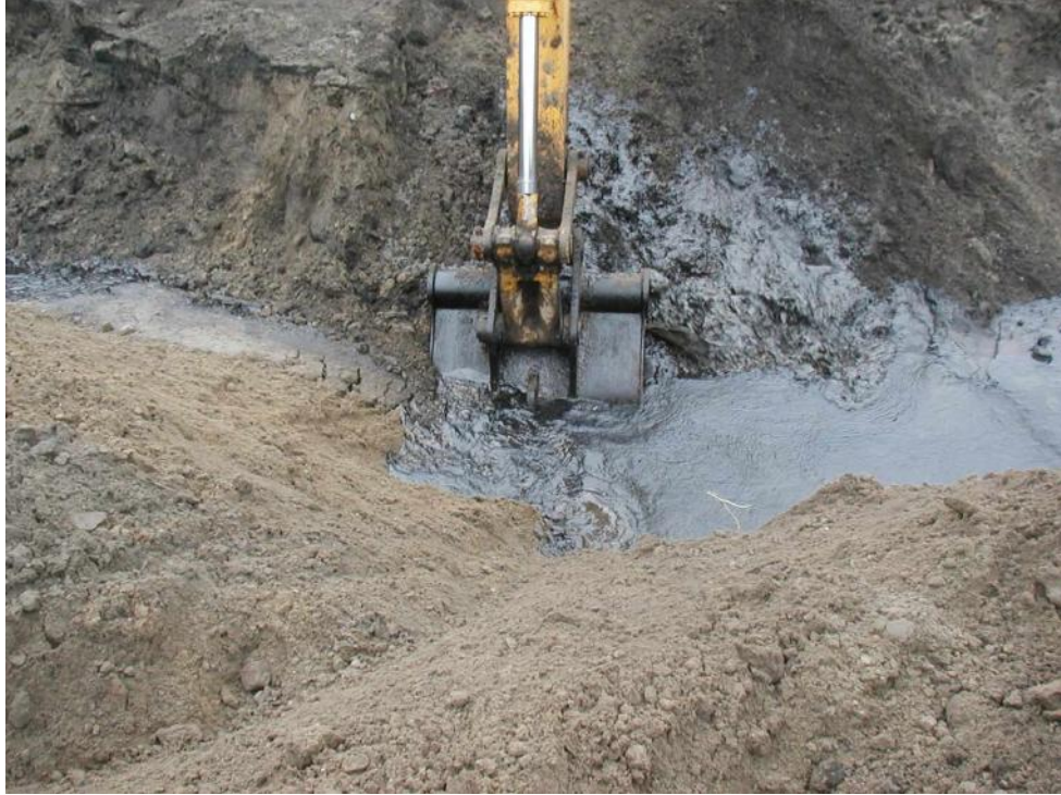
Photo 3. NAPL soil removal below water table.
