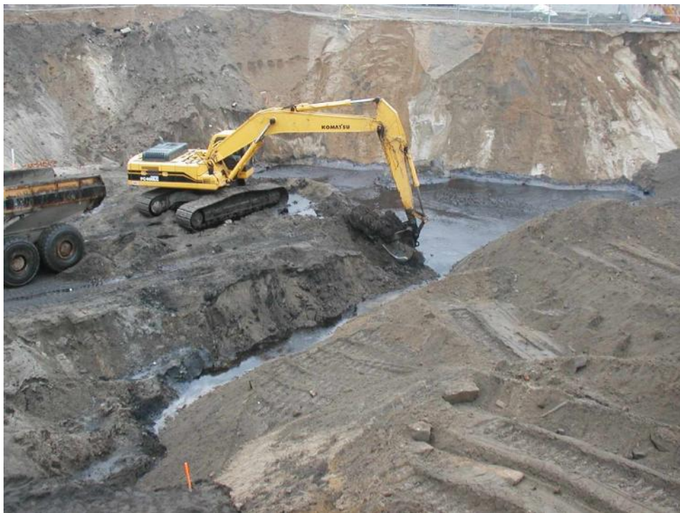
Photo 2. Removing NAPL soils.
