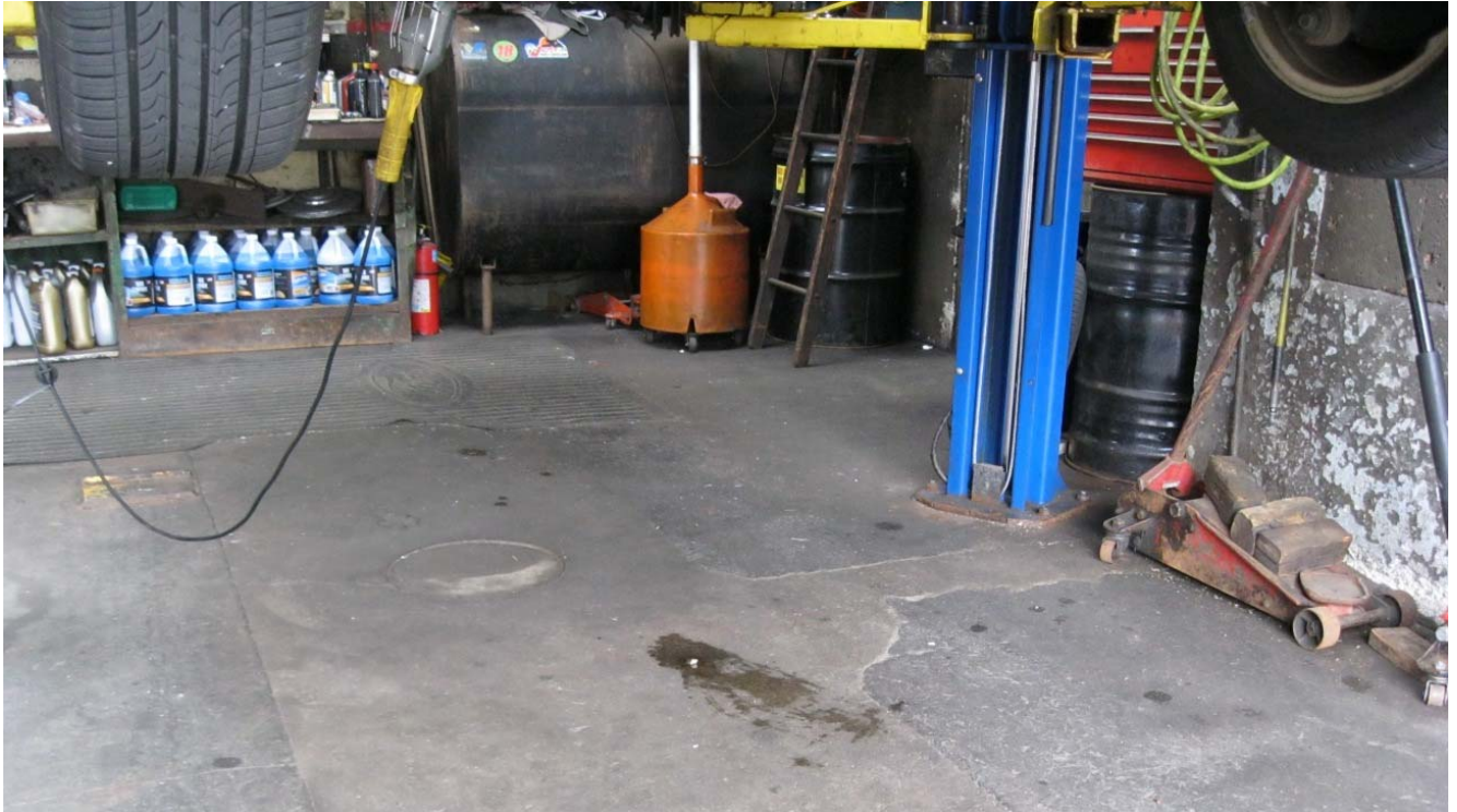
PHOTO 14: Looking north-northeast into the eastern service bay, showing heating oil AST.
