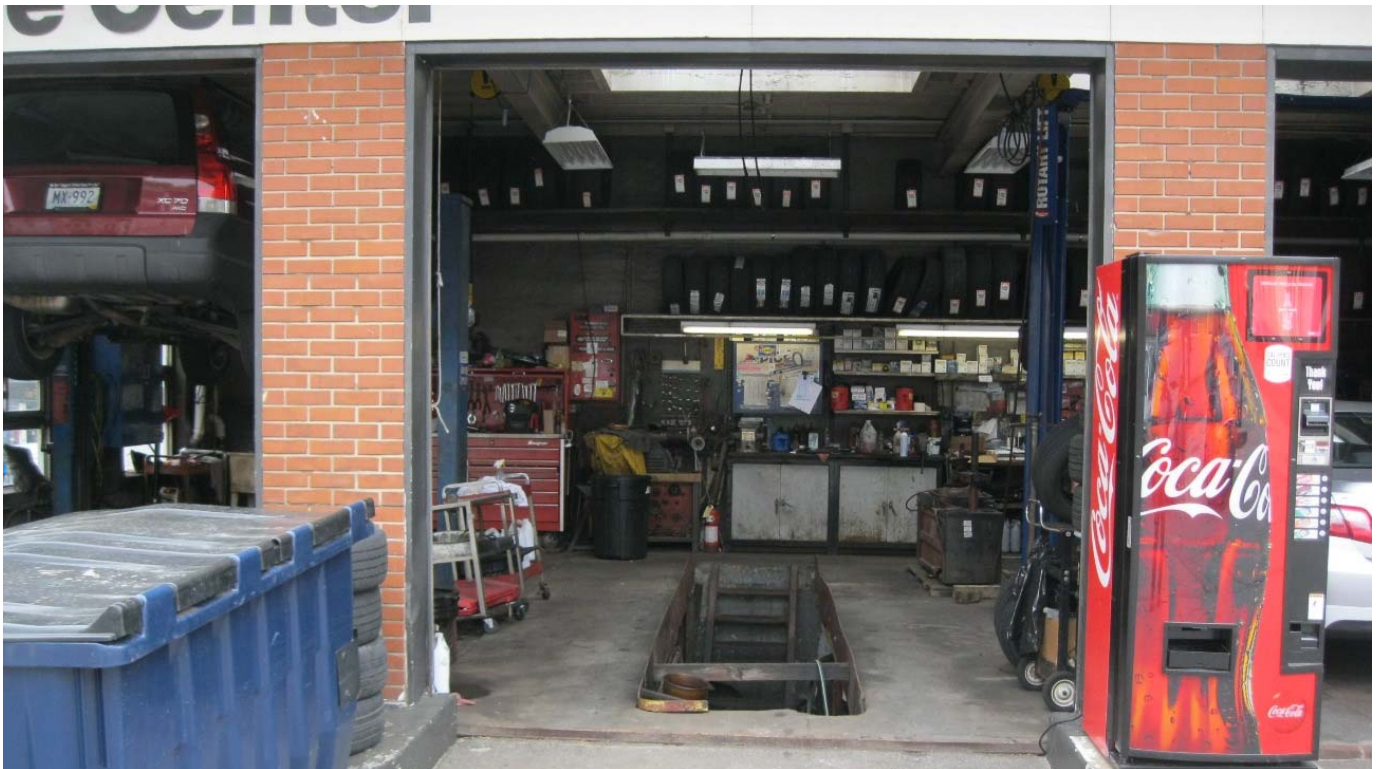
PHOTO 11 : Looking north into the center service bay, showing mechanic's pit opening.
