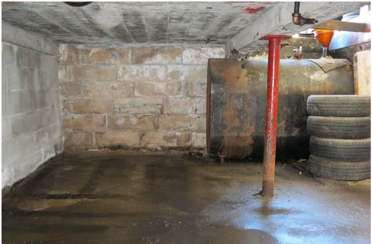
PHOTO 13 : Looking south, as above, showing waste oil UST.
