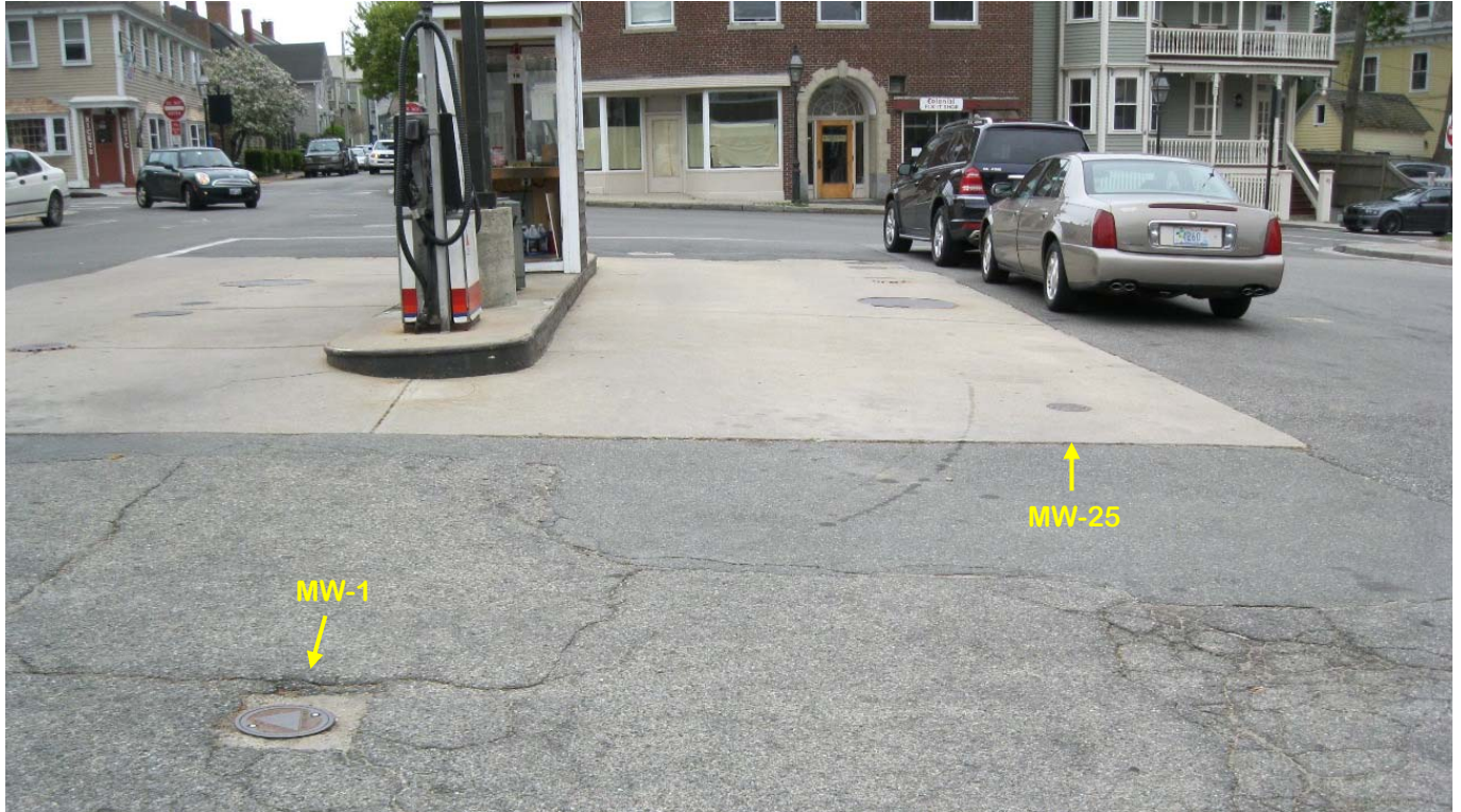
PHOTO 5: Looking south-southwest from the subject property, showing the pump island, tank pad, and residential and commercial properties across Touro Street. Monitor wells MW-1 and MW-25 are visible.
