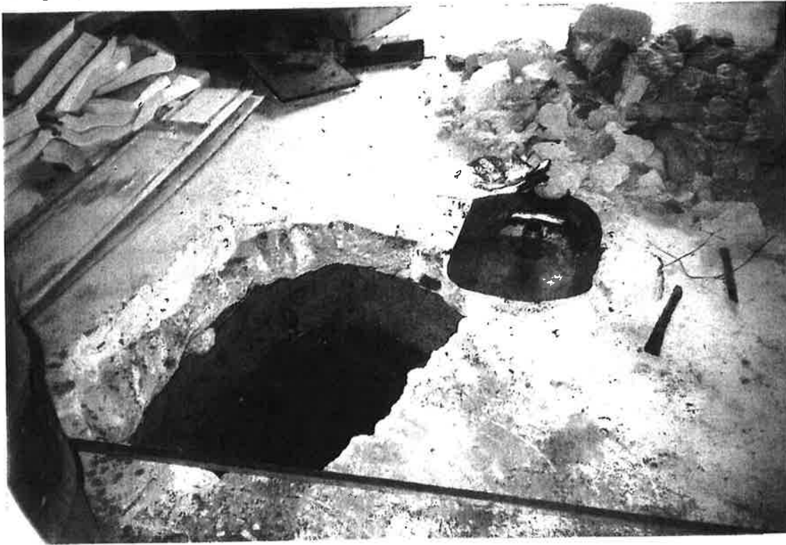
P-1 UST area prior to cleaning and filling.
