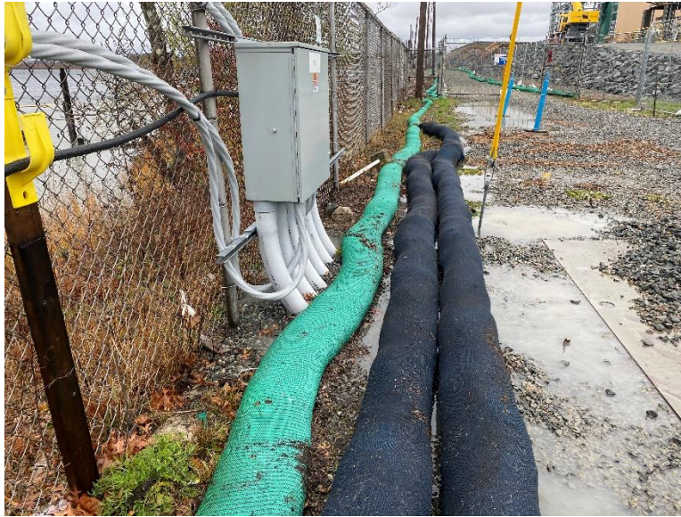
Photo 3: Additional filtrexx soxx installed in response to the unanticipated bypass.
