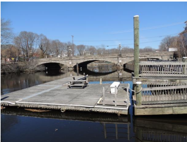
View downriver towards Valley Falls Dam from boat ramp
