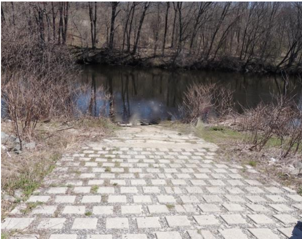
Boat Ramp at Rivers Edge Rec Complex (site of DV-02)
