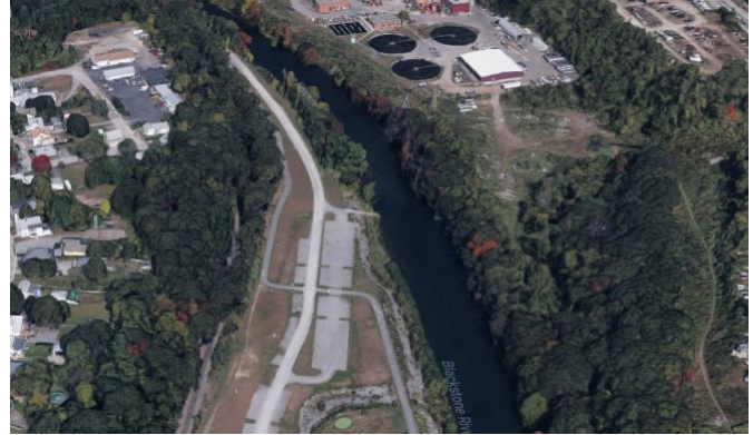
Site of DV-02 at Rivers Edge Recreation Complex looking upriver
