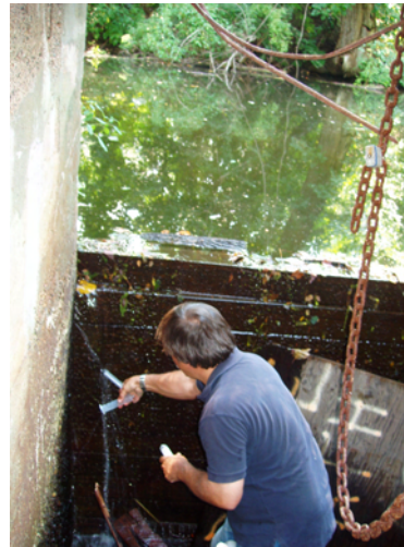
Figure 8-5: Blackstone Canal, southern weir, looking toward the canal (8/10/04).
