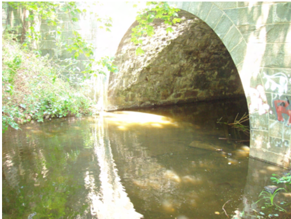
Figure 8-9: Blackstone Canal, sill at Front Street bridge (7/12/05).
