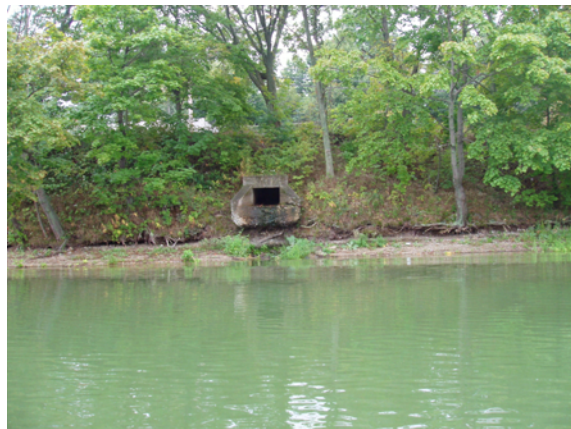
Figure 8-12: Scott Pond South, outfall OF-407 on southern shore (9/16/04).
