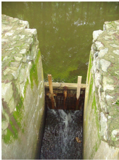
Figure 8-3: Blackstone Canal, northern weir, looking toward the canal (7/14/04).
