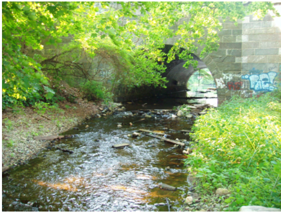
Figure 8-8: Blackstone Canal, sill at Front Street bridge (8/10/04)
