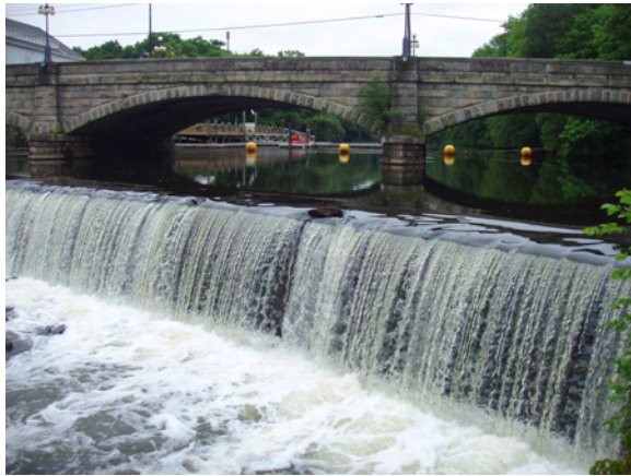
Figure 7-2: Valley Falls Dam, controlling the elevation in Valley Falls Pond (7/14/04).
